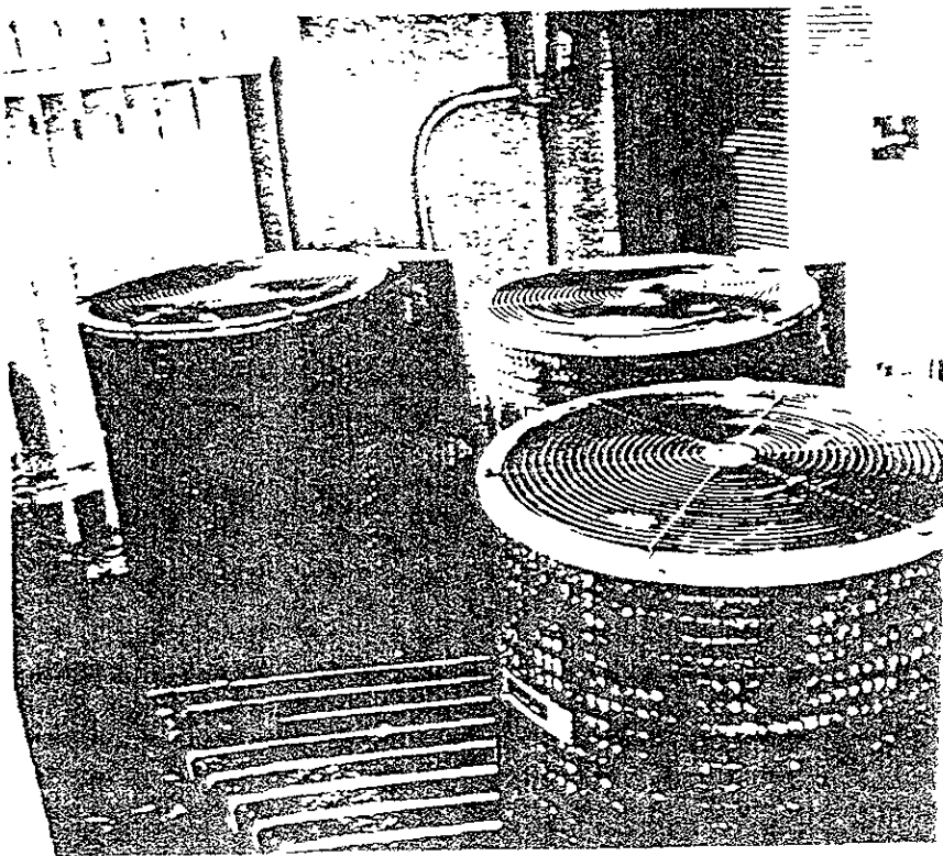
Air conditioning unit, south side of building
