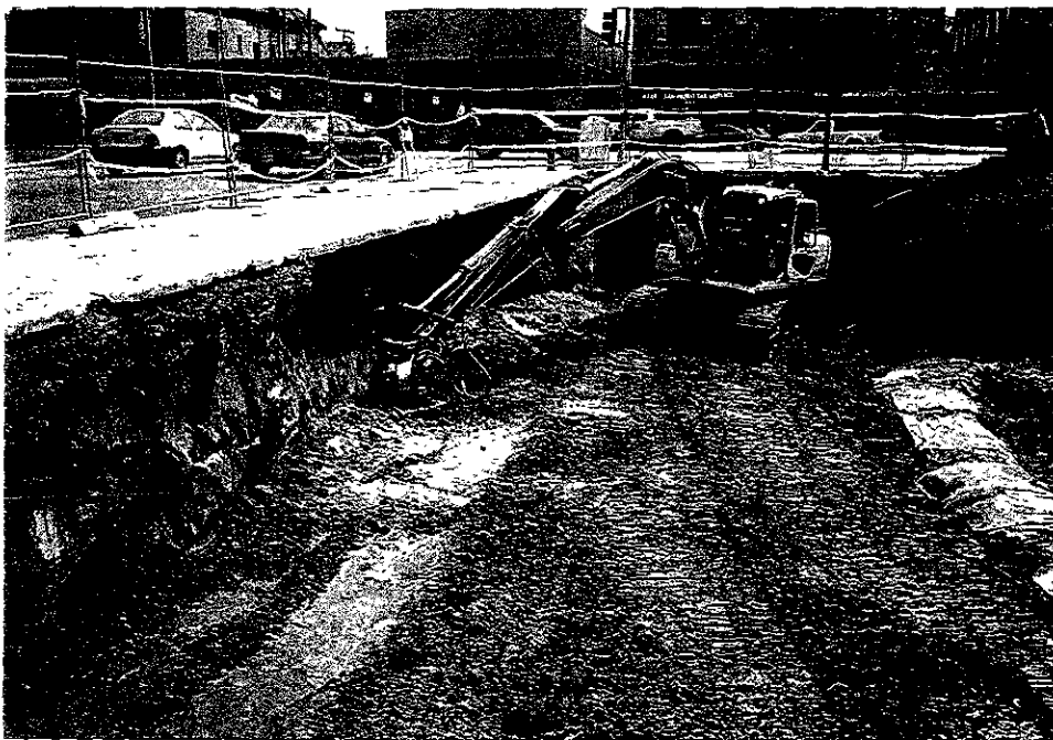
Soil Backfill Being Compacted Along Edges of Excavation with Vibrating Plate Compactor Photo R6-F27 - View: East
