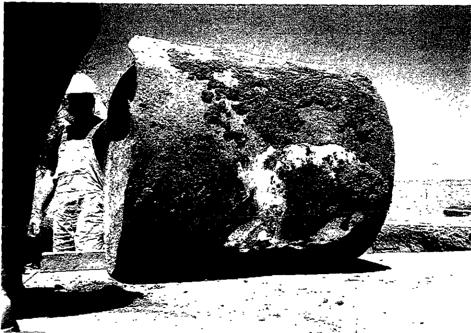
UST # 3: Bottom in Fair Condition Photo R5-F12
