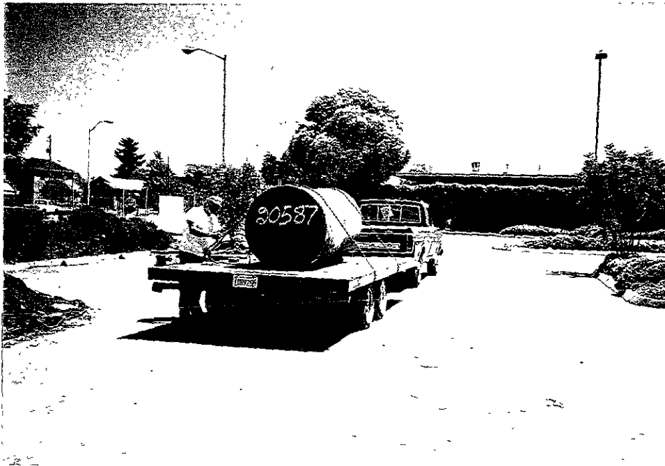
UST # 2 Loaded For Transportation From the Site Photo R2-F5
