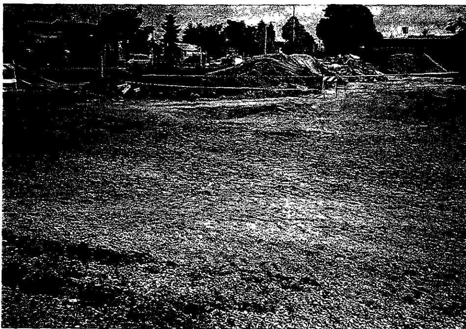
Excavation Backfilled to Near Ground Surface Pending Site Restoration Photo R7-F7 - View: Southeast
