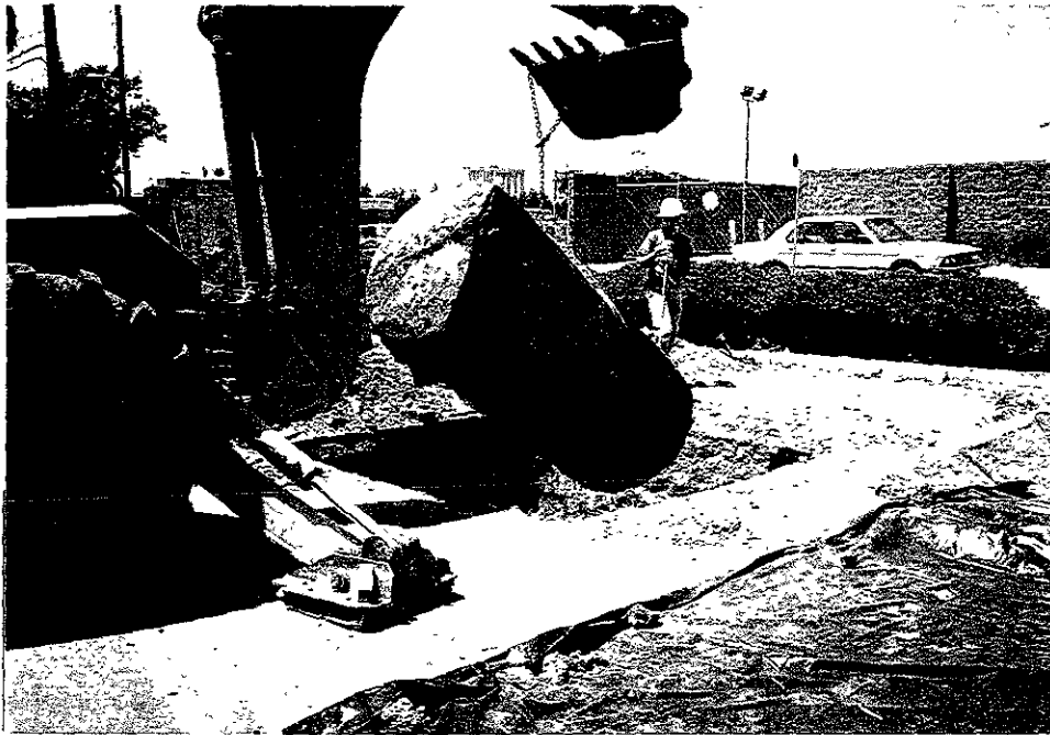
UST # 1 Being Removed From the Excavation Photo R1-F4 - View: Northwest
