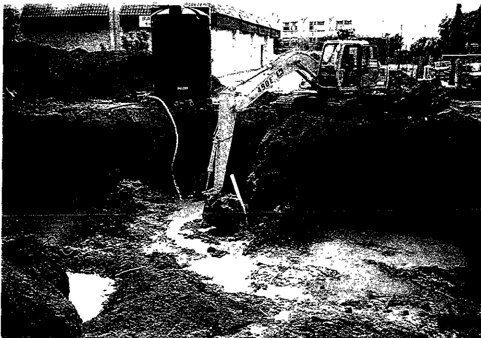
Detruction of Groundwater Monitoring Well MW-1 Photo R4-F7 - View: West
