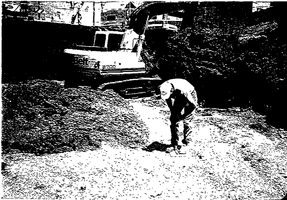
Compaction Testing Being Conducted by Miller Pacific Engineering Group, Inc. Photo R6-F22 - View: Northeast
