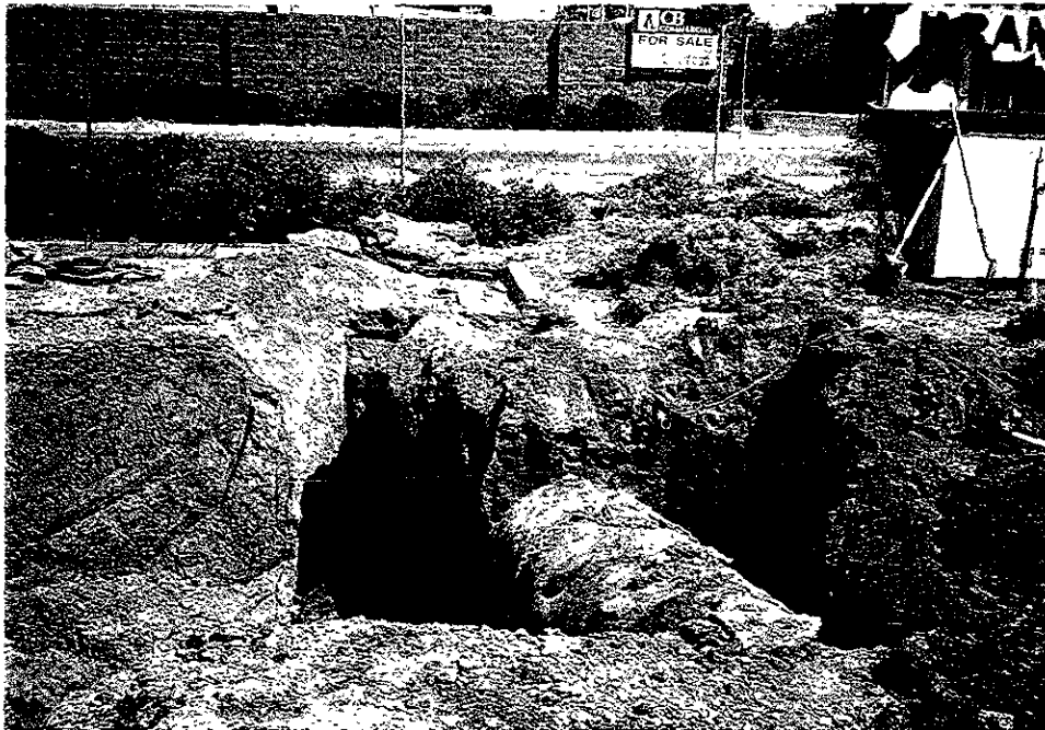
UST # 2: In Place Just Before Removal Photo R1-F21 - View: North
