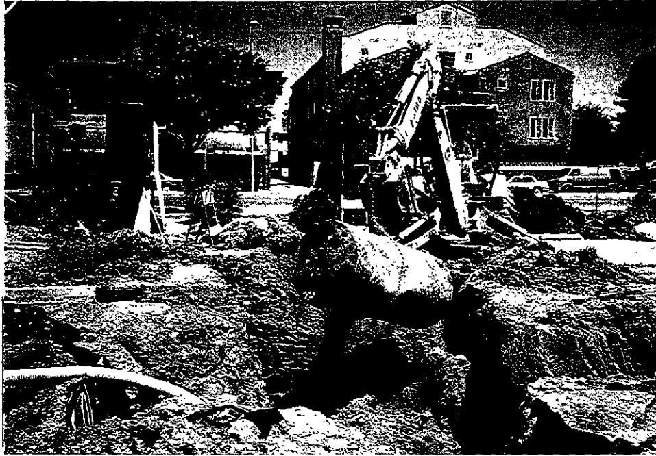
UST # 2 Being Removed from the Excavation: Soils Below UST Not Obviously Impacted Photo R1-F25 - View: East
