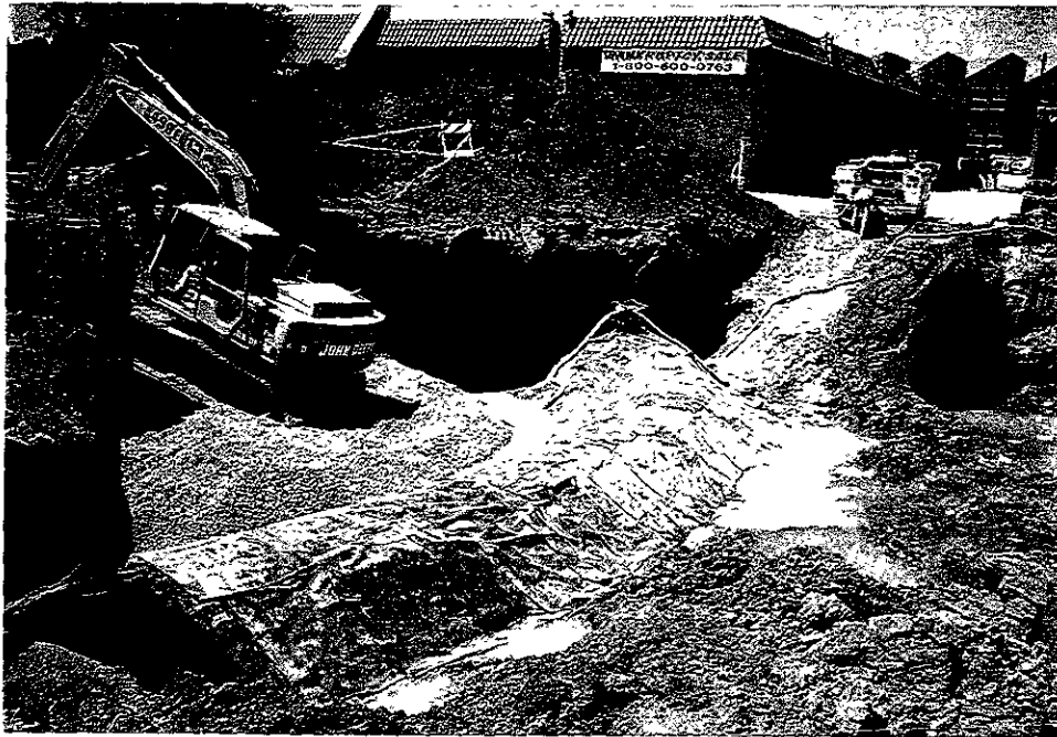
Polyethylene Liner with Bentonite Back Placed Over Berm and Concrete Layer Photo R6-F13 - View: Southwest
