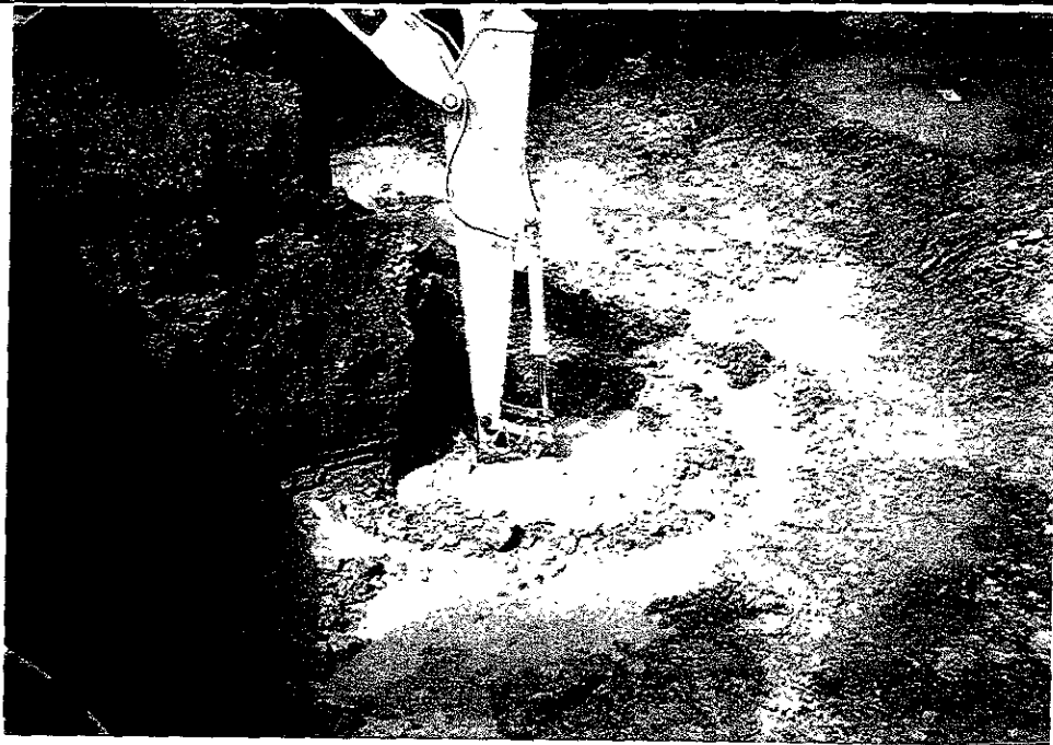
Over-excavation of Monitoring Well Filter Pack Photo R4-F14 - View: North
