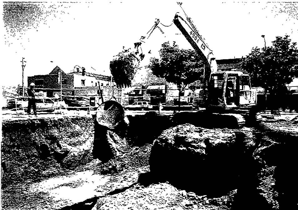
UST # 4 Being Removed From the Excavation: Soils Below UST Not Obviously Impacted Photo R5-F15 - View: Northeast
