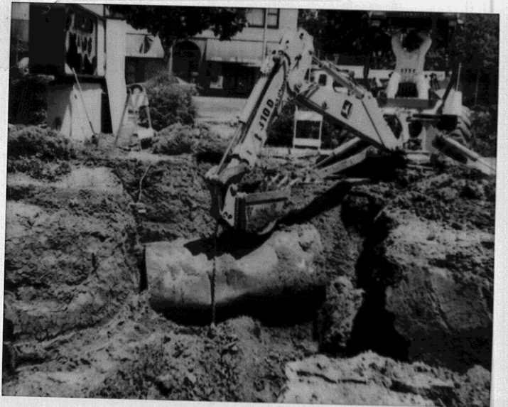
Work #2 - facing San Pablo St. 7/21/97
