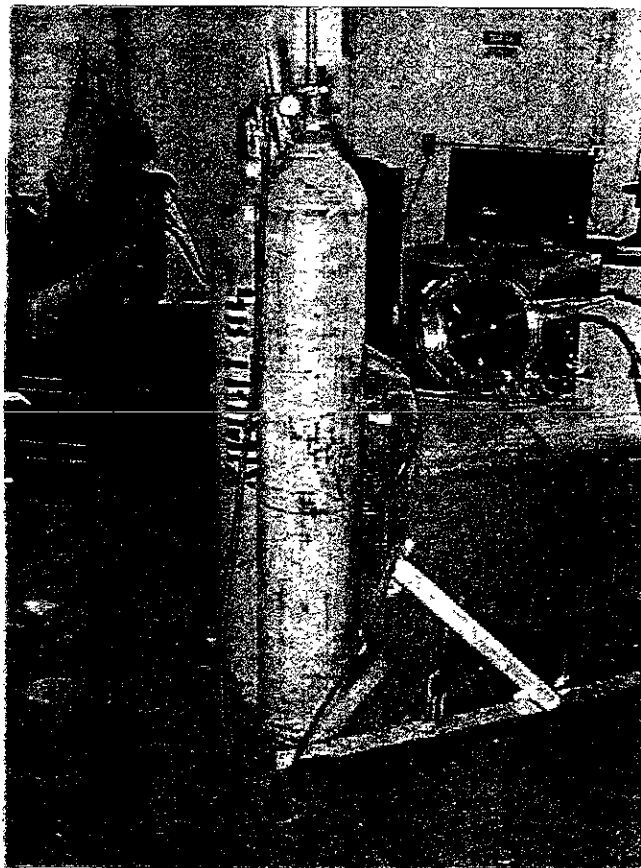
Photograph #8 Argon/helium and carbon dioxide cylinders stored at Van Mulder Sheet Metal.
