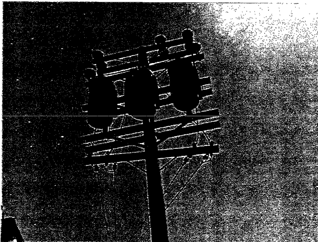
Photograph #10. Pole-mounted transformers.
