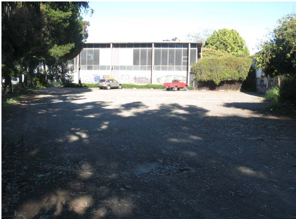
Photo 6: Looking east from the central site parking area at the rear of the office building.
