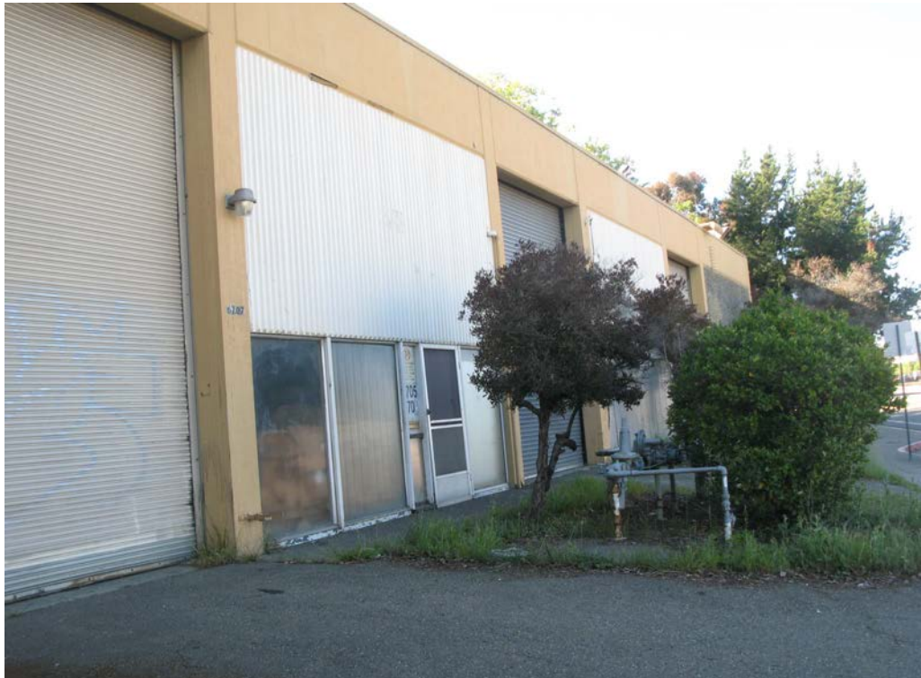
Photo 5: Looking northwest at the eastern wall of the warehouse building.
