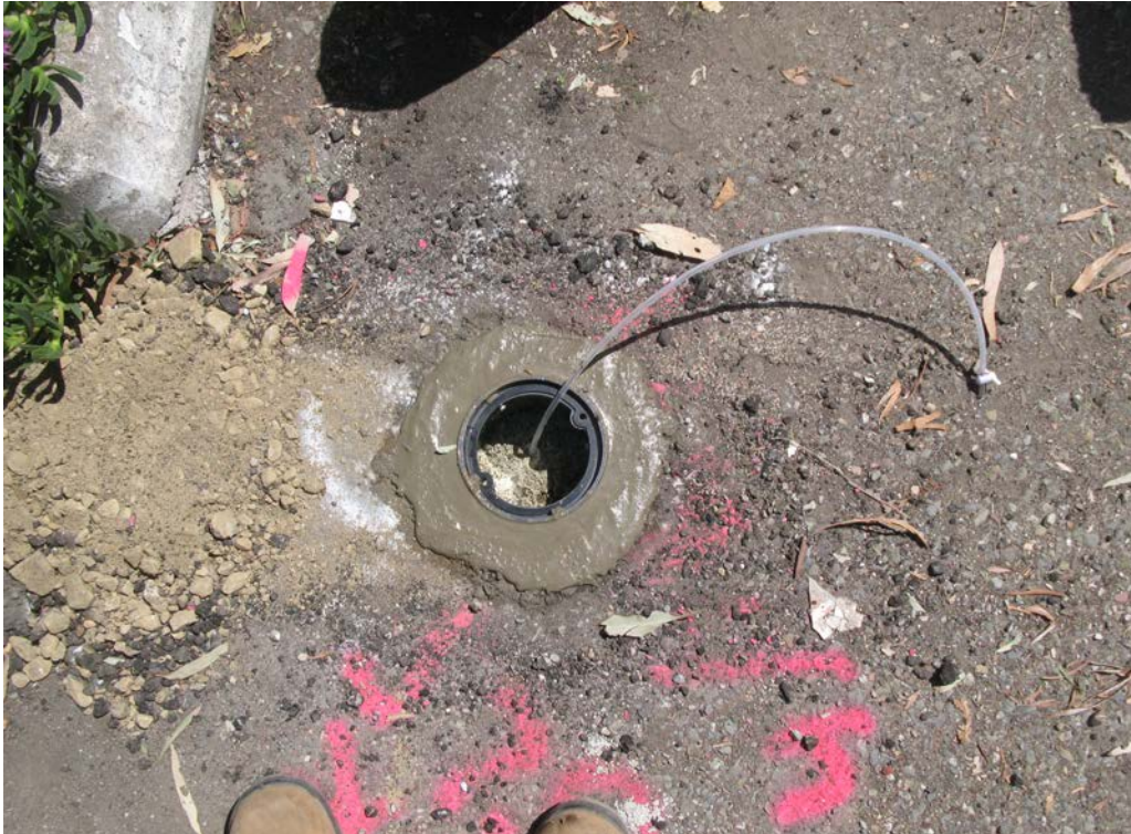
Photo 21: Semi-permanent soil vapor well at location SG-1 after installation.
