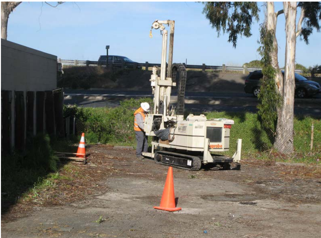
Photo 18: Looking west at drill rig positioned at location SG-5.
