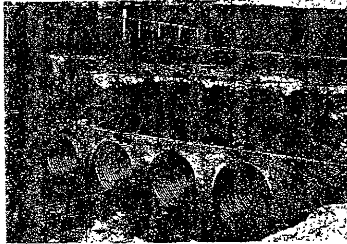
The structural capacity of Terra-Fill was utilized in this culvert fill to overcome heavy traffic loading on a roadway with minimal top cover over the culvert. — La Cygne, Kansas
