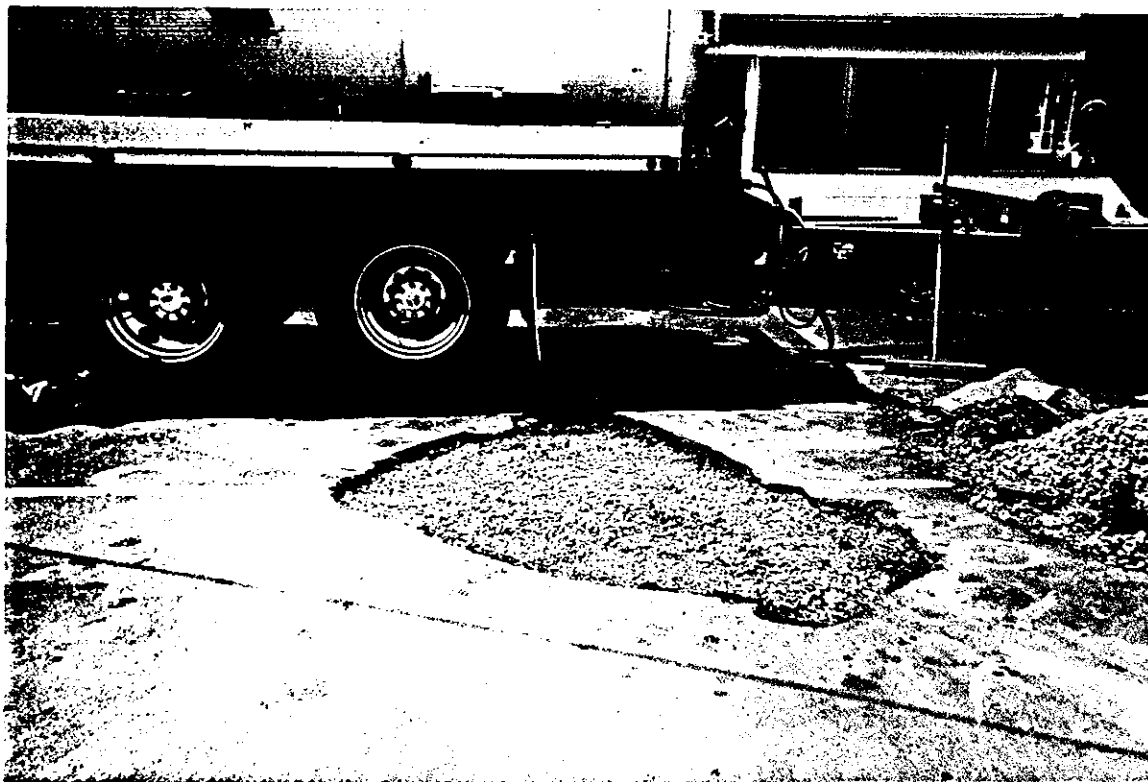
PHOTO 8. Excavation after crushed gravel has been compacted.
