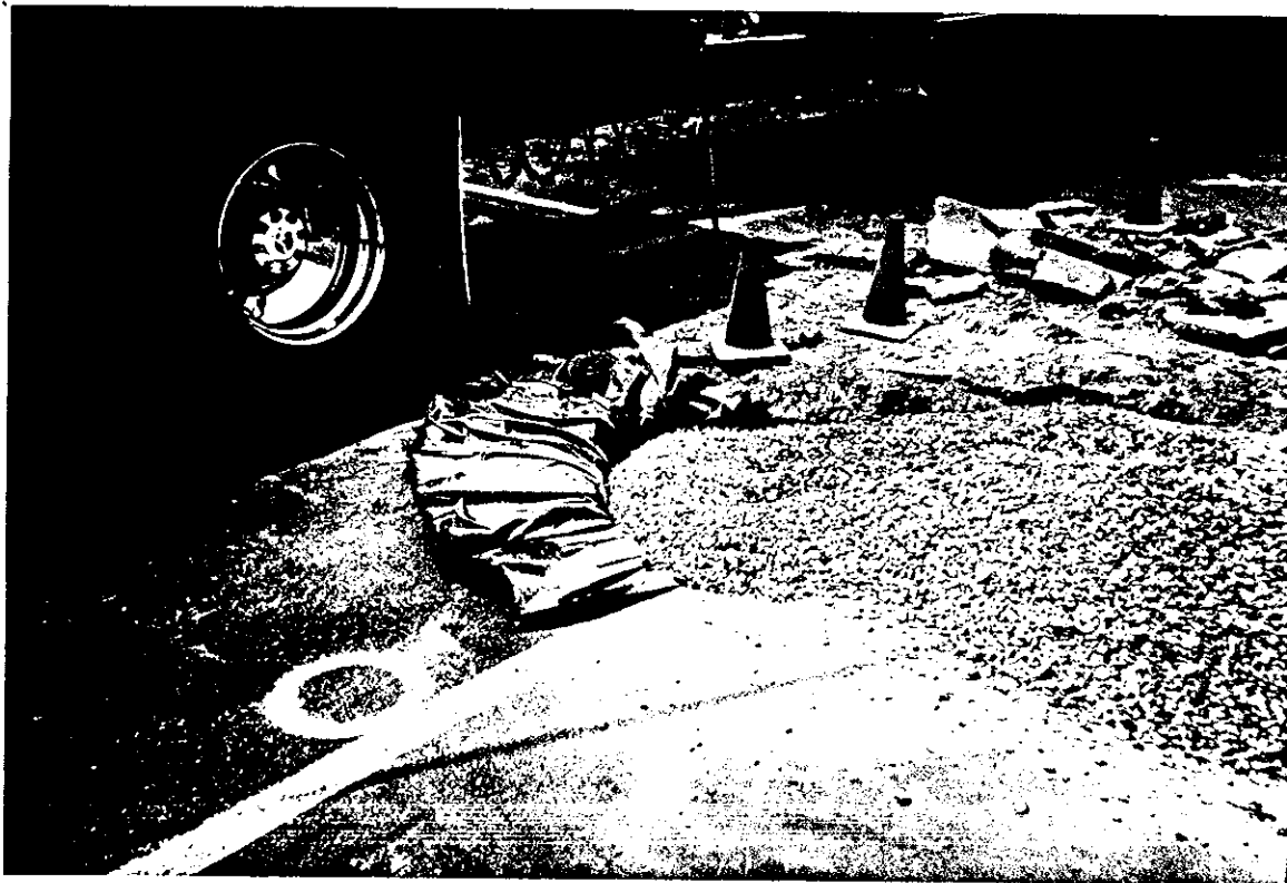
PHOTO 7. Partial view of backfilled excavation. Plastic sheet separates fill from 3/4" diameter crushed gravel.
