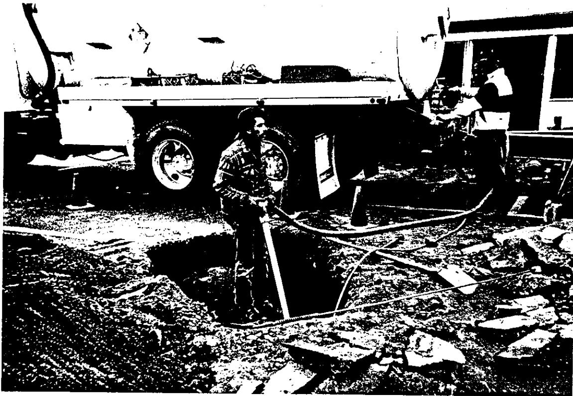
PHOTO 3. Pumping waste oil out of UST.
