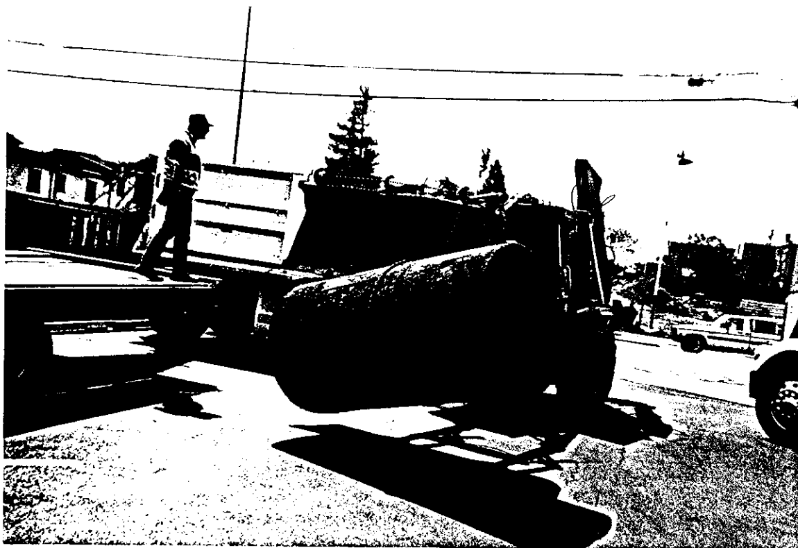
PHOTO 4. Hauling off UST.
