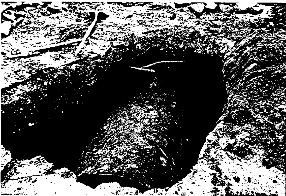
PHOTO 2. View of the 550 gallon UST and underground pipes. Pipe running across excavation is not associated with the tank.
