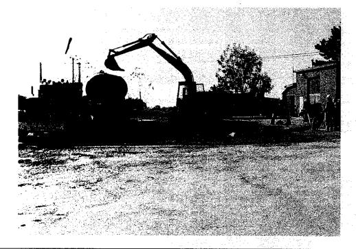
Subject: Removing tanks and loading onto truck to haul off for destruction.
