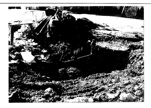
Subject: First evidence of contamination encountered while exposing the diesel piping to the UFST: product seem along piping
