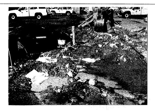
Subject: View of backhoe breaking up and scraping away concrete cover before starting to excavate
