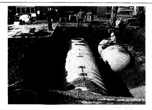
Subject: View of new 12,000 gallon gasoline and 2,500 gallon diesel tanks being installed in excavation, looking north
