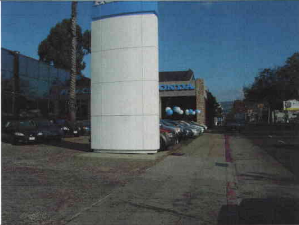
East side of Property (along Broadway) from the south
