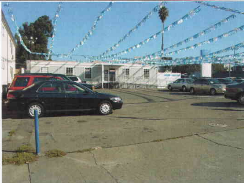
South side of Property (former gasoline station) from the southwest
