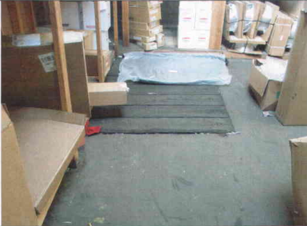
Wood hatch over pit in 3741
