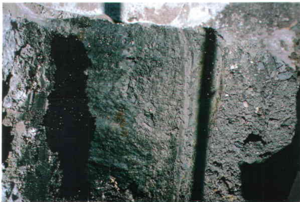
PHOTOGRAPH 8. SECONDARY EXCAVATION (14 FEET BELOW GRADE)
