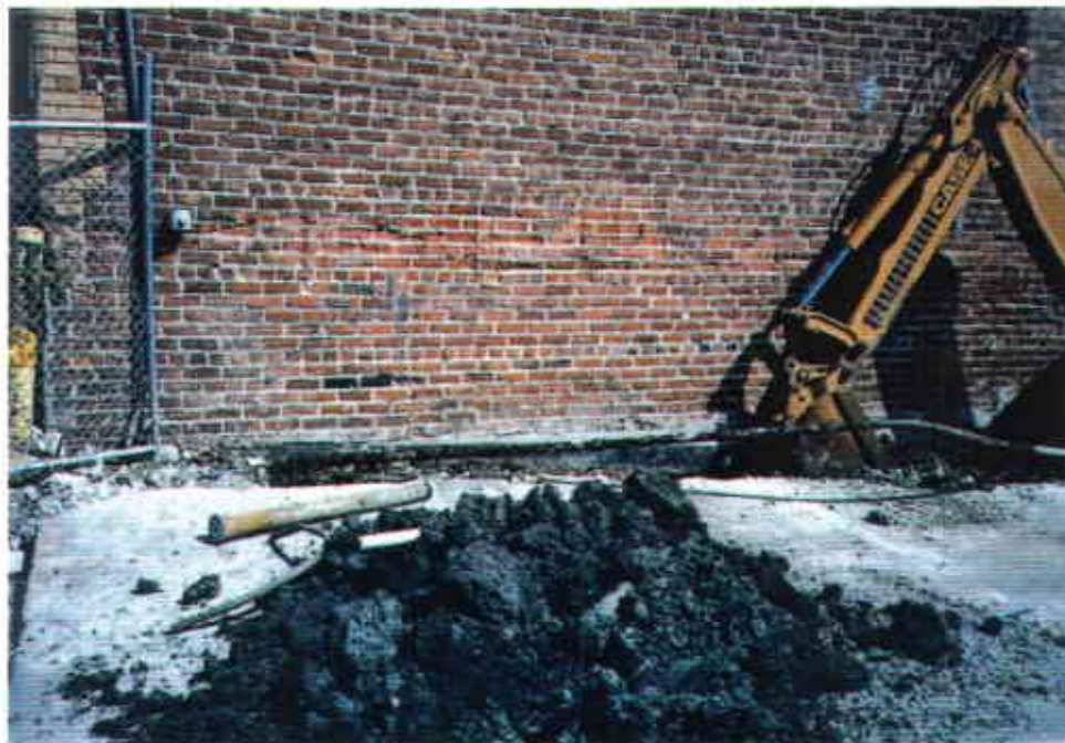
PHOTOGRAPH 4. EXCAVATION OF THE PRODUCT LINE
