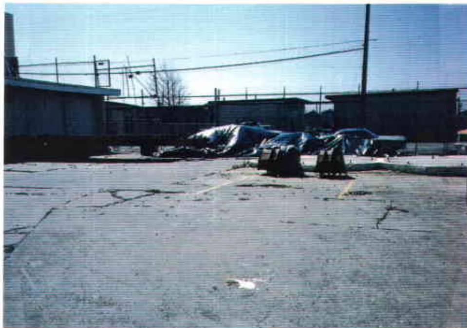
PHOTOGRAPH 6. EXCAVATED SOILS COVERED WITH VISQUEEN
