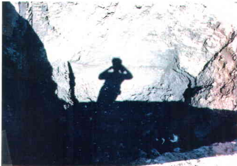
PHOTOGRAPH 5. BOTTOM OF TANK PIT AFTER TANK WAS REMOVED
