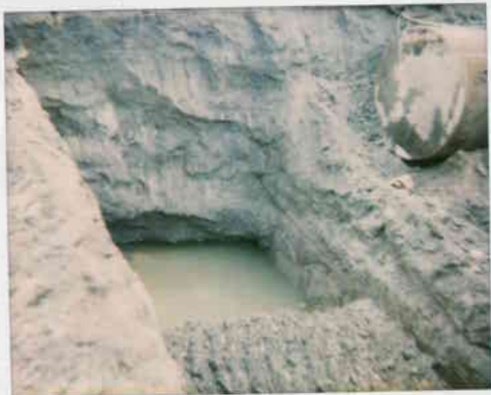
- 11/10/94 - overexcavated leach pit S. end Unocal 7850 Am. Valley Rd
