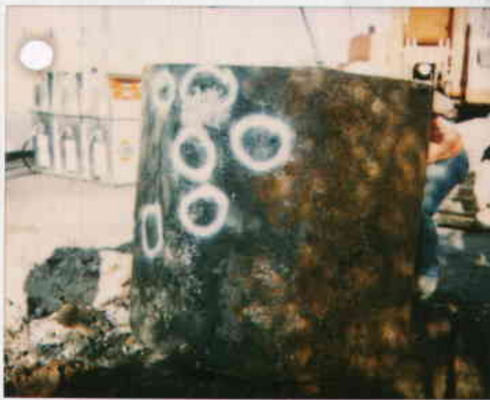
11/9/94 7850 Amador Valley 280 waste oil tank - circled holes
