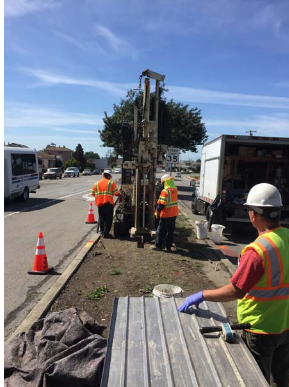
Plate 7. Cascade Drilling Converting MW-10 to MW-10R
