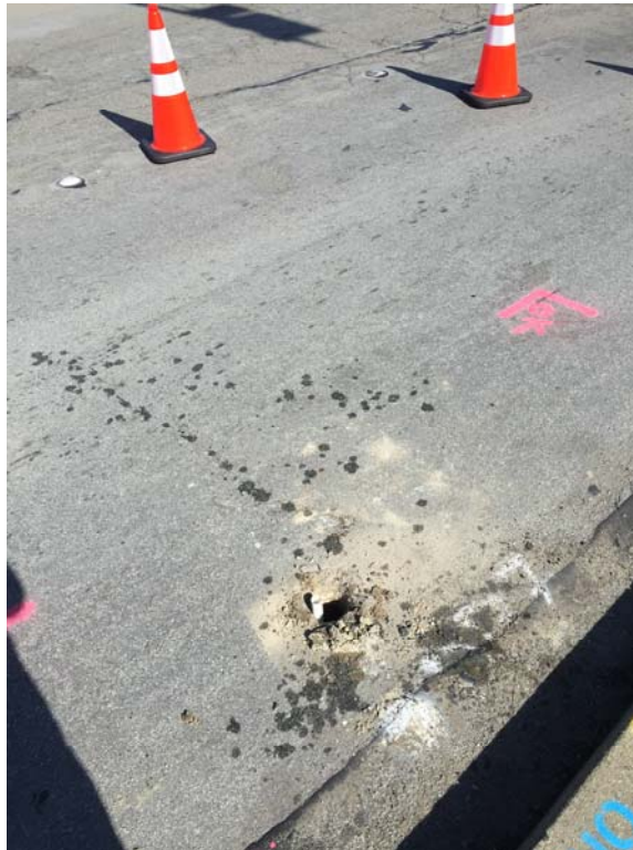
Plate 1. Completion of DP-9
