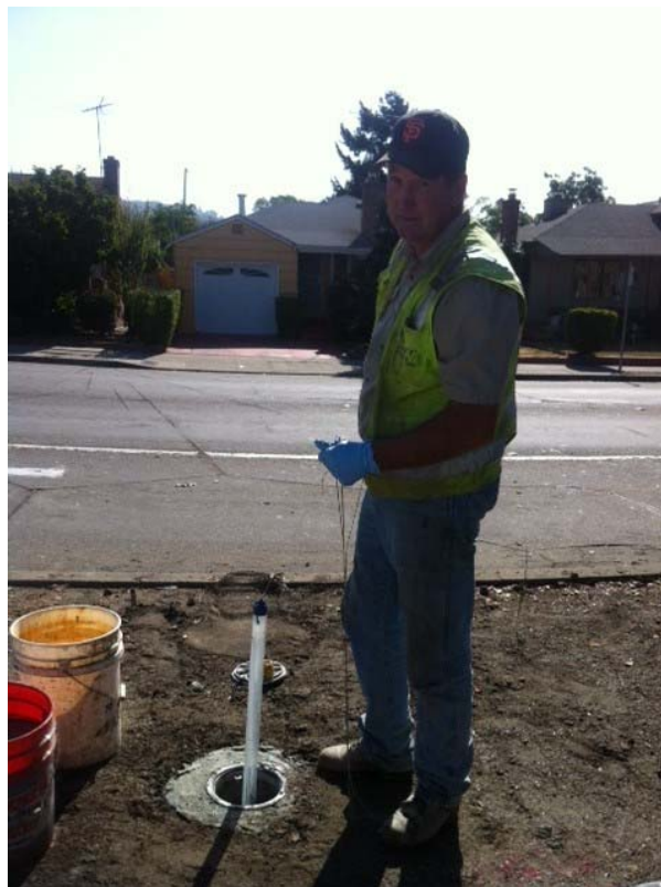
Plate 4. Fisch drilling developing MW-10
