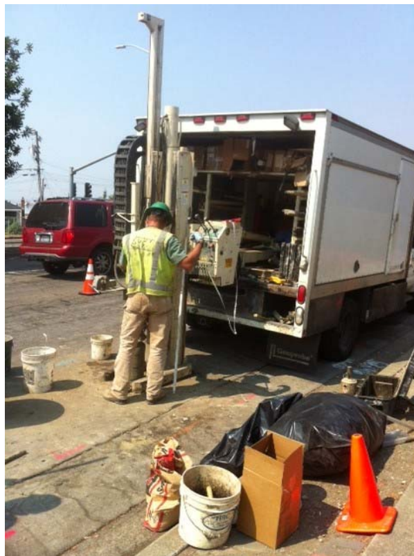
Plate 2. Fisch Drilling set up on MW-11
