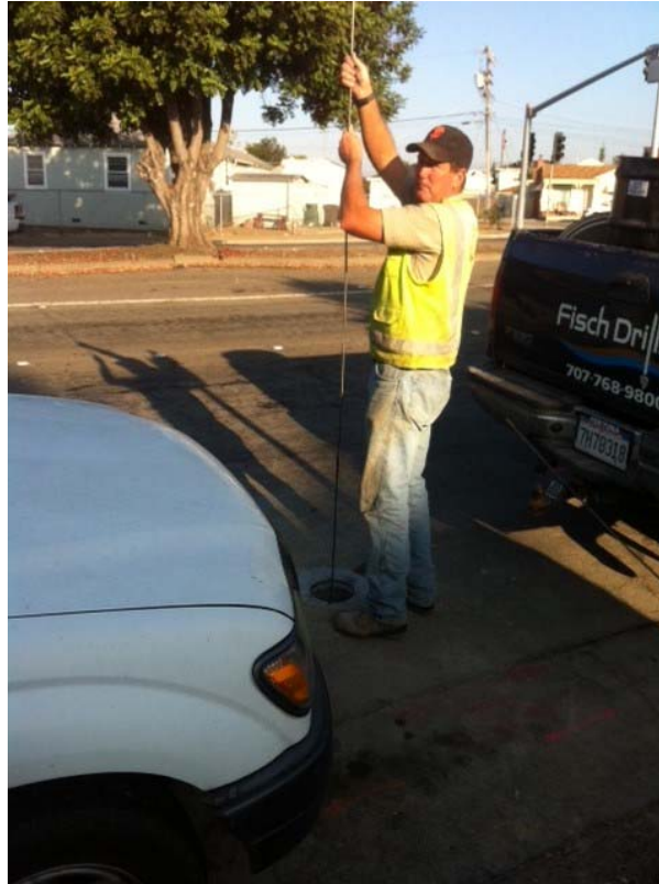
Plate 3. Fisch Drilling developing MW-11
