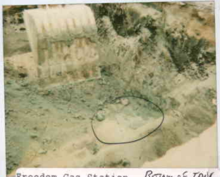
Freedom Gas Station 15101 Freedom Ave. San Leandro 5/20/99 RW Tank removal activities
