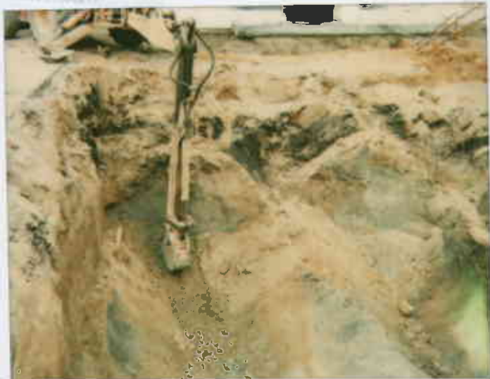
Freedom Gas Station 15101 Freedom Ave. San Leandro 5/20/99 RW Tank removal activities
