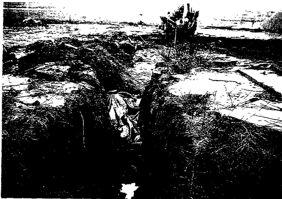
Westside view of Over-Excavation Activities at Building 888 February 11, 1998
