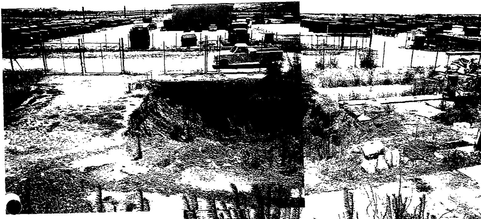
Northside view of the former UST at Building 888 June 1997
