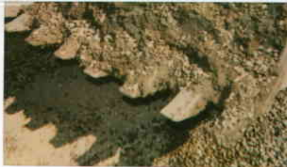
Soil beneath w/o UST 9/29/96 appeared to have no odors or staining
