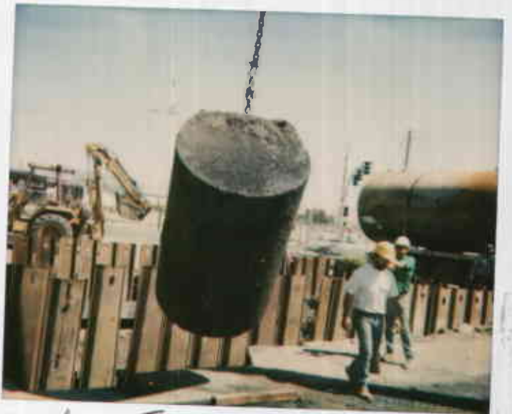
Waste oil Tank 6401 Dublin, Failed waste oil Tank Unocal
