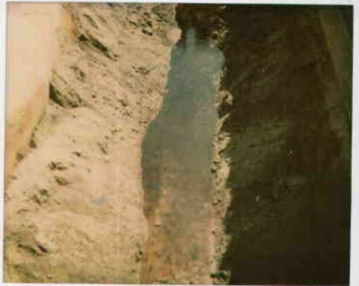
Unocal Station Tank Removal 6401 Dublin Dublin. oil/H 2 O/GAS
