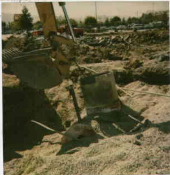
waste oil UST in progress 9/27/96 6401 Dublin Blvd Dublin
