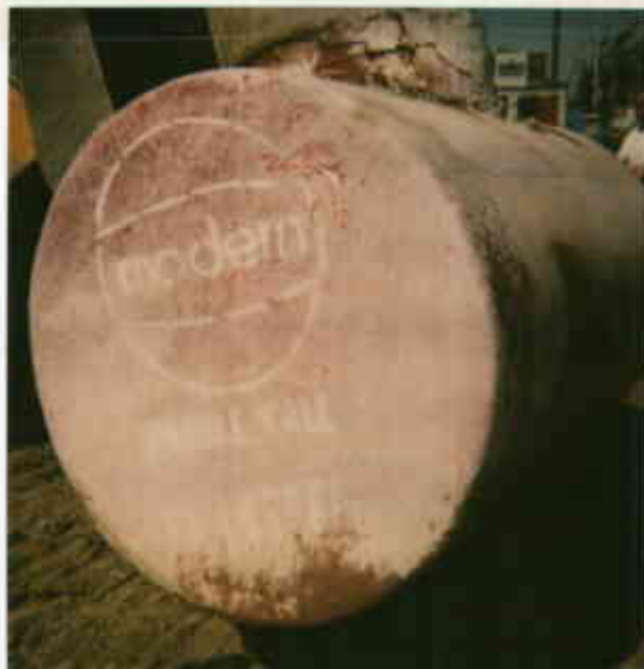
waste oil UST 9/27/96 fiberglass double walled in good condition 6401 Dublin Blvd Dublin
