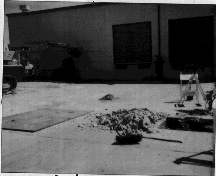
7-30-93 Aratex - 330 Chestnut St. Oakland CA GE fueling pit removals
