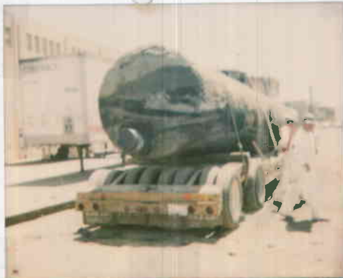
8/13/94 1450 Sherwin Ave 7P-4 USTs removed 83317211124-2
