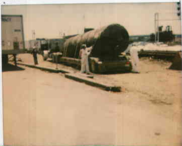
8/3/94 Sherwin Ave - SP underground 83317211124-2 Tank removed.
