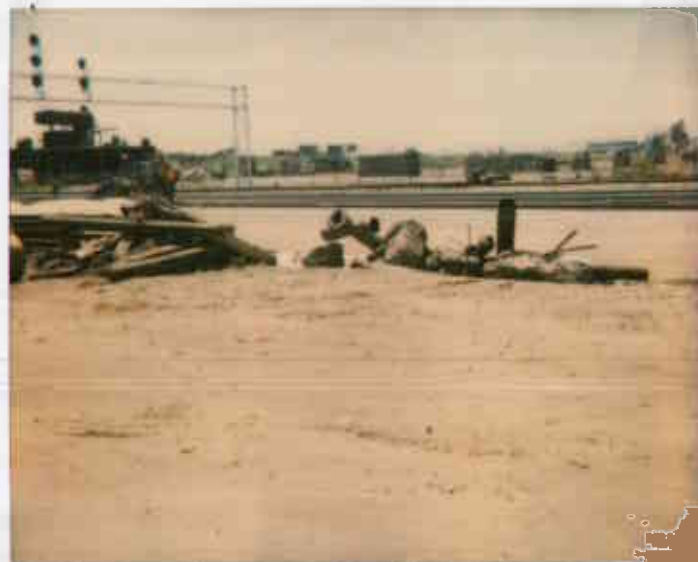
8/3/94 1450 Sherwin Ave - SP 03317211124-2 UST removal
