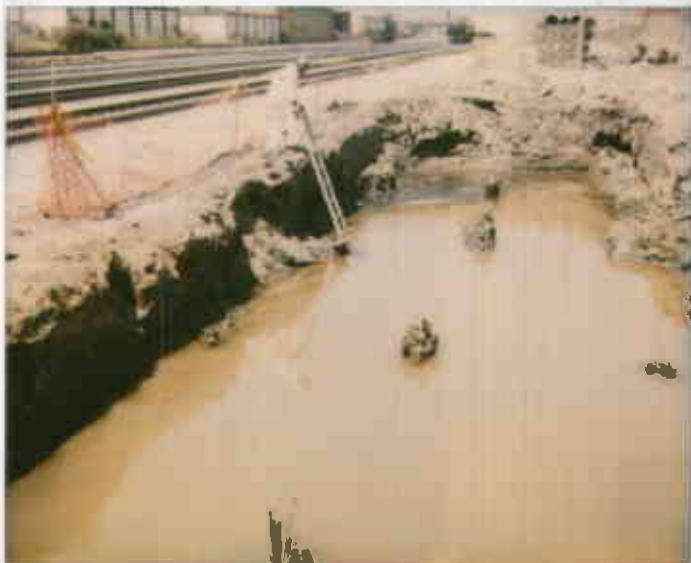
8/3/94 1450 Sherwin Ave 83317211124-2 4 USTs removed
