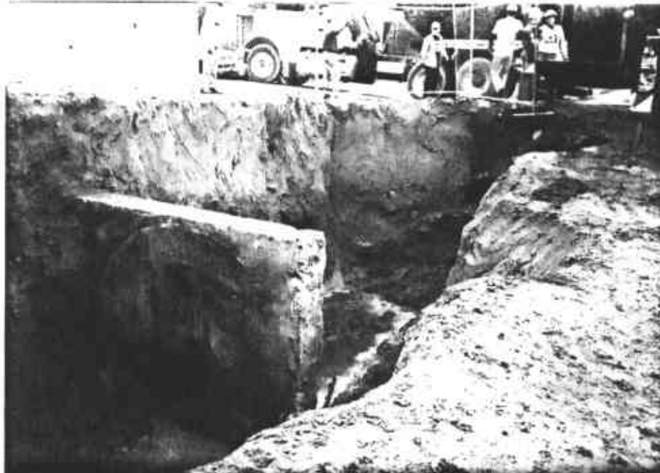
Views of soil contamination on the southwest and southeast sides of the excavation. There was approximately 6-inches of rain water at the bottom of the excavation.
