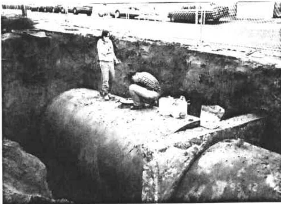
Adding dry ice to the fuel tanks prior to removal
