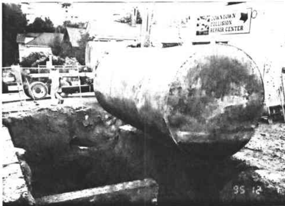
View of Tank No. 1 prior to being removed. Note the concrete separation wall between the two tanks. The separation wall was left in place.
