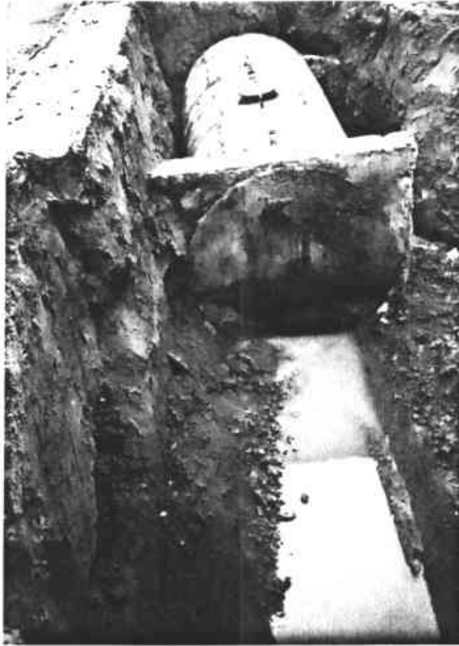
View of Tank No. 1 prior to being removed. Note the concrete separation wall between the two tanks. The separation wall was left in place.
