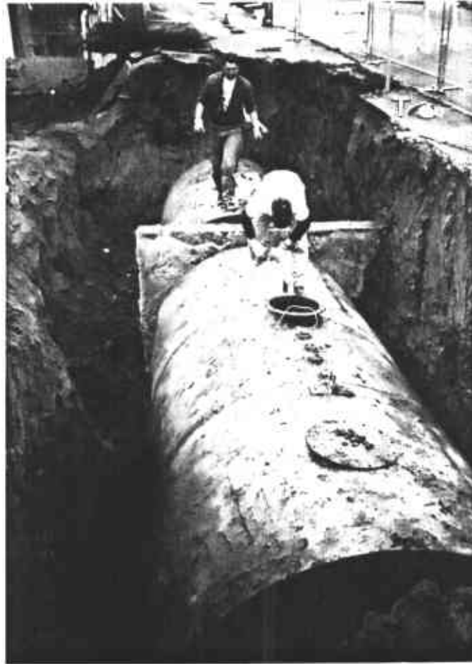
Adding dry ice to the fuel tanks prior to removal
