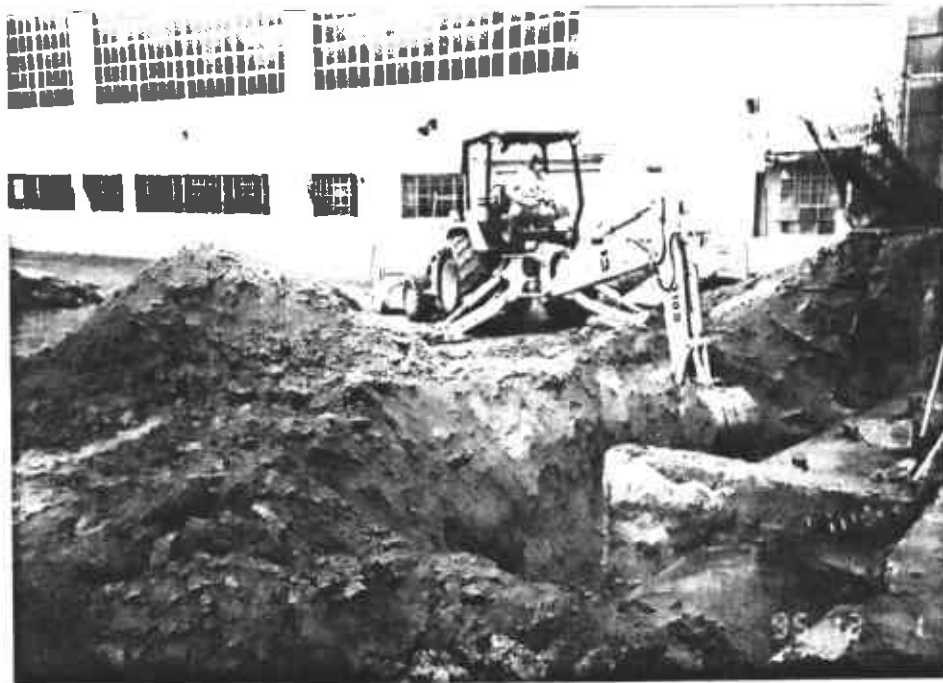
Uncovering top of fuel tanks under sidewalk adjacent to 30th Street.
