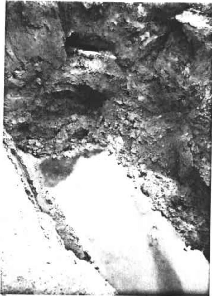
Views of soil contamination on the southwest and southeast sides of the excavation. There was approximately 6-inches of rain water at the bottom of the excavation.
