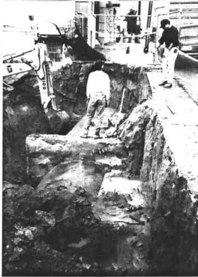
Uncovering top of fuel tanks under sidewalk adjacent to 30th Street.
