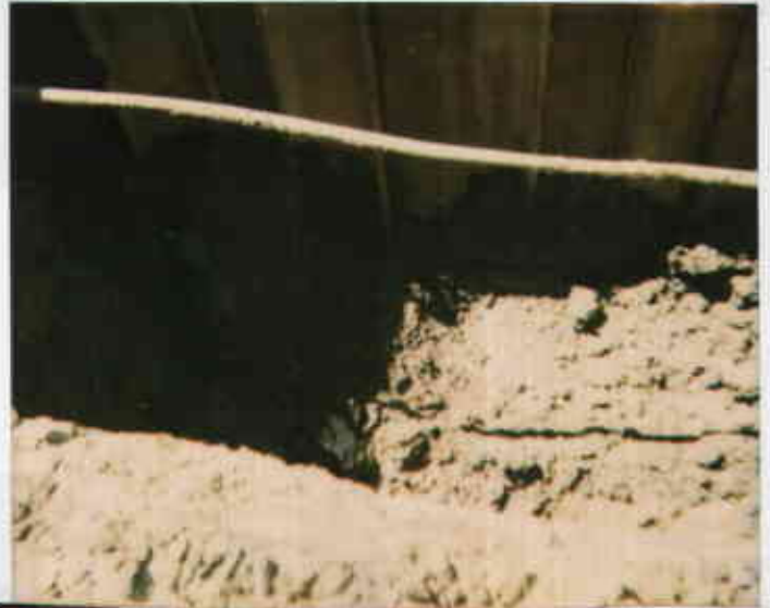
Former Firestone Tire 2984 Broadway - Oak 01717328093-2W 0026 5246 Tank pit established soil w/ storm COPIES & ENLARGEMENTS CALL 800-421-1030
