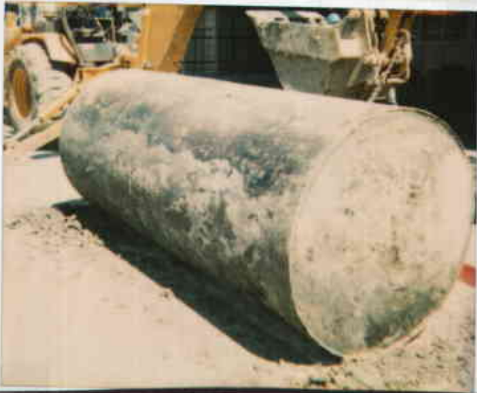
Former Firestone 2984 Broadway - Oak 01717328093-2W 0026 5245 ~1500g. Heating oil UST in good condition COPIES & ENLARGEMENTS CALL 800-421-1030
