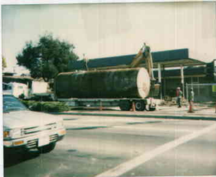
Basin # 604 1619 - 1st St. Livermore 10K-unleaded tank across 1st St. 03216211255-8 11/10/92
