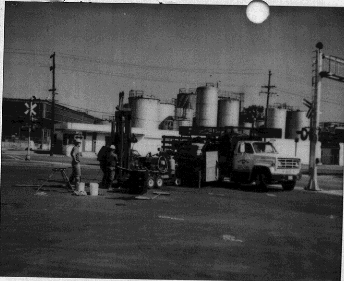
3925 Alameda Ave 3/7/94 Hydro-punches w/ Scotch Lube in background
