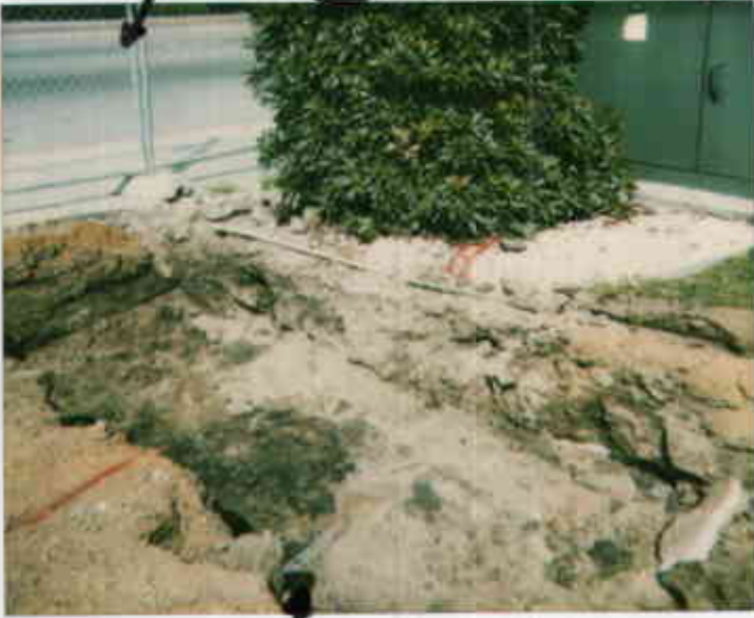
High voltage line
