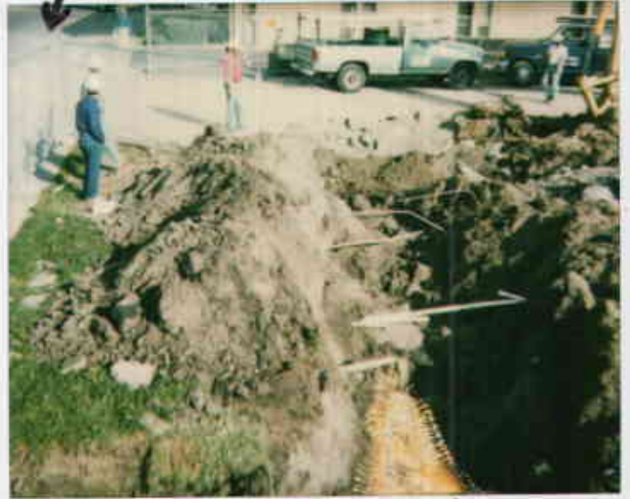
2nd/3rd generation piping trench
