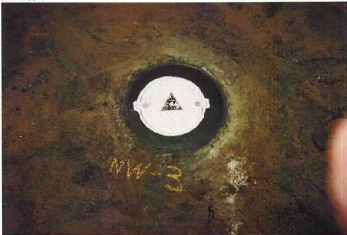
Photo 8: Nested well (NW-3) located along southern border of the Site after installation of traffic box.
