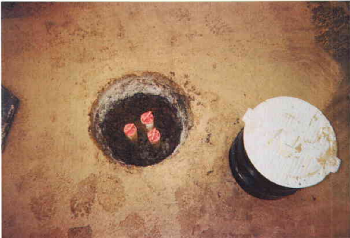
Photo 7: Nested well (NW-1) located along northern border of Site before installation of traffic box.
