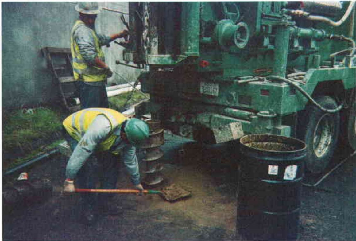
Photo 12: BC 2 Environmental crew during installation of nested well NW-3.
