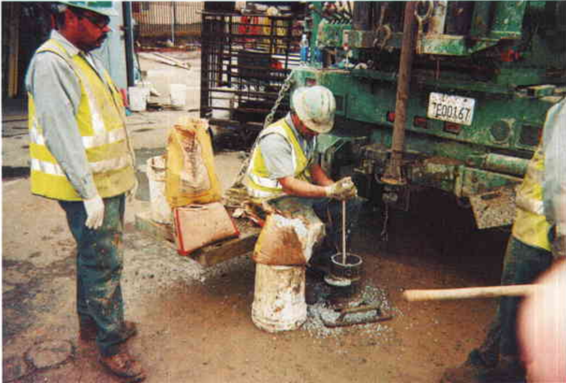
Photo 11: BC 2 Environmental crew during installation of nested well NW-2.
