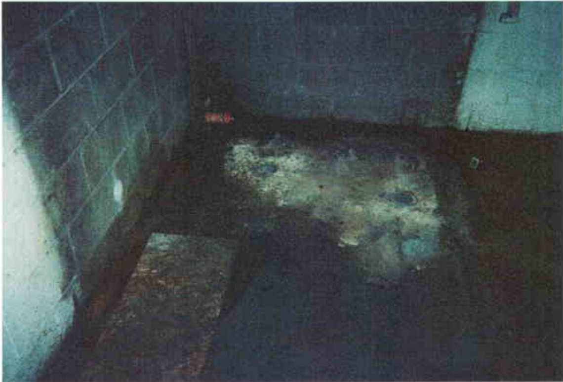
Photo 5: Boring 4BE(10') 4.5-5' at southeastern corner of the pressure wash room inside the manufacturing/office building.
