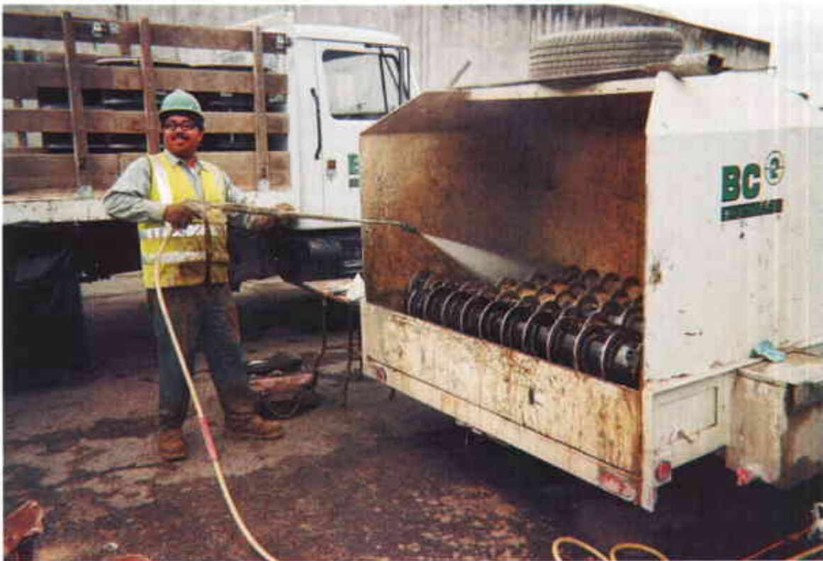
Photo 13: BC 2 Environmental crew steam cleaning augers used for drilling nested wells.
