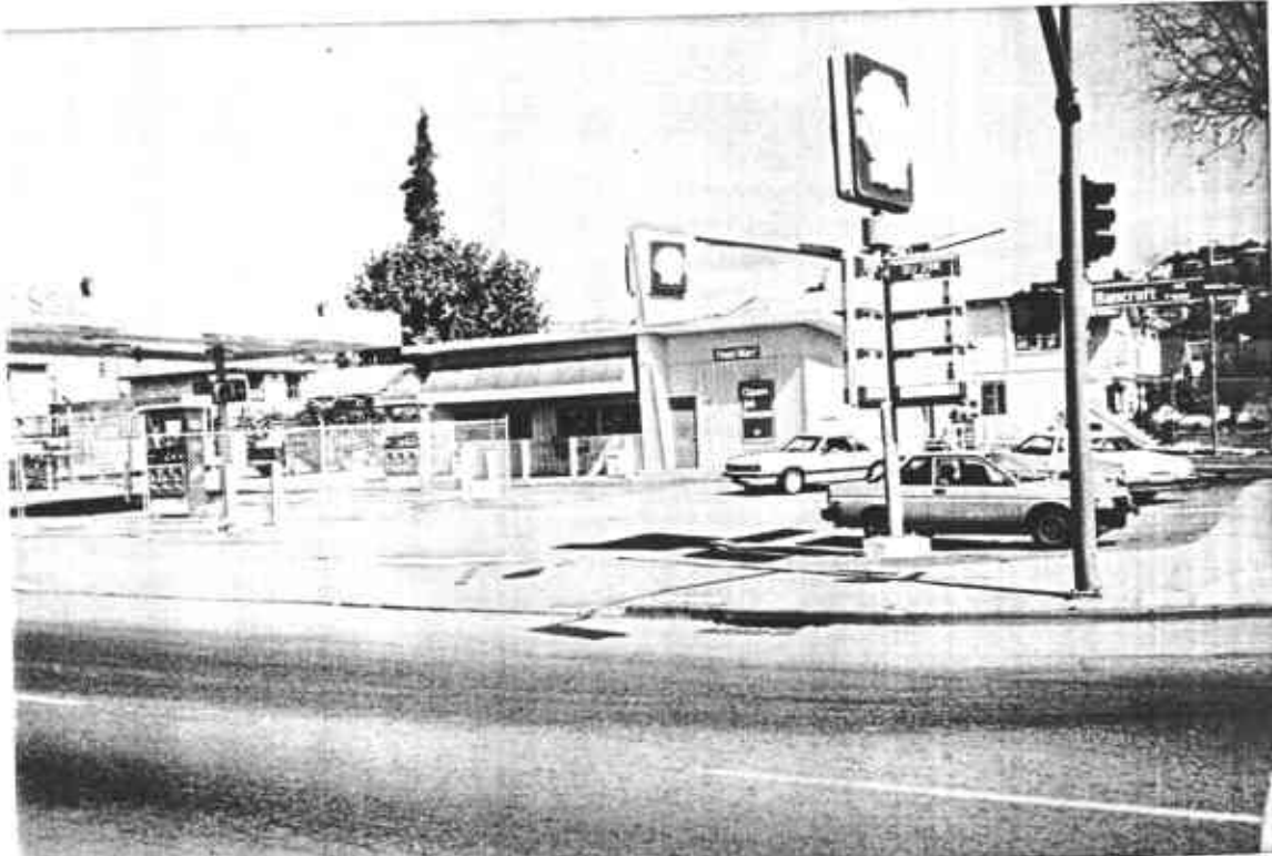
Photo No. 5: Looking northeast at the subject property, UST slab visible in center of photo.
