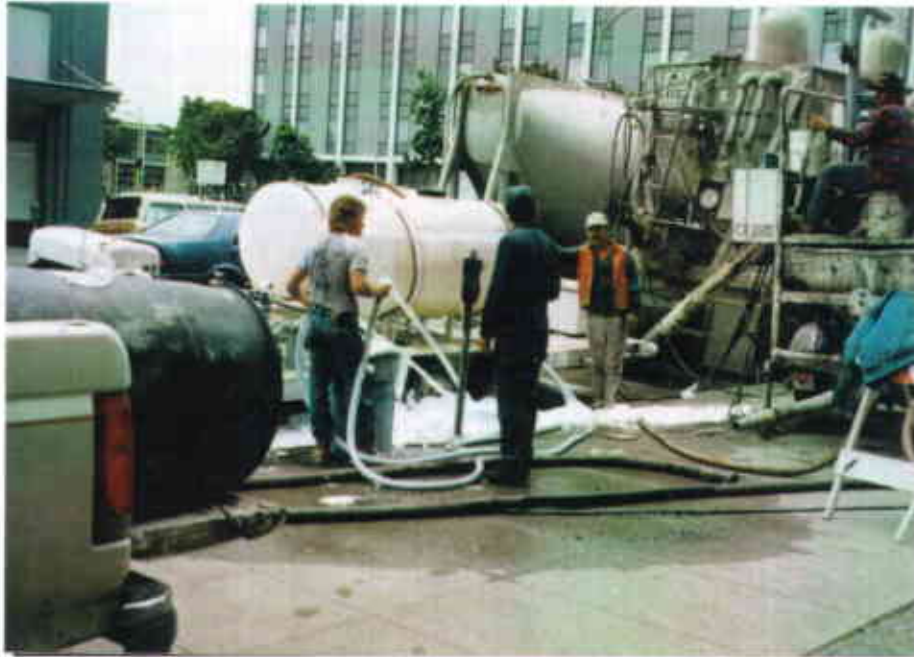
Figure 12: Preparation of concrete.
