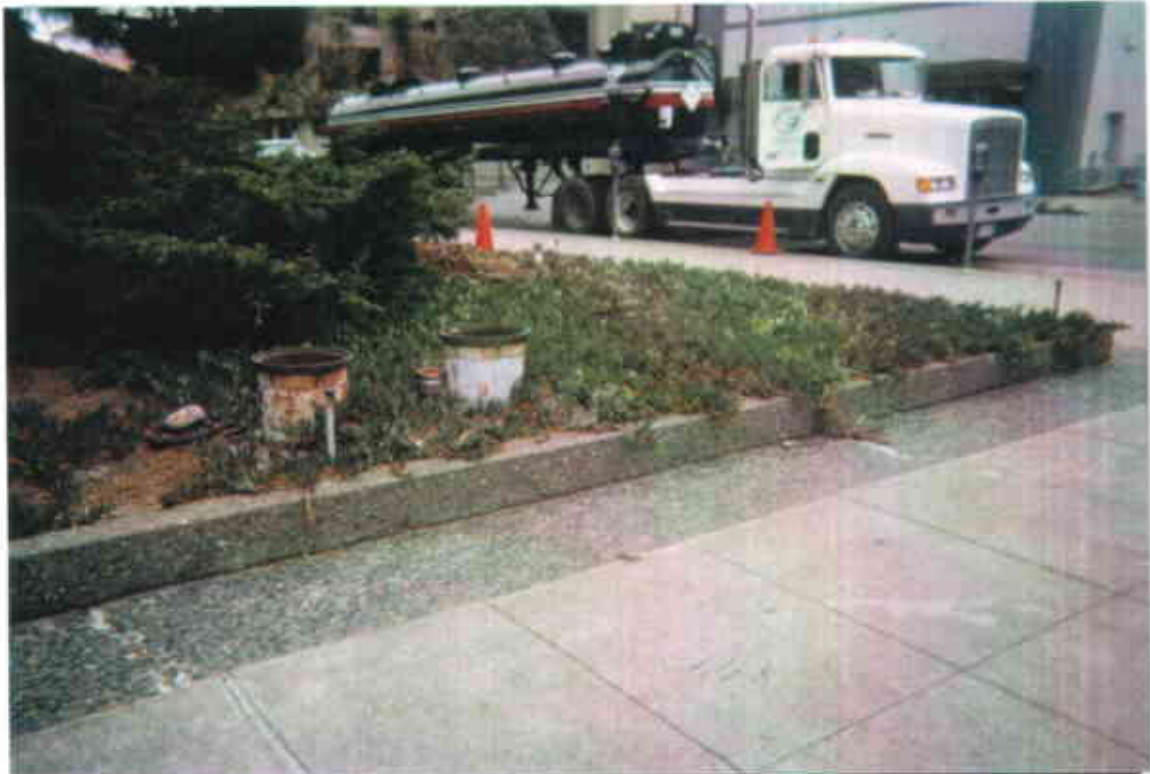
Figure 4: Looking south across subject site. Vapor recovery systems are located inside bucket-shaped steel containers.
