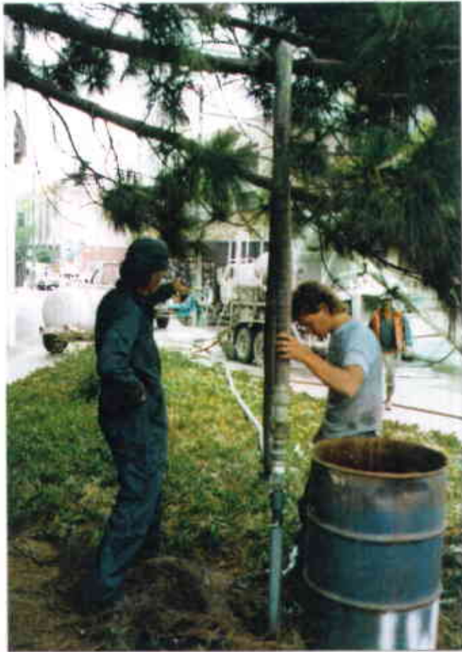
Figure 14: Filling of an UST with concrete through the vent line.
