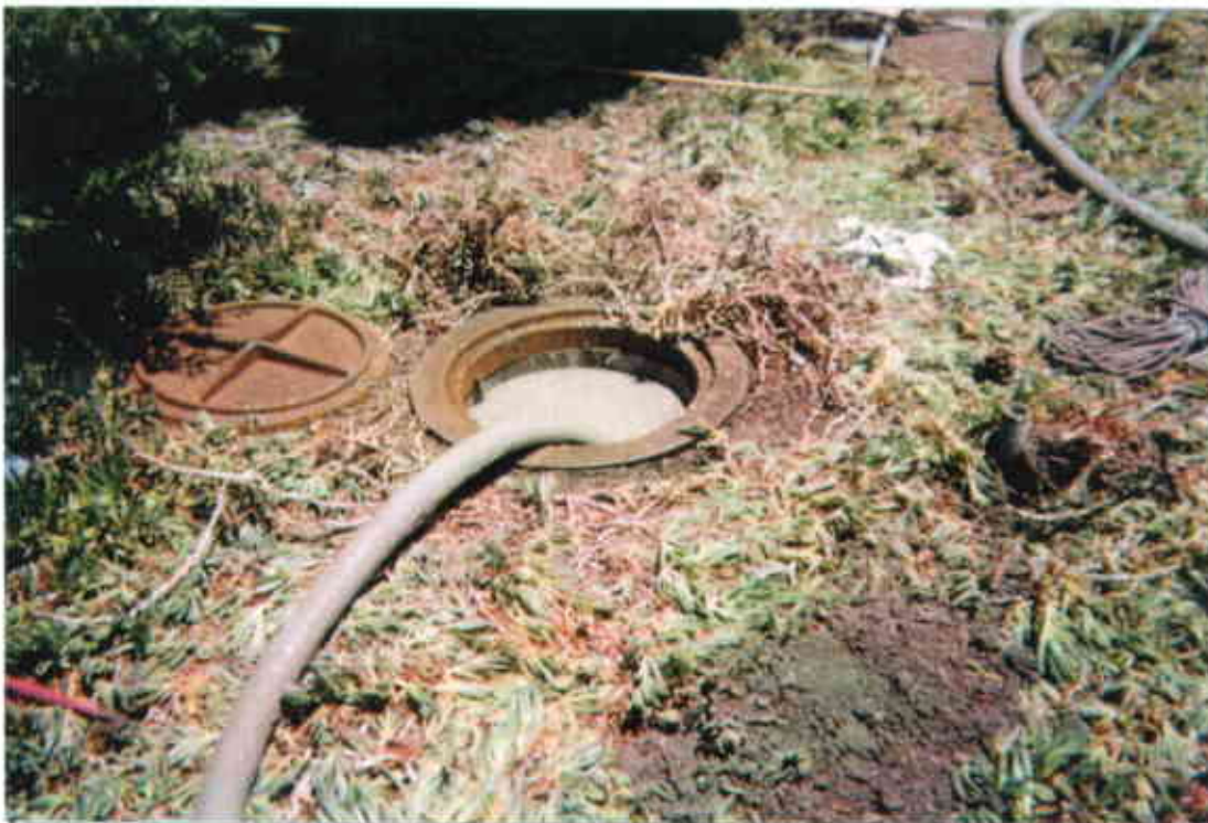
Figure 17: Manway being topped off with concrete.
