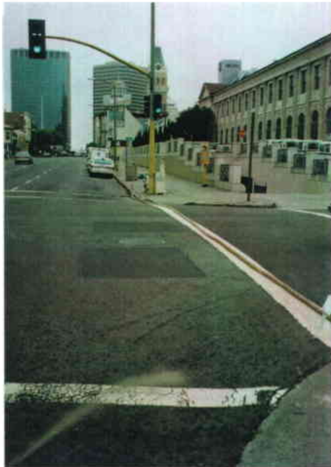
Figure 13: A fire hydrant provided water for the mixing of concrete.
