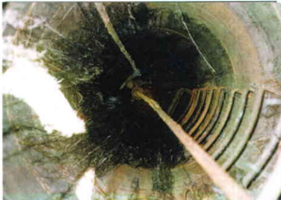
Figure 15: View down manway prior to filling with concrete.
