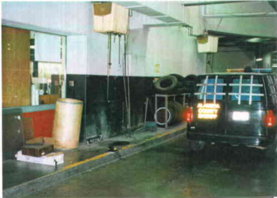
Figure 8: ALCOPARK's basement: dispenser line's riser is at the base of the dip sticks.
