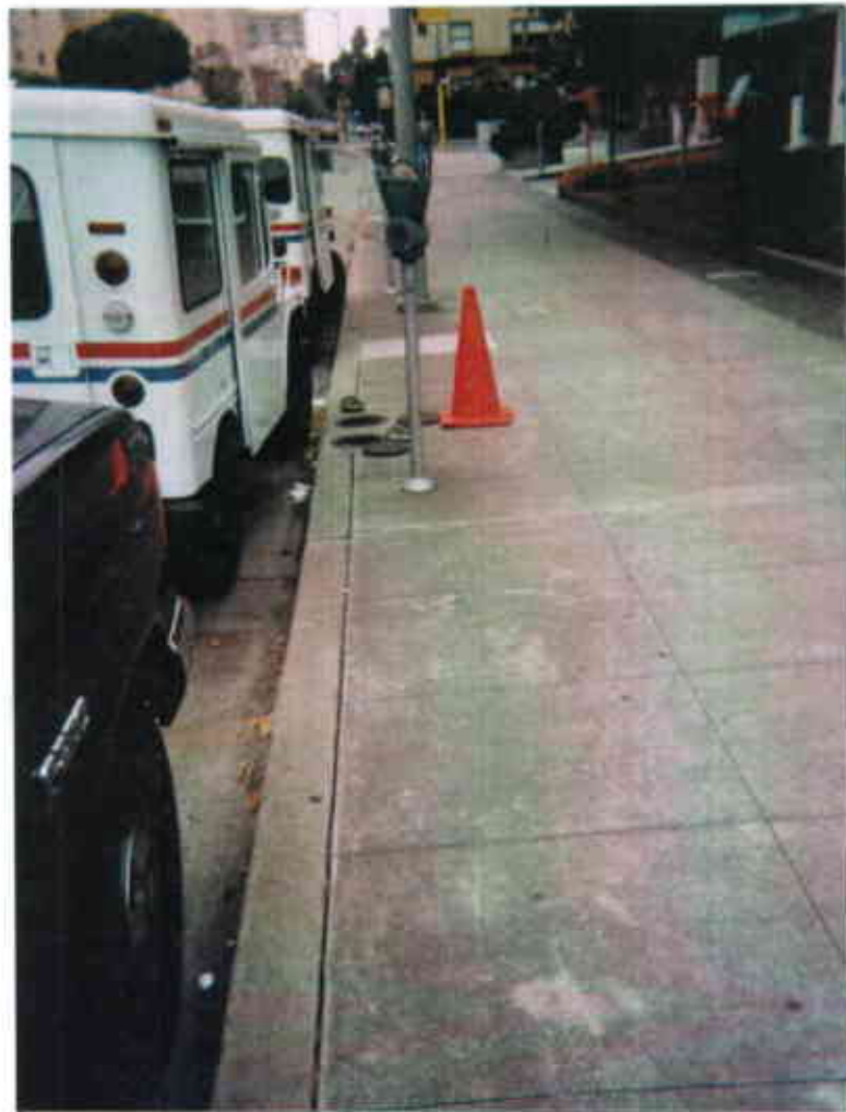
Figure 3: Looking north-east down Jackson Street. Fill lines are visible.
