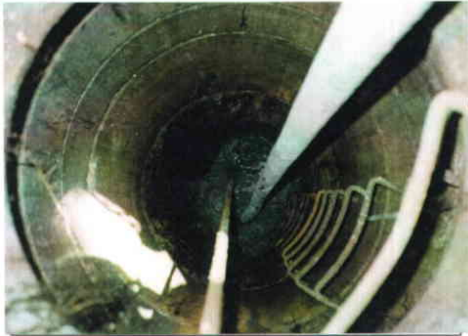
Figure 16: View down manway while being filled with concrete.
