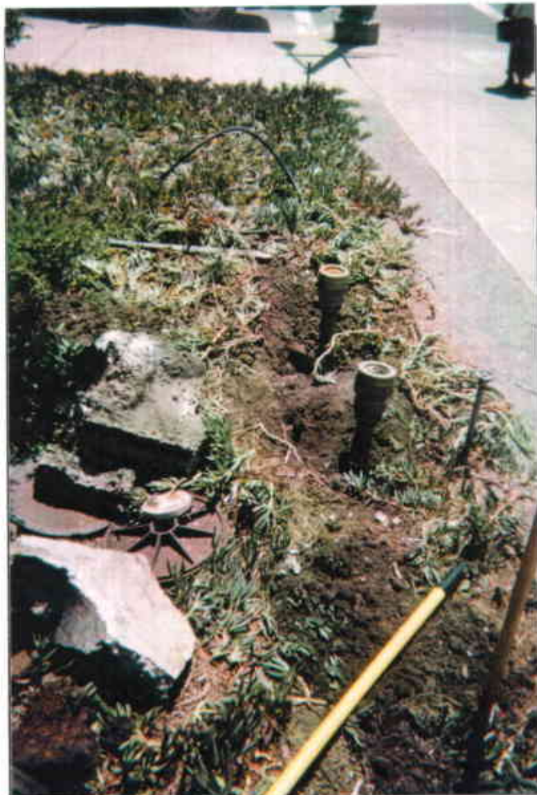
Figure 7: Vapor recovery lines after concrete blocks and steel containers were removed.
