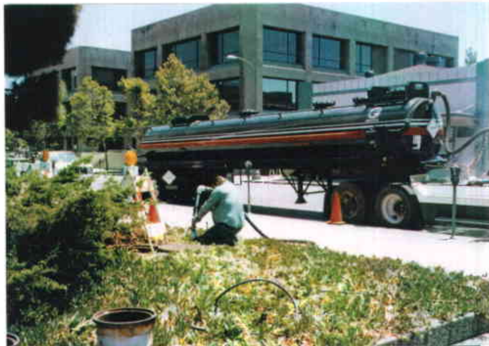
Figure 5: Rinsing and vacuuming of USTs. Vacuum truck visible in background.
