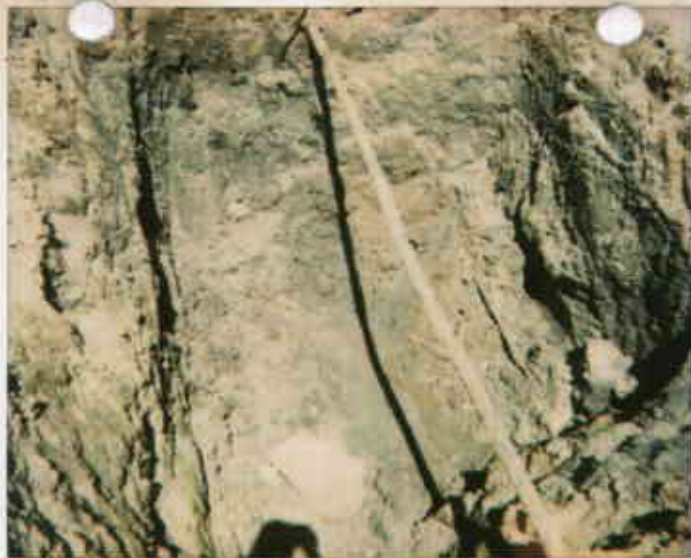
FANKA PO utility + water 2547 E 27th St Present 8/30/94
