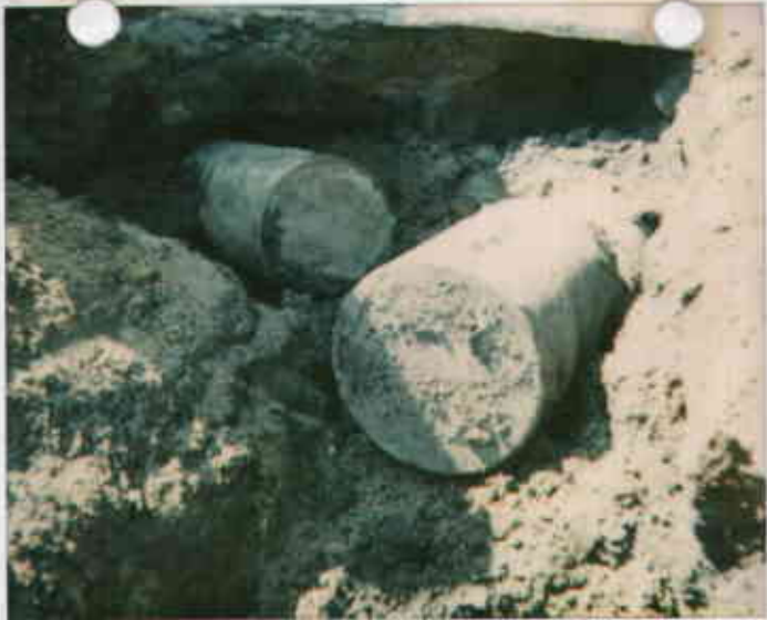
3 - 500 gallon gas tanks (B-D) 8/30/94 2457 E 27th
