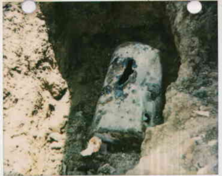
Waste oil tank 8/30/94 2547 E 27th St 1 large hole on top
