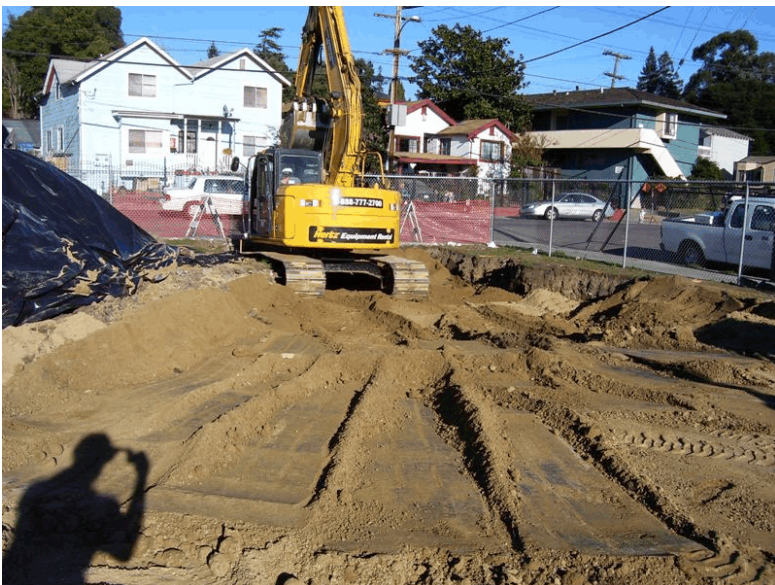
Photograph 15 - View of compacting work.
