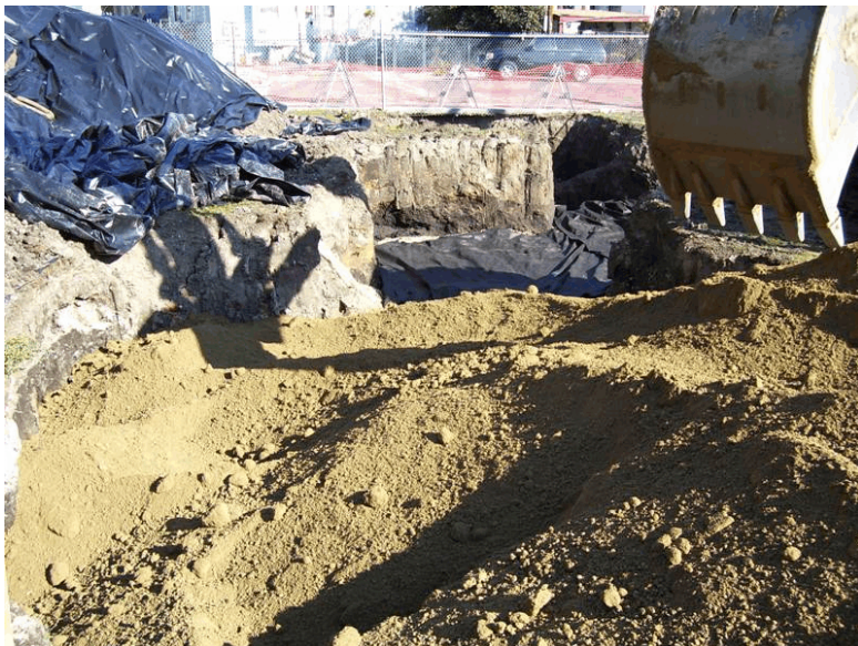
Photograph 12 - Backfill of imported fill material
