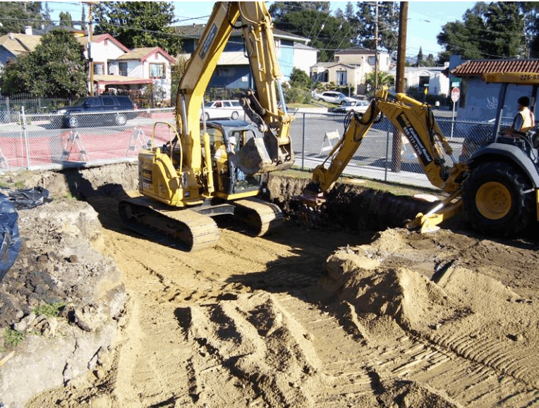
Photograph 14 - View of backfilling and compacting work.
