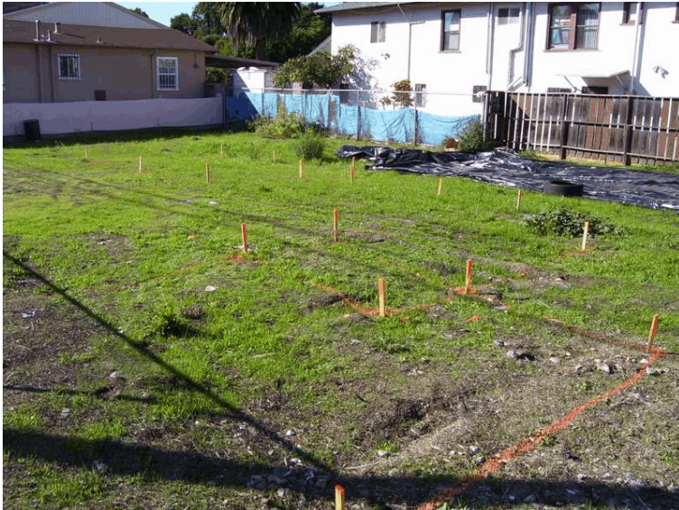
Photograph 2 - Excavation outlines, Areas II and III.
