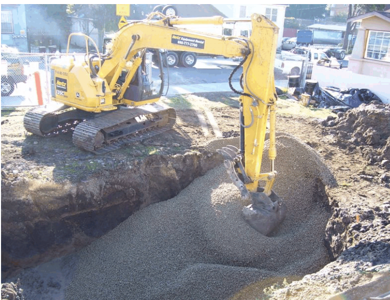
Photograph 9 - Backfilling with quarry materials.
