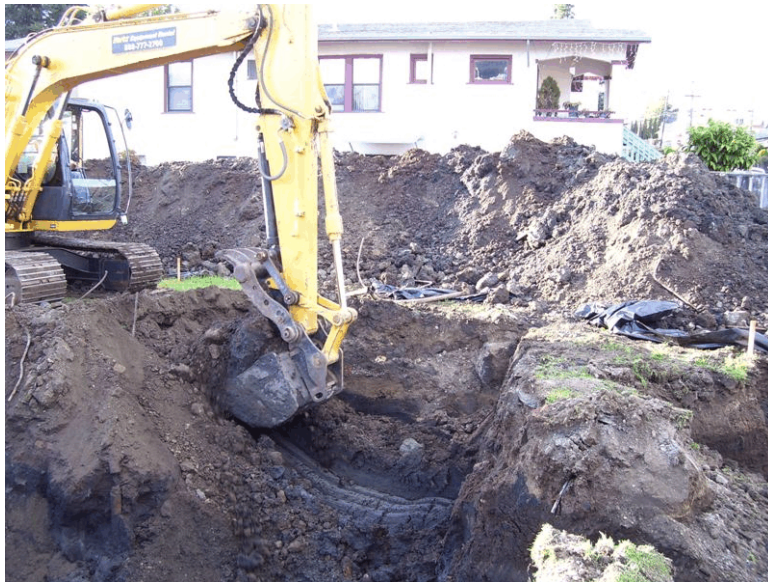
Photograph 5 - Excavation of Area II, in progress. Note stained soil being removed.
