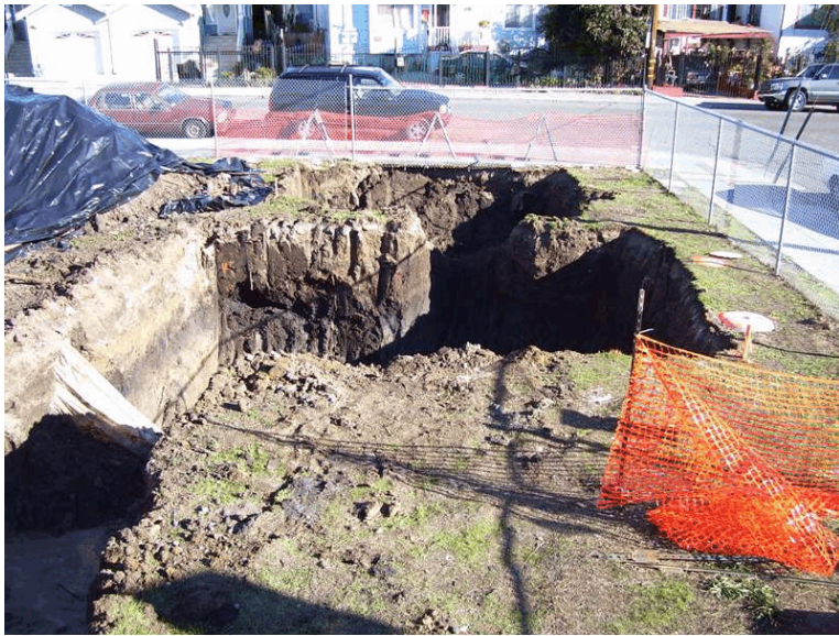
Photograph 7 - View of the extent of excavation of Area I and II.
