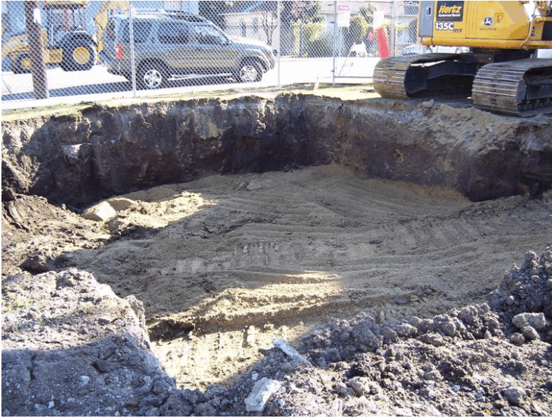
Photograph 13 - View of partially backfilled excavation.
