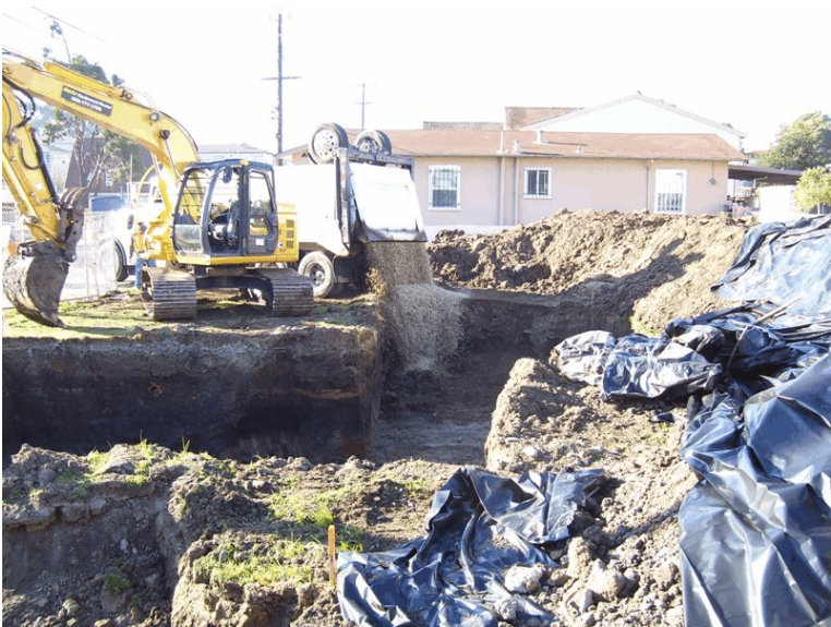
Photograph 8 - View of initial backfilling of Area III.
