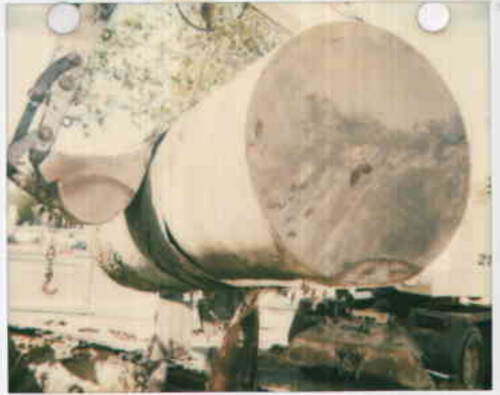
10K Super tank 9800 E 14th Ave 10/30/91, tar wrapped paper peeling
