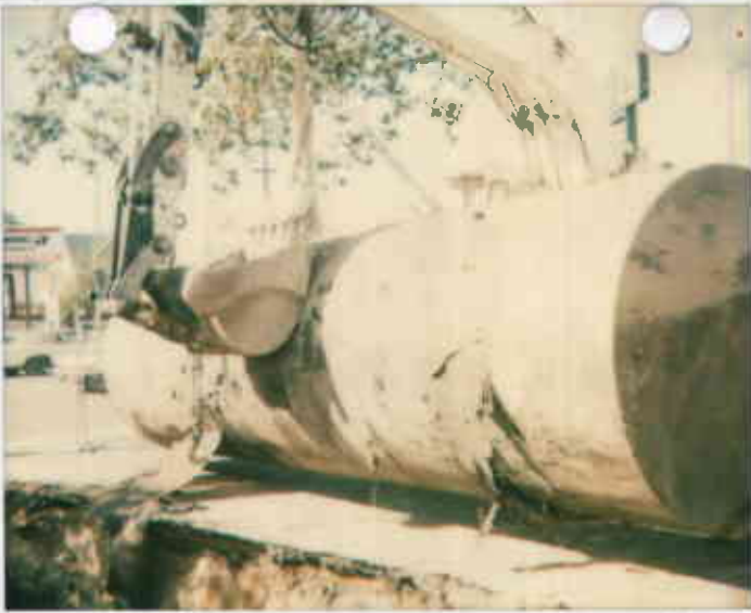
10K Reg Tank - wrapping emergency tank 9800 E 14th Ave
