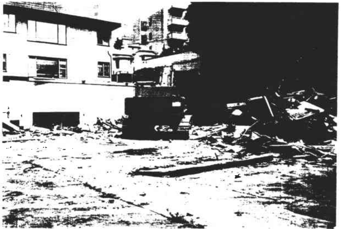
Photo 1: Debris resulting from demolition of building.
