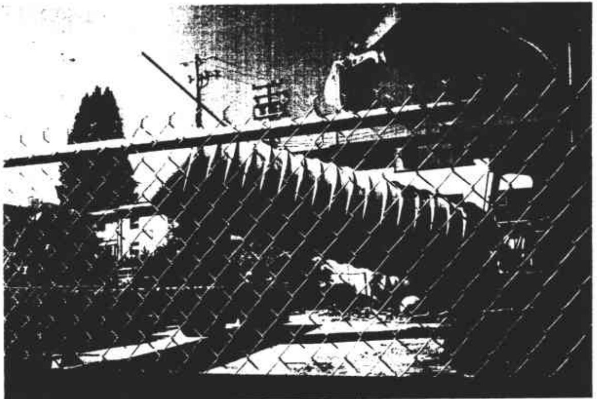
Photo 12: Loading UST onto flatbed truck for removal from site.
