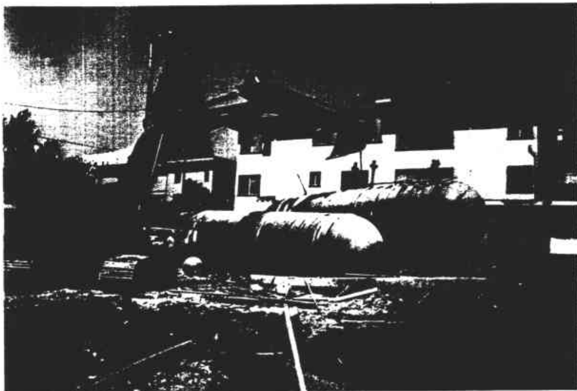
Photo 8: Tanks #2 and #3 after removal from excavation.
