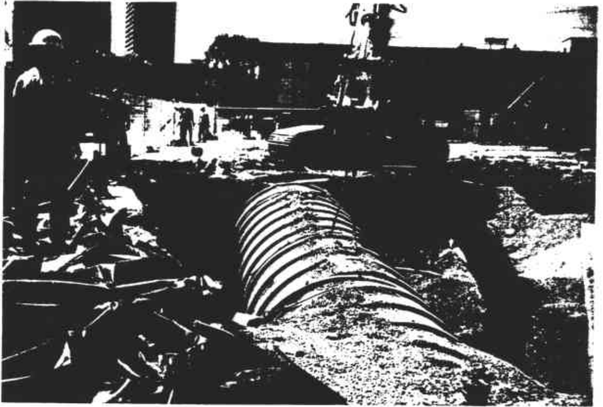
Photo 11: Removing Tank #1 from excavation.
