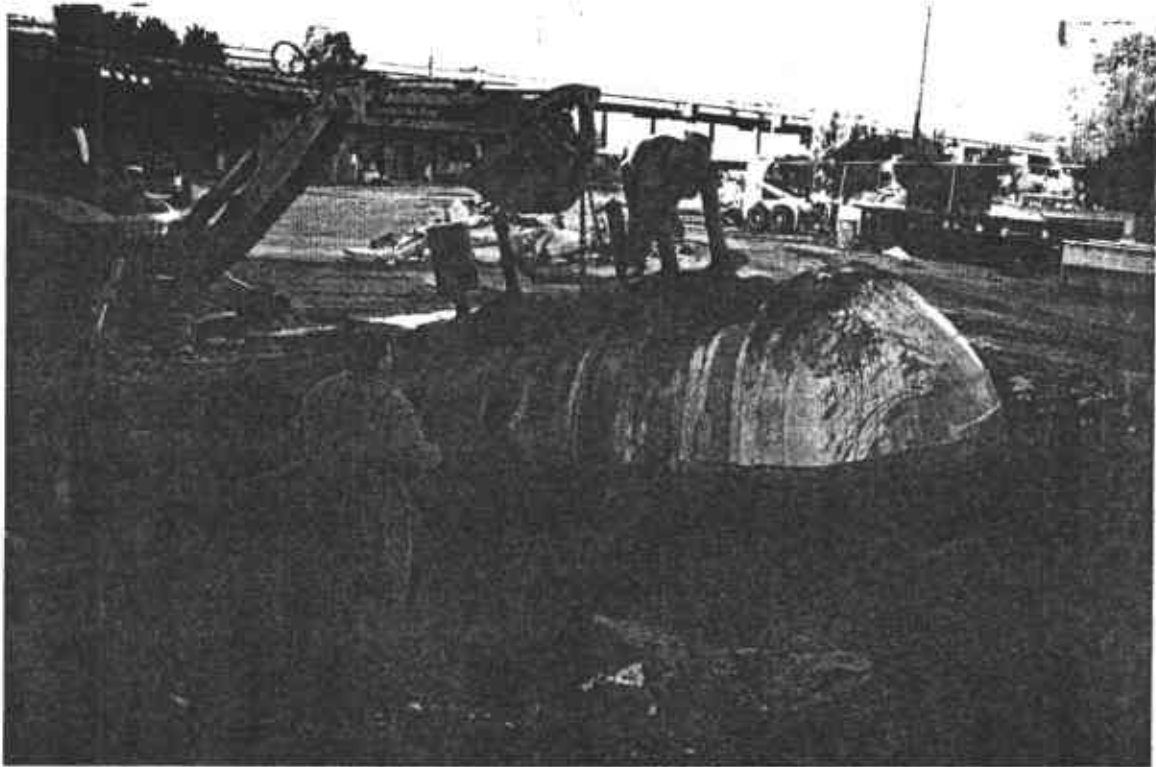
Photograph 4: Removal of Tank No. 2 (Middle Tank)
