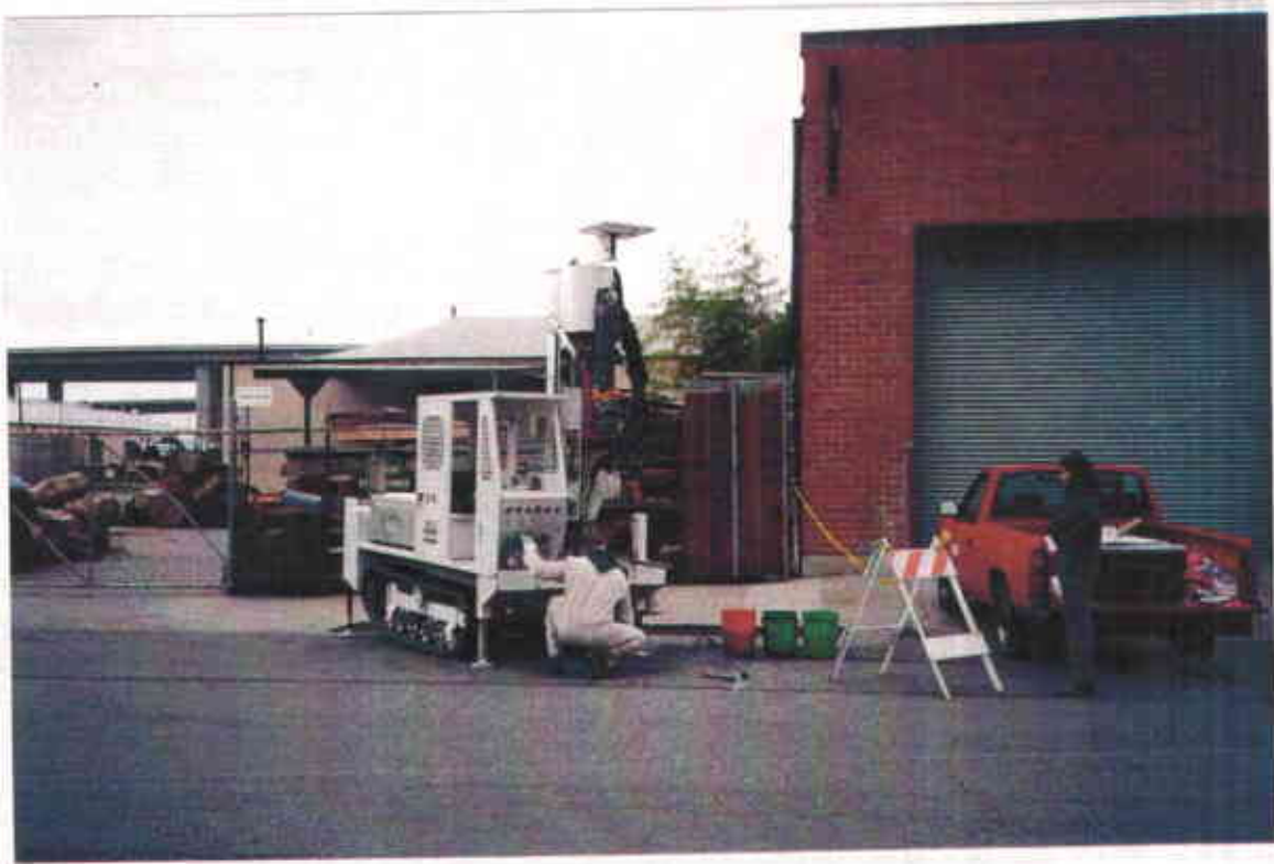
Photograph 1 View of Rhino drill rig during the installation of SB-8.
