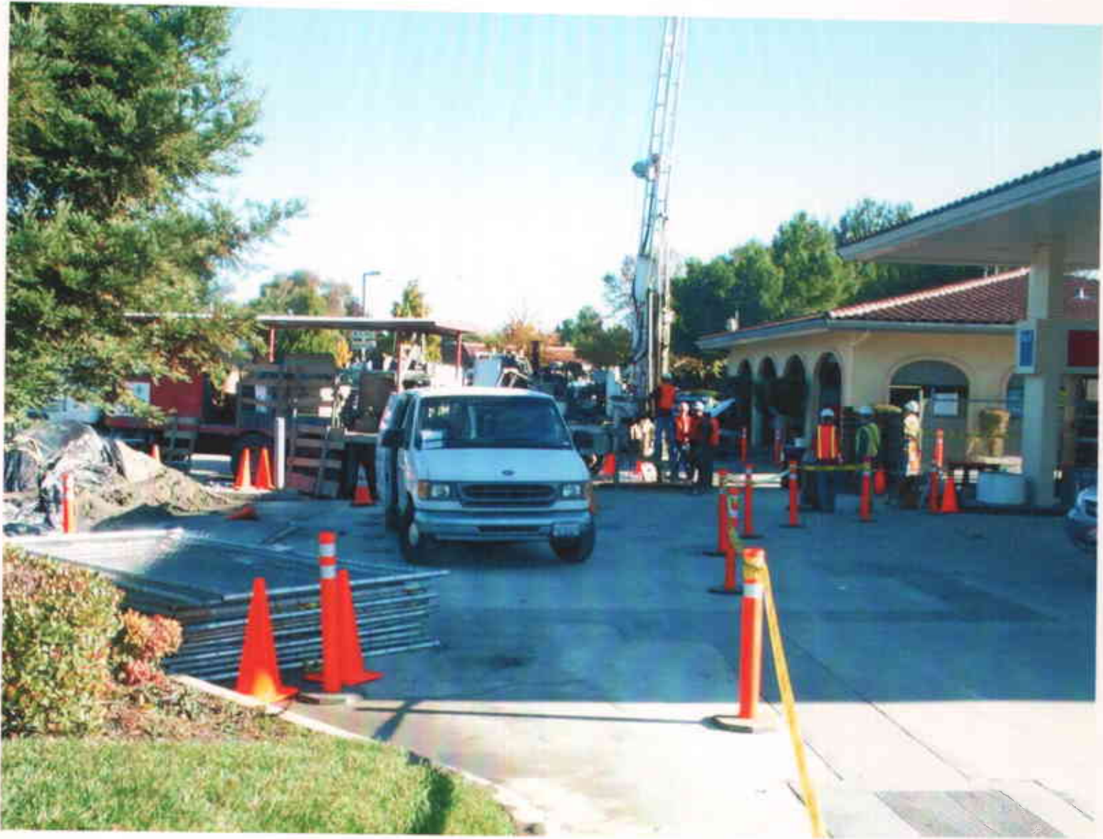
Drilling well MW-9A
