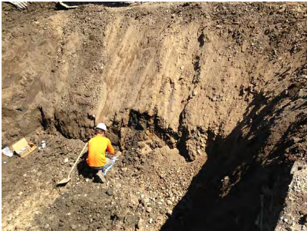
Excavation 2 - overexcavation of the north wall; looking towards the north
