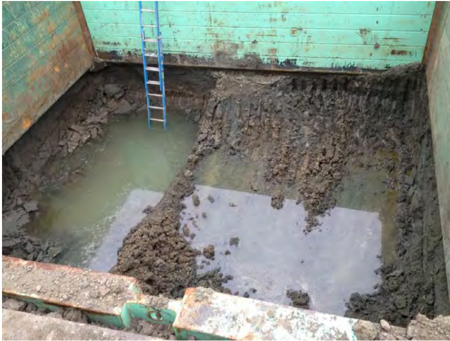
Excavation 1-looking towards the east at approximately 11 feet bgs
