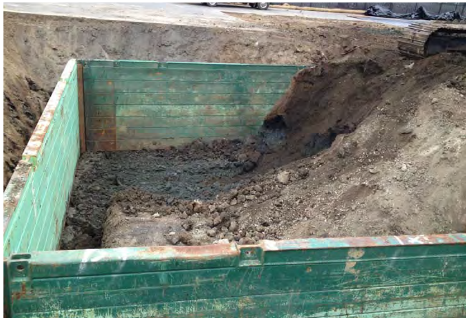
Excavation 1 - looking towards the south with shoring installed.
