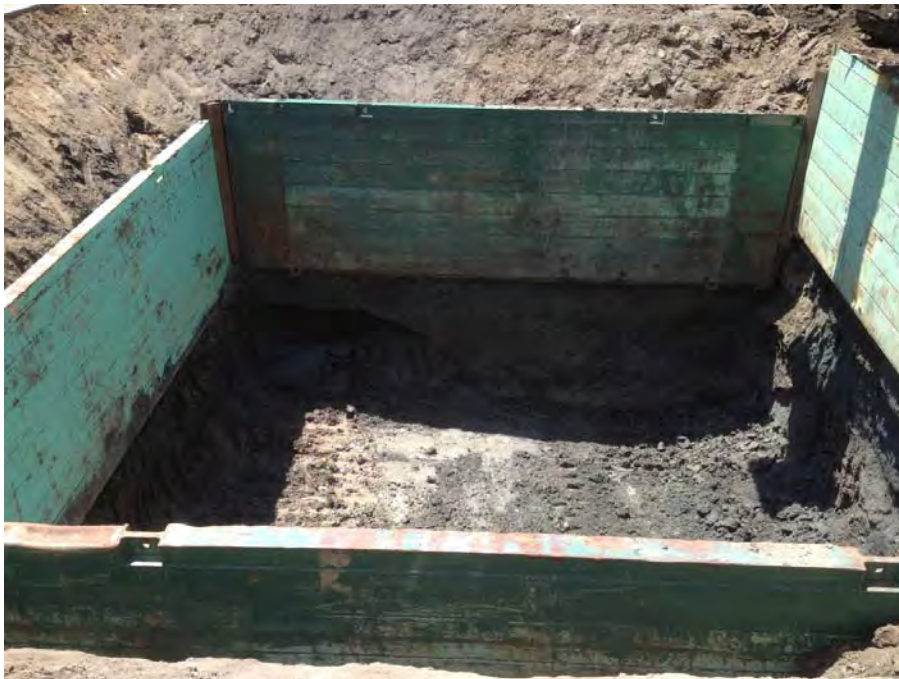
Excavation 1 – final excavation at 17 feet bgs looking towards the south.
