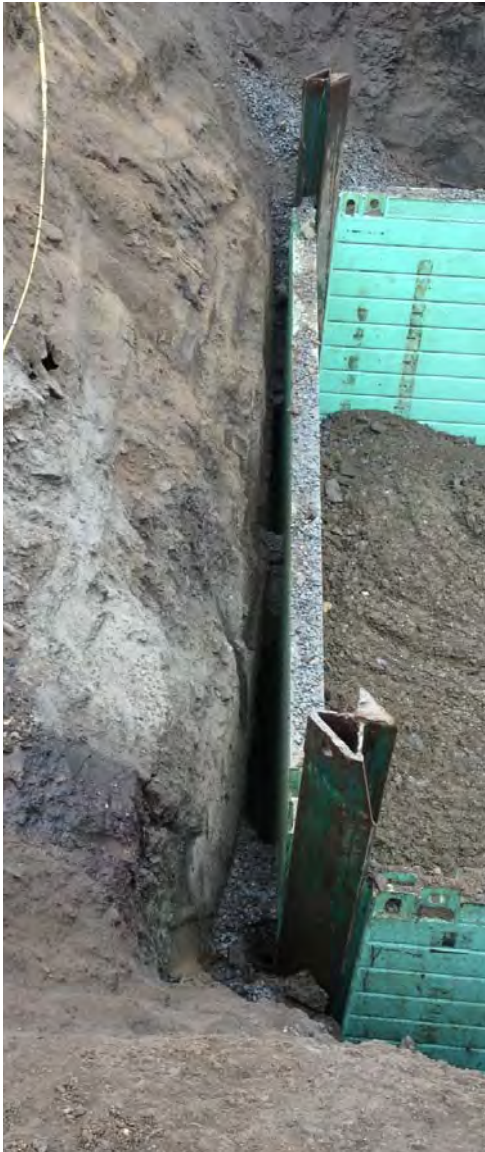
Excavation 2 - looking towards the north prior to any overexcavation.
