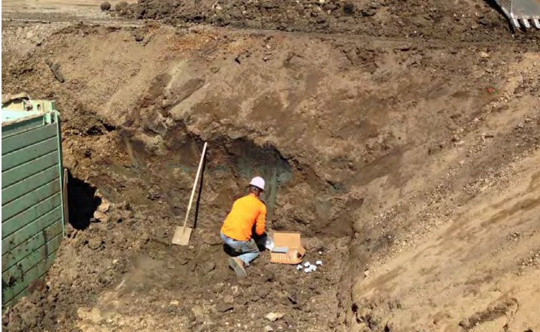
Excavation 2 - overexcavation of the north wall; looking towards the west
