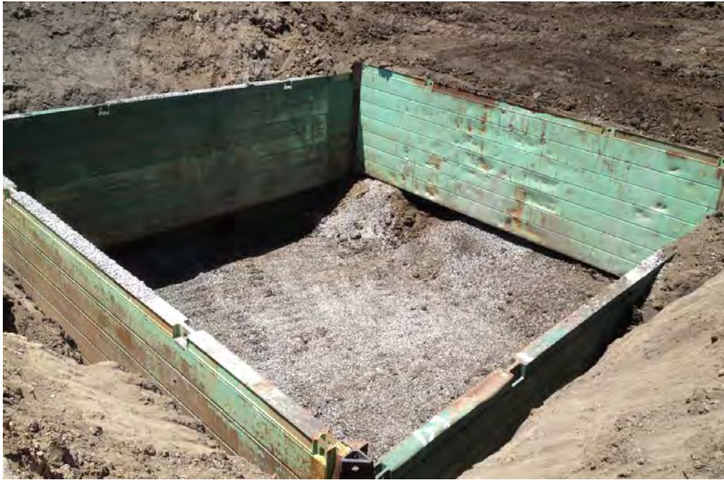
Excavation 1-looking towards the southwest. Approximately 2.5 to 3 feet of drainrock backfill.
