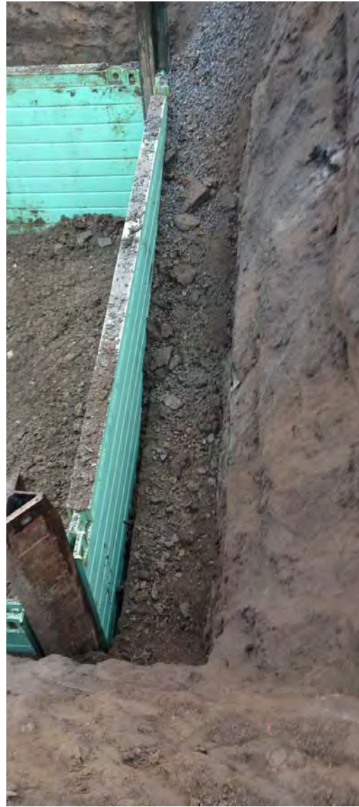
Excavation 2 - looking towards the east
