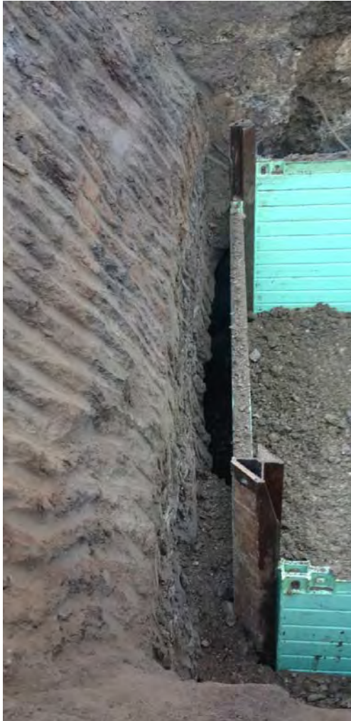
Excavation 2 - looking towards the south
