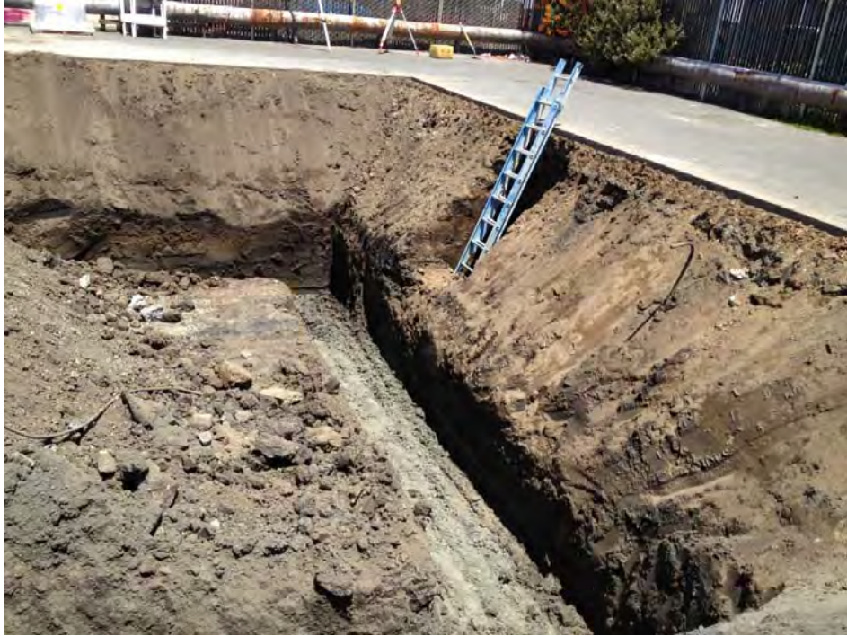
Excavation 1-excavating for shoring installation.
