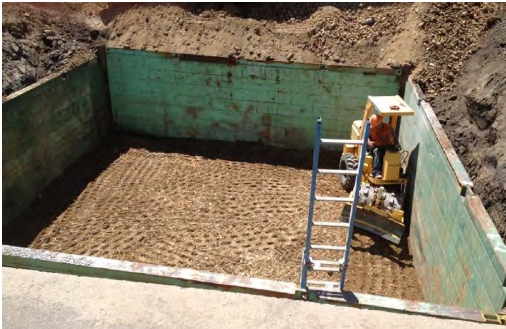
Excavation 1 – Compacting 4-inch minus backfill; looking towards the west.
