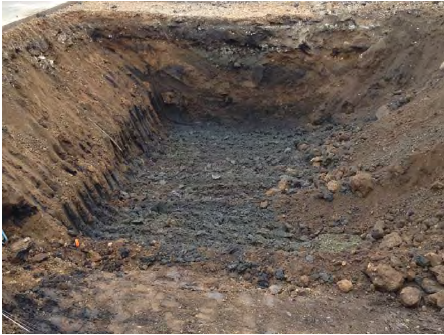
Excavation 1 - looking towards the southeast approximately 9 feet bgs.
