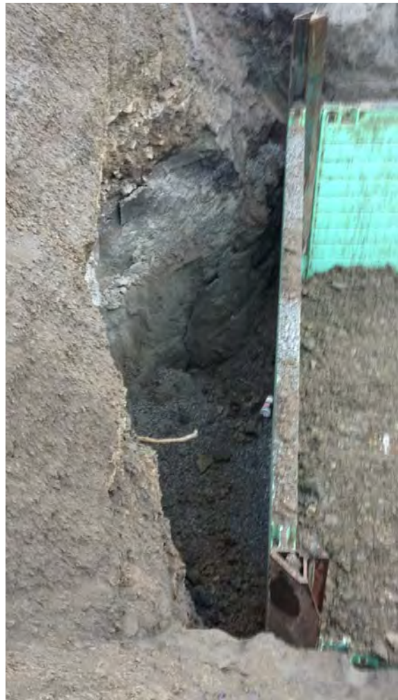
Excavation 2 - looking towards the west
