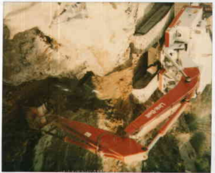
- east wall of excavation
