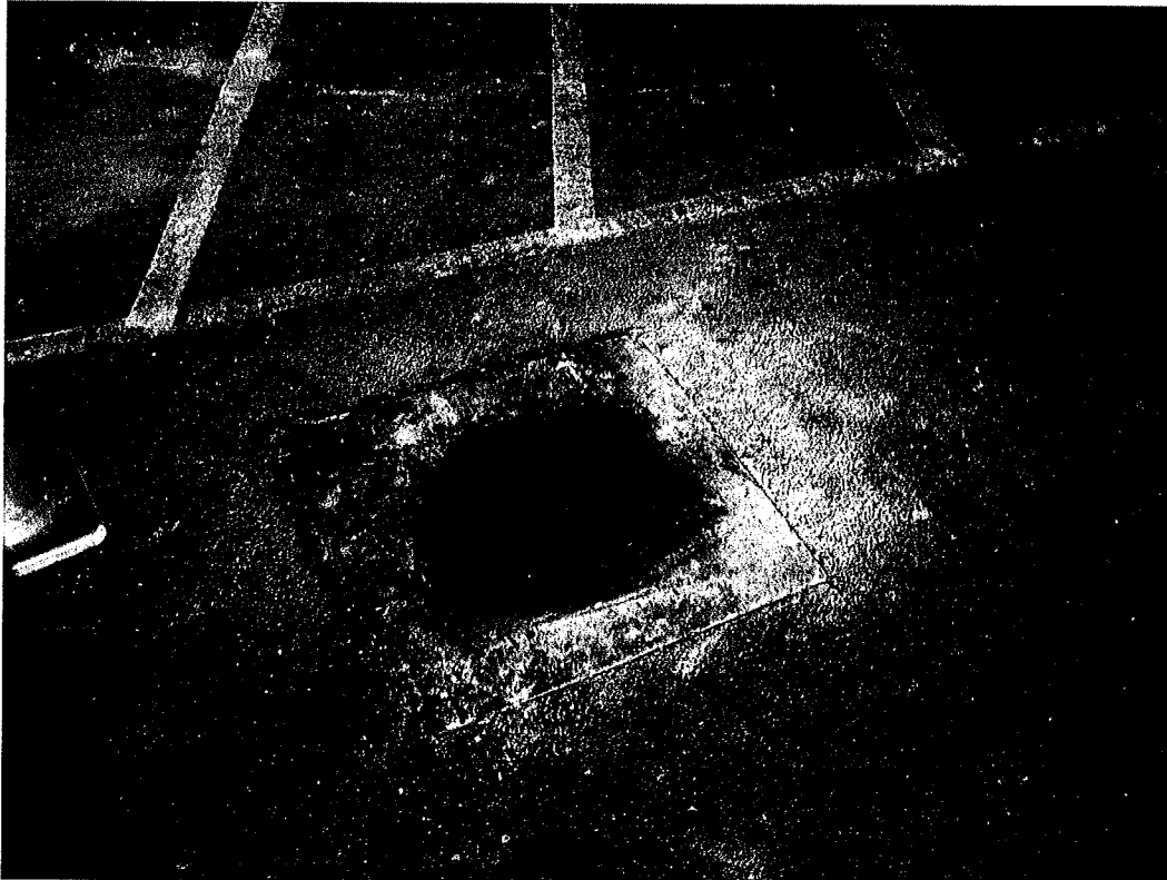
Well RE-2 After Abandonment
