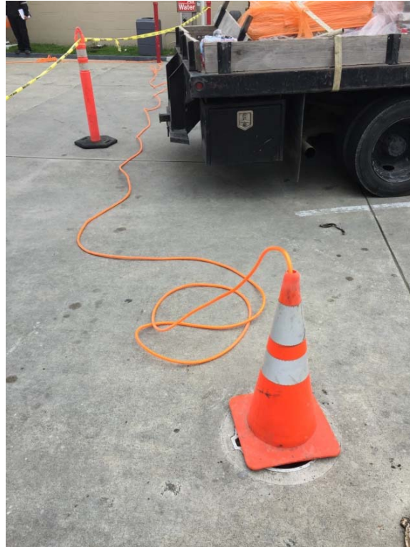
Plate4 Applying Pressure to Complete Pressure Grouting
