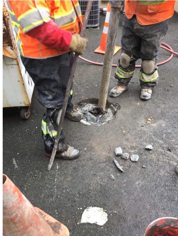
Plate6 After Pressure Grouting Removing Well Box
