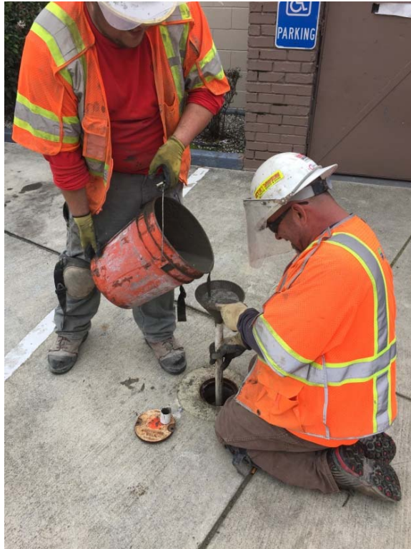
Plate3 Pouring Cement into the Well
