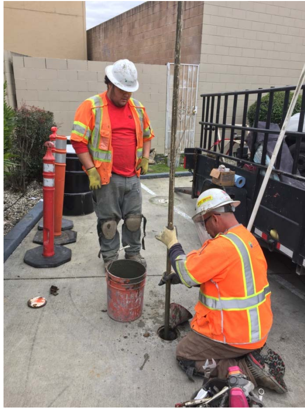
Plate1 Pouring Cement into the Well
