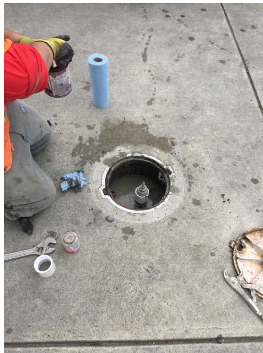
Plate2 Gluing Connector to the Top of Casing for Applying Pressure
