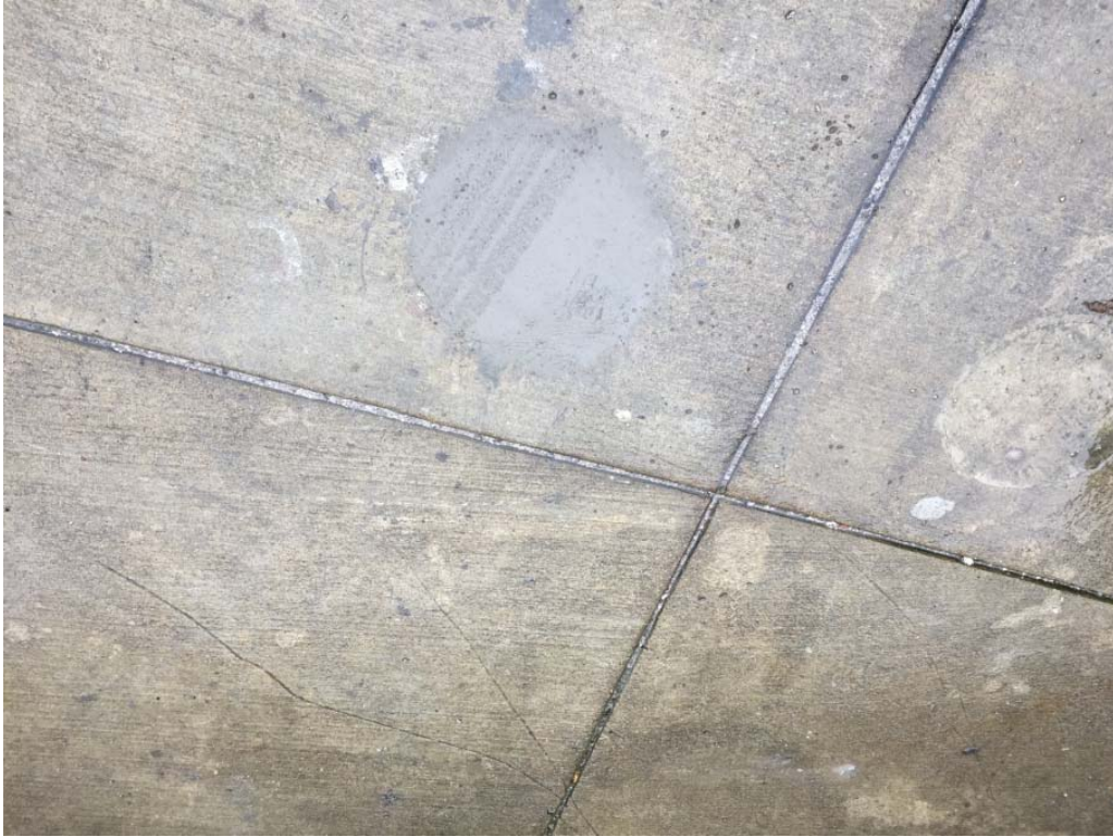
Plate7 Finished Decommissioned Well
