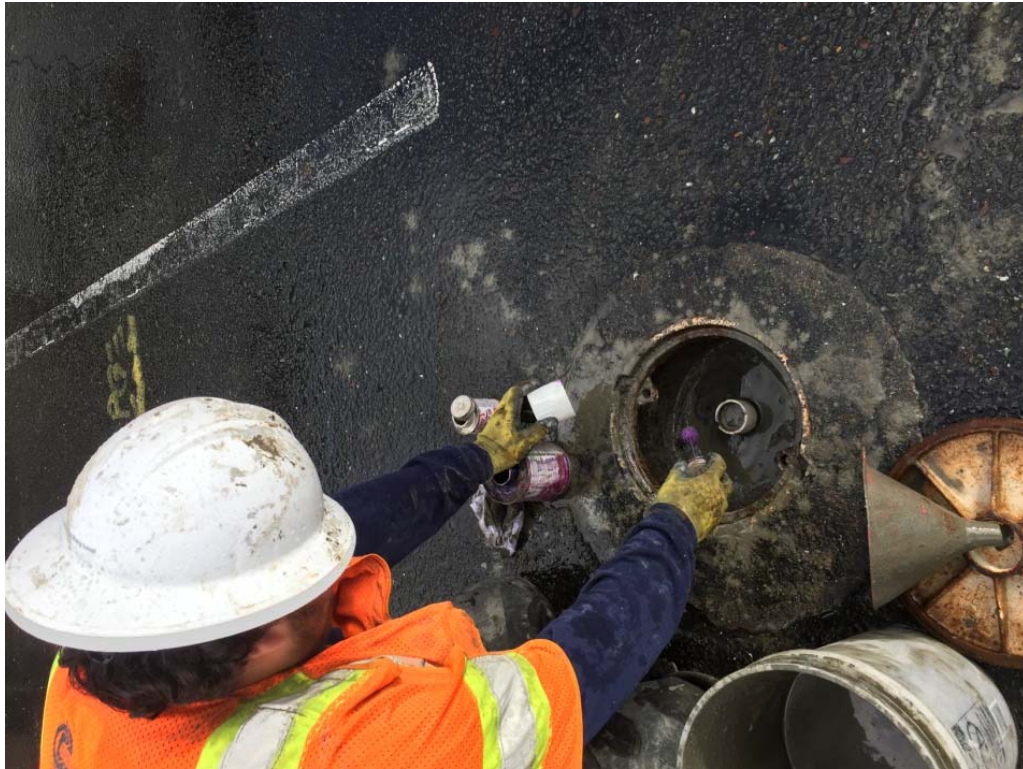
Plate5 Gluing PVC Connector to the Top of Casing for Pressure Grouting
