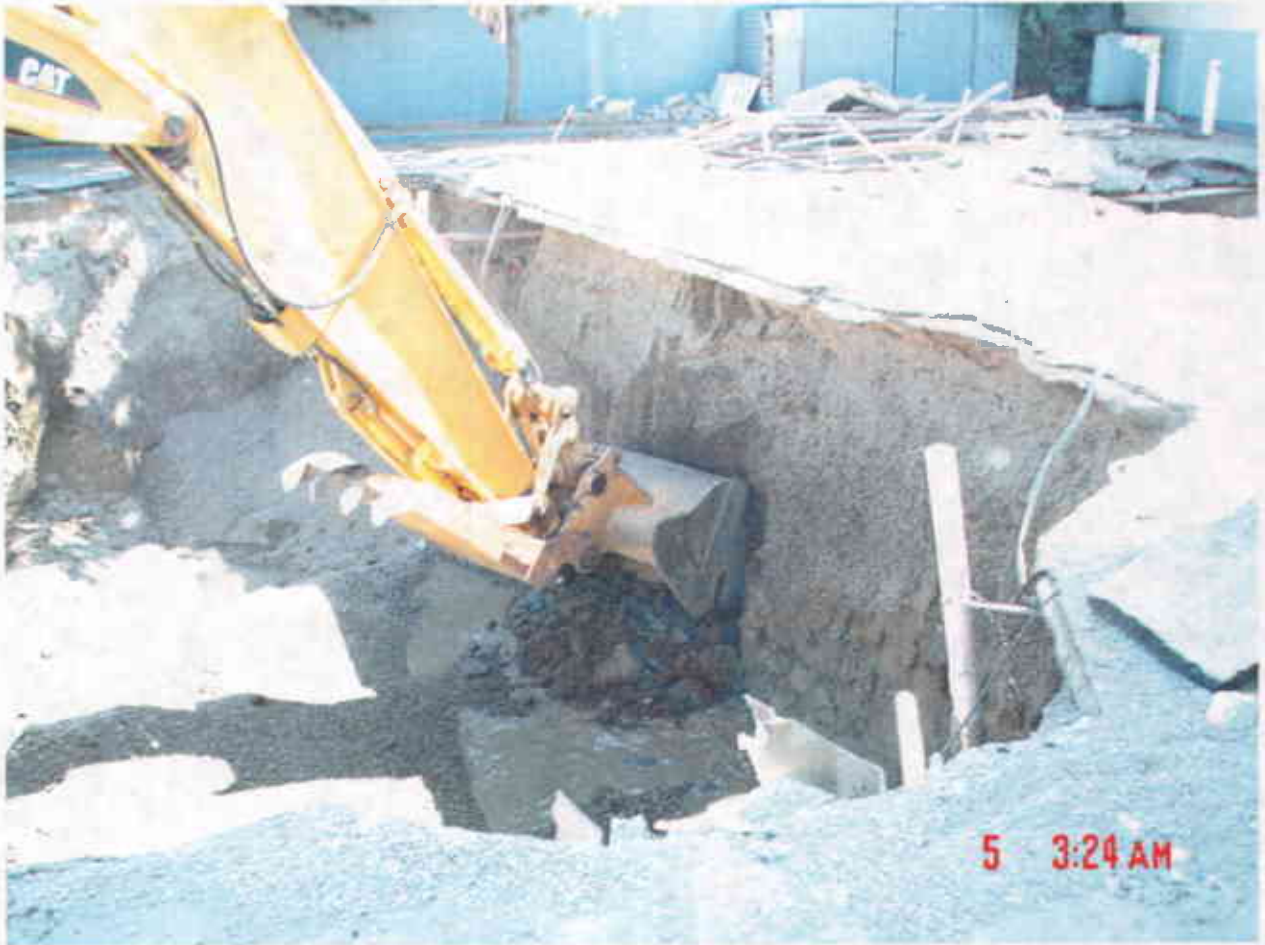
Plate 19: View Southeast showing collection of southwest sidewall sample from capillary fringe with groundwater pooling at bottom of former UST pit.
