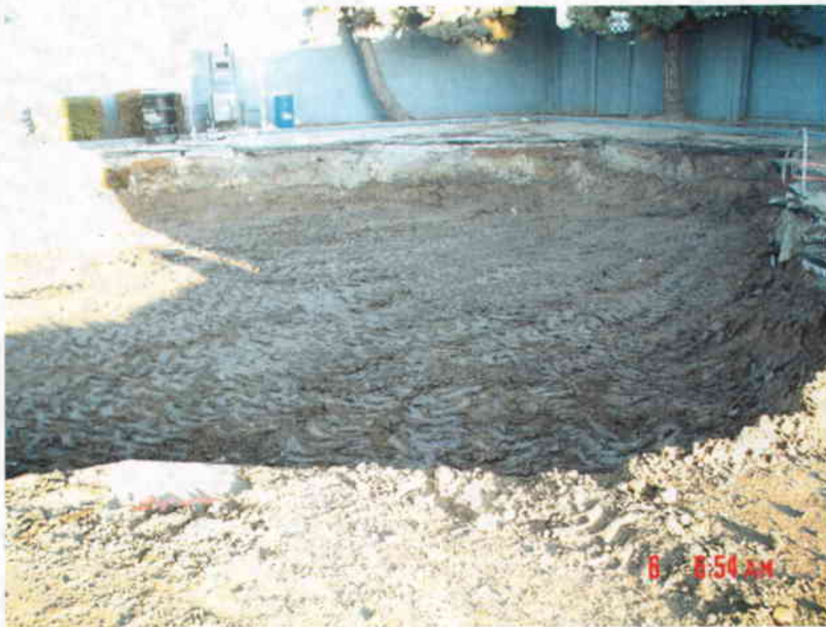
Plate 29: View Southwest showing final compacted surface of sandy backfill.
