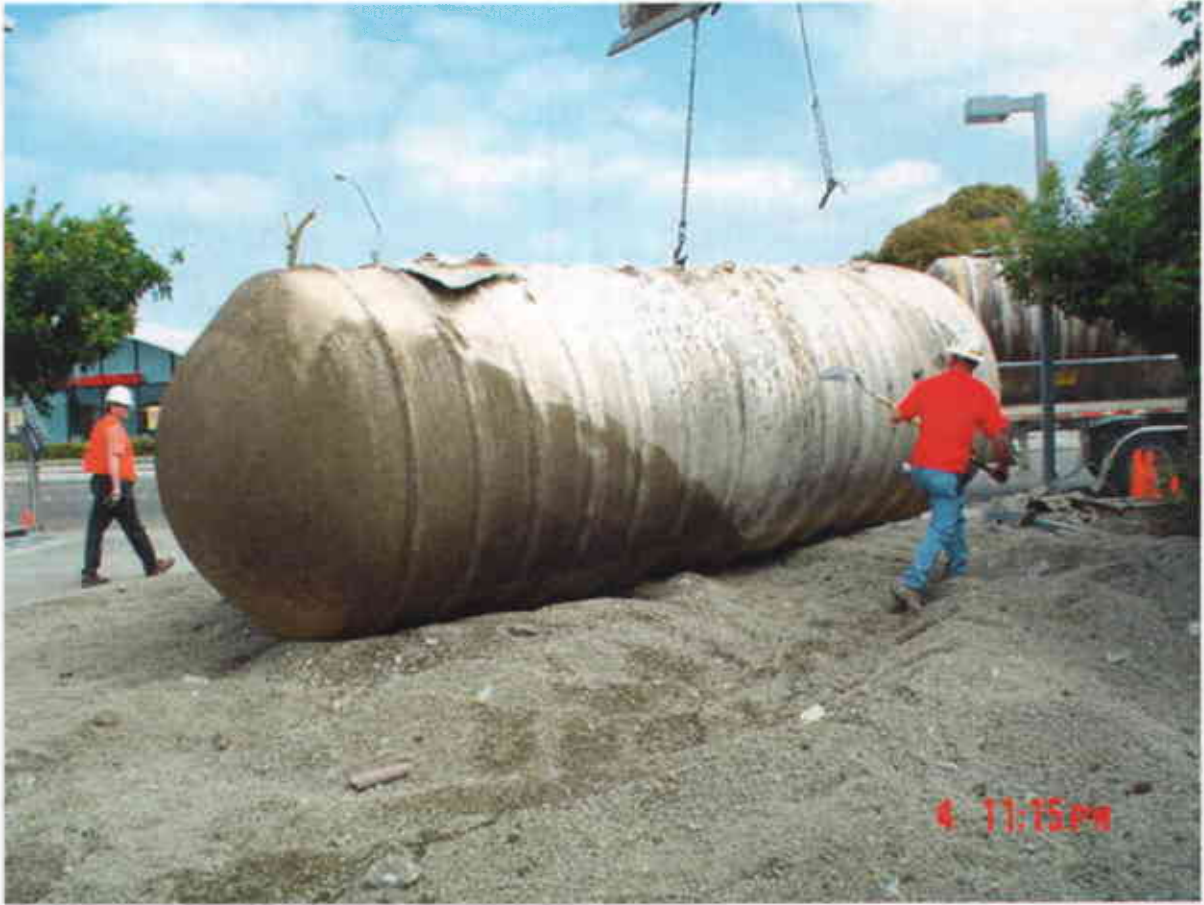
Plate 15: View Northeast showing cleaning of UST#1 before inspection by ACHCSA inspector.
