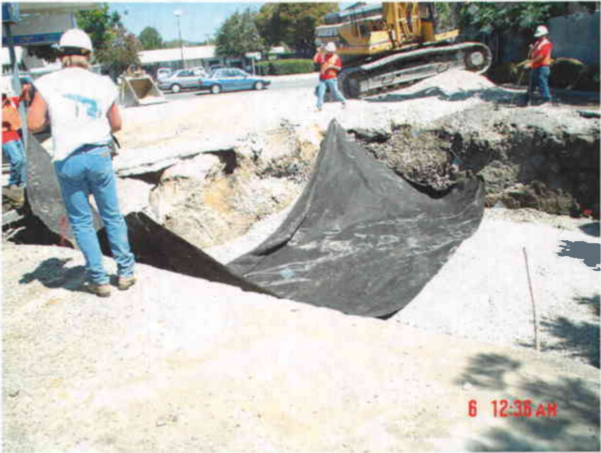
Plate 24: View North showing emplacement of filter fabric over compacted drain rock.
