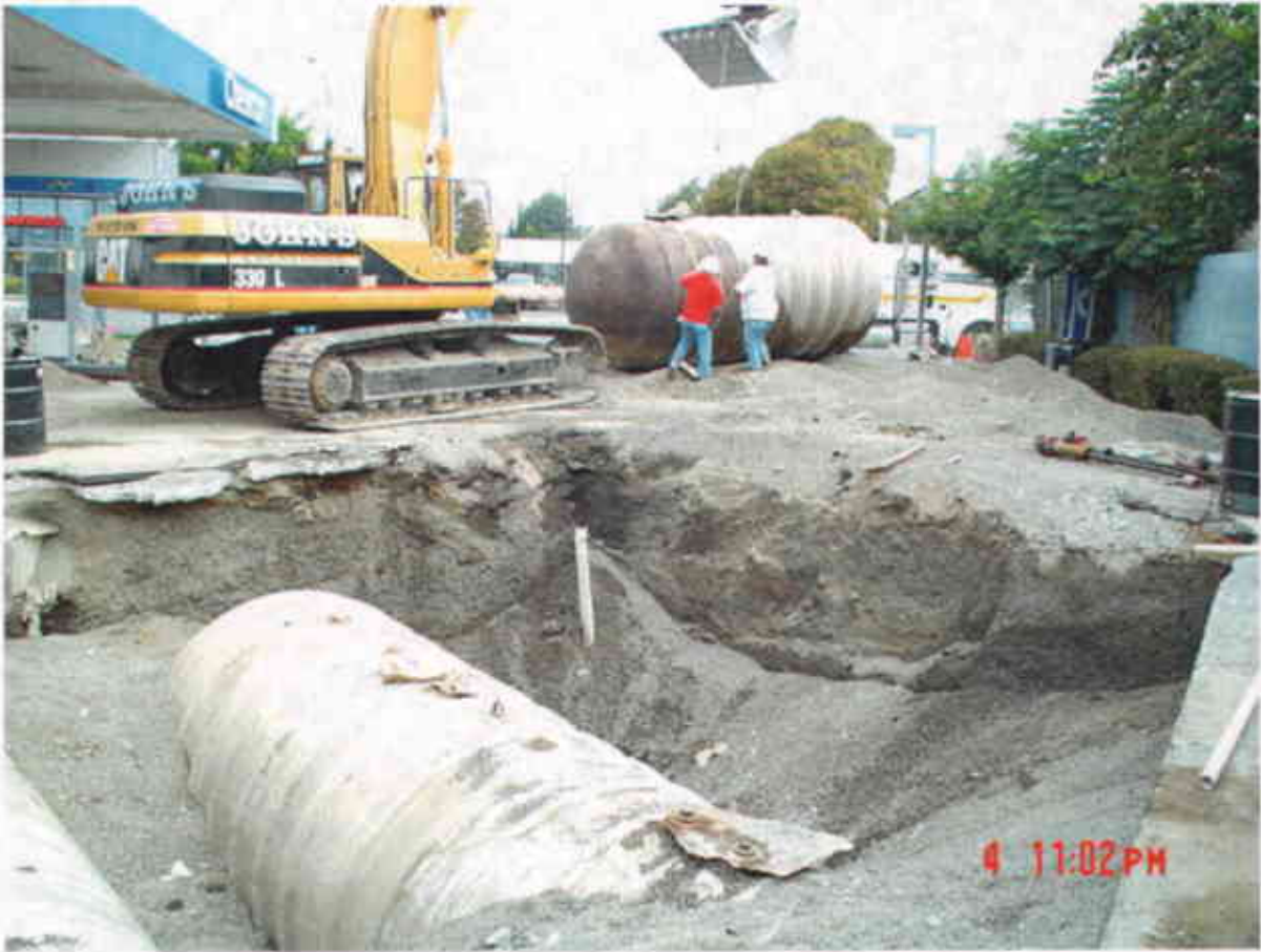
Plate 14: View North showing removal of UST #1.
