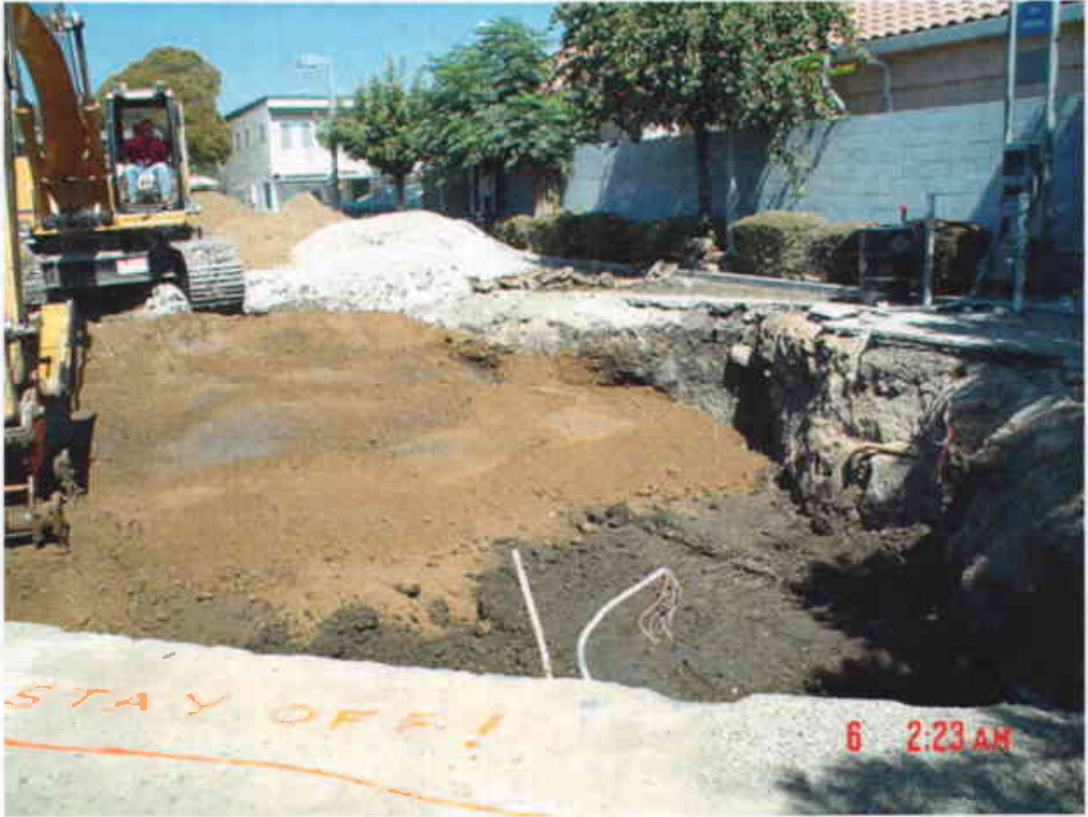
Plate 27: View North showing emplacement and compaction of imported sand backfill.
