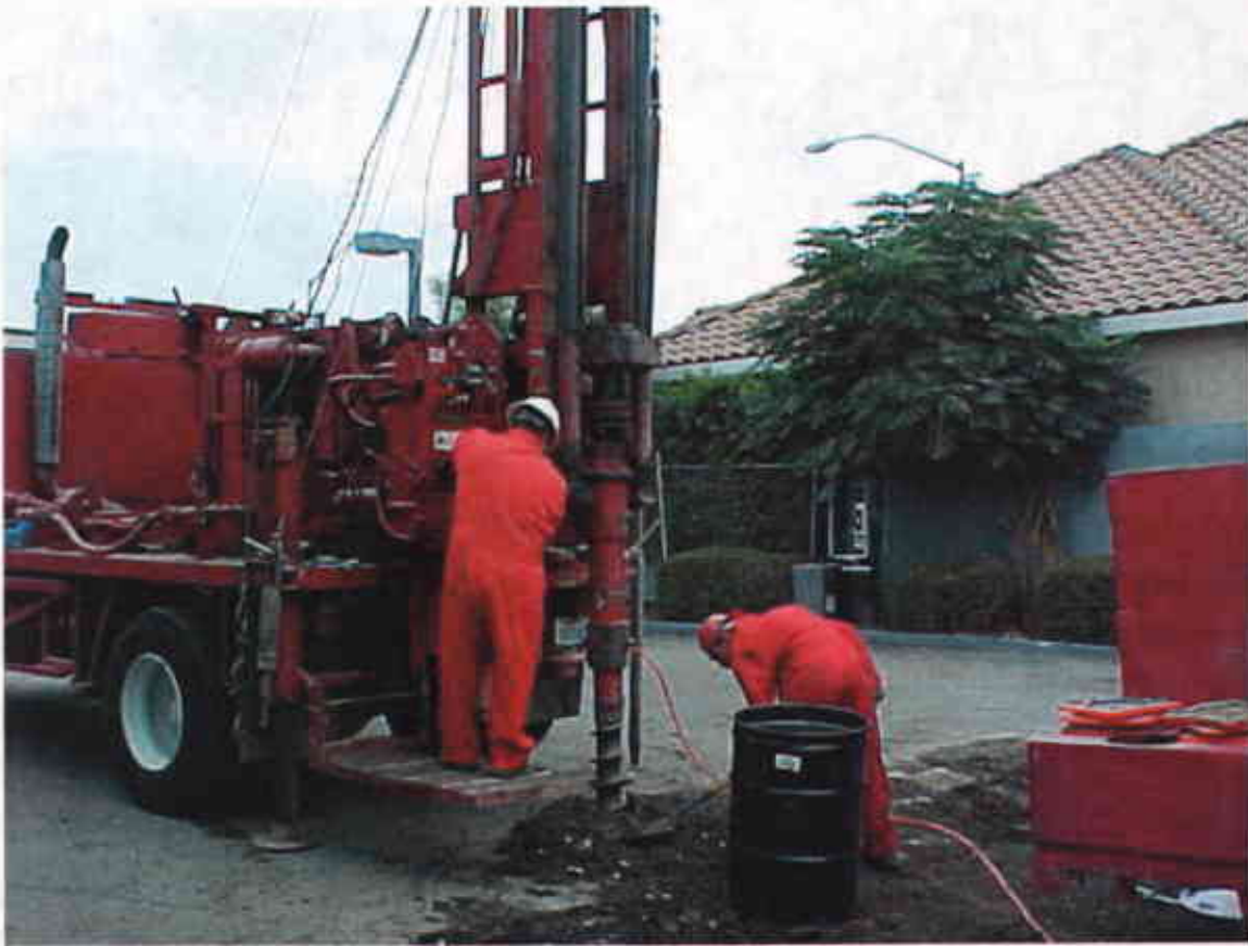
Plate 35: View Northeast showing drill-out of well ESE-3.
