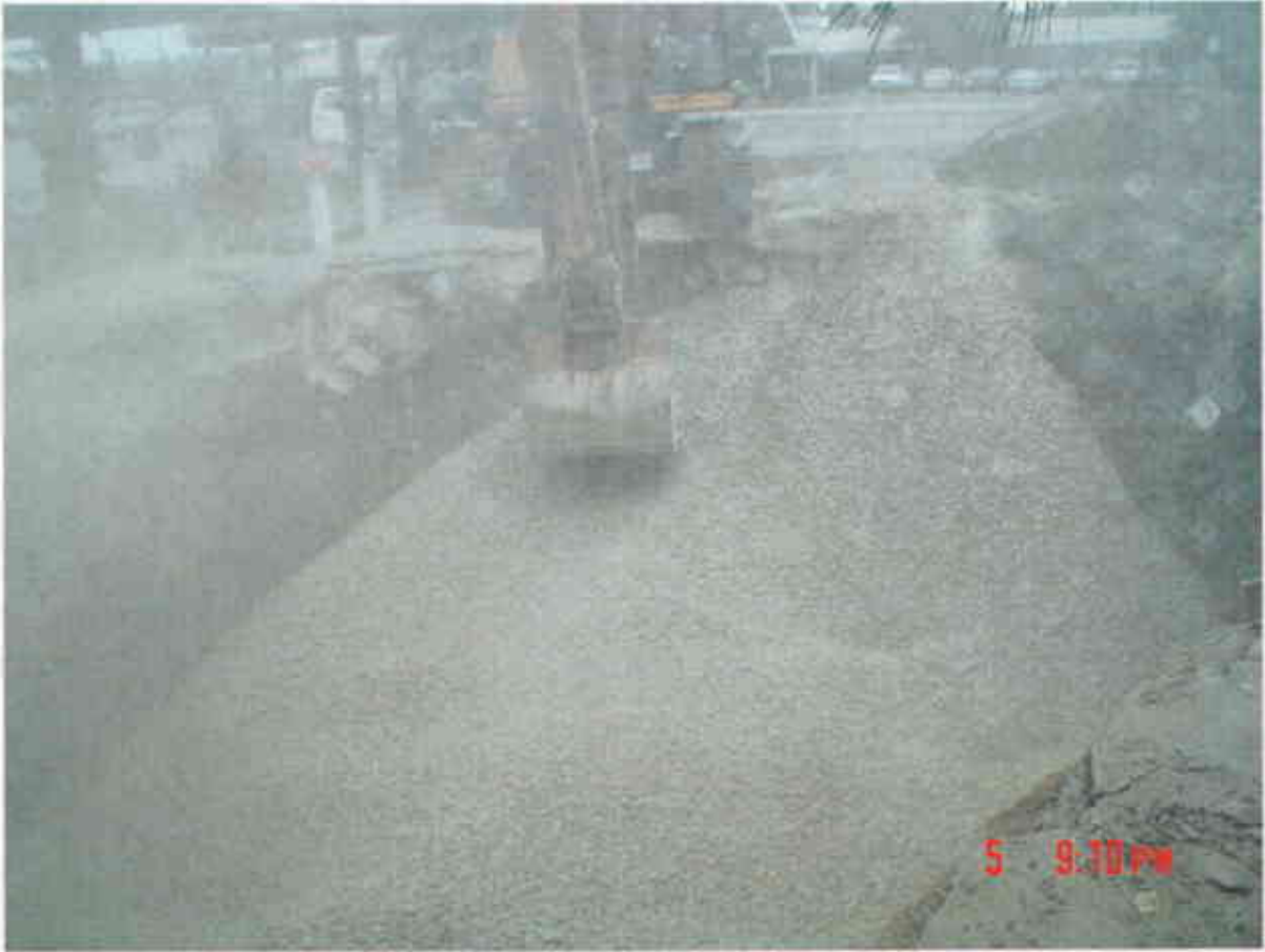
Plate 22: View North showing emplacement of drain rock into former UST pit.
