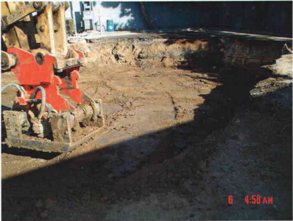
Plate 28: View West showing compaction of imported sandy backfill approaching final grade.
