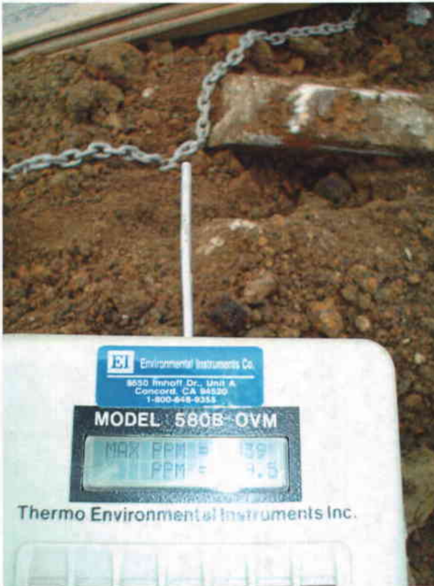
Plate 8: Elevated PID readings as high as 139 ppm during emplacement of shoring.
