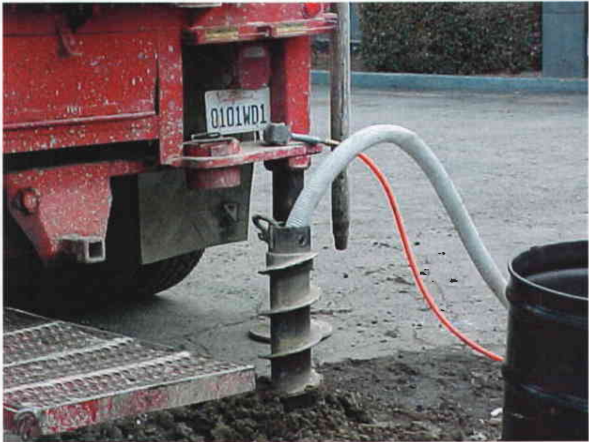
Plate 36: View Northeast showing grouting of well destruction borehole ESE-3.
