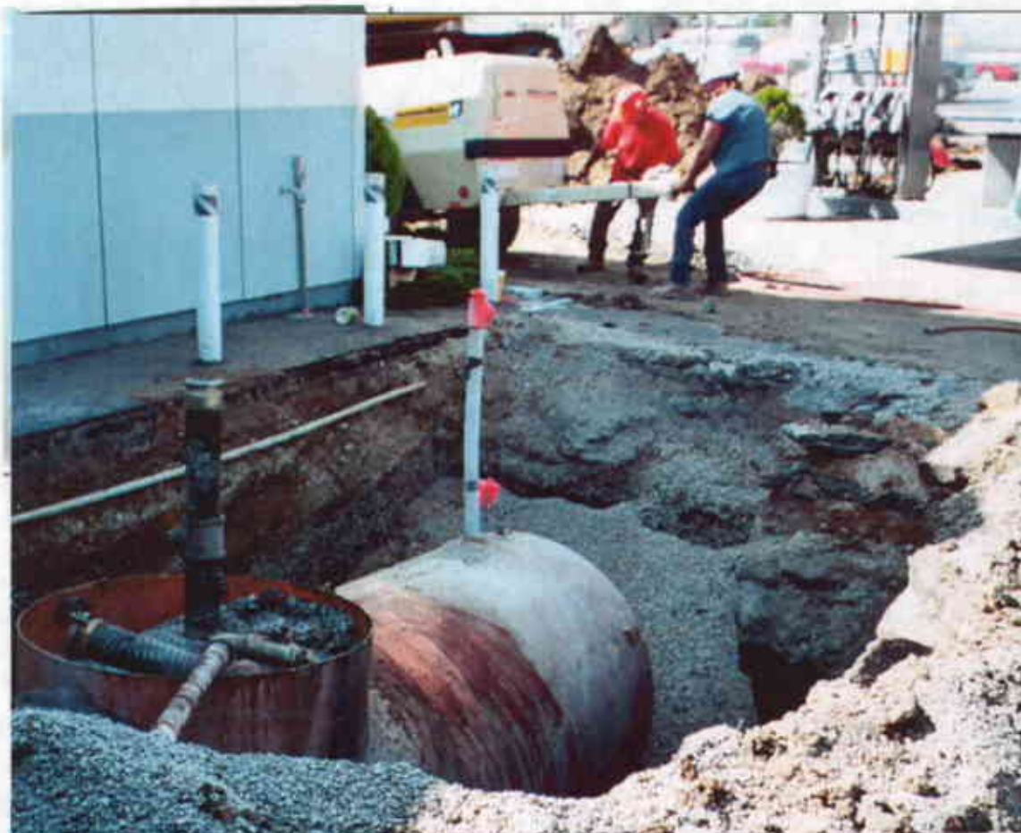
Plate 2: View Northwest showing partially excavated waste oil tank.
