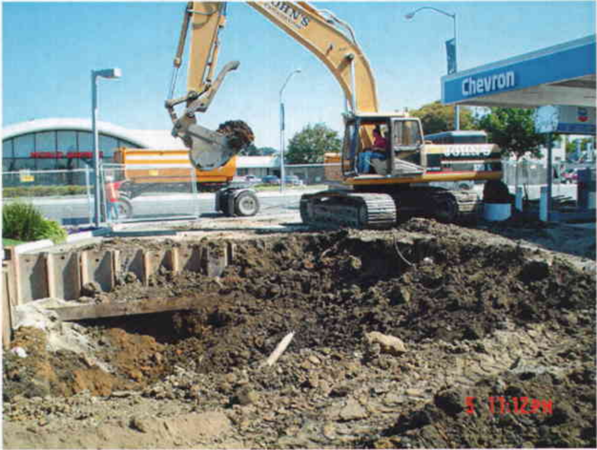
Plate 30: View East showing continued excavation of new UST area.
