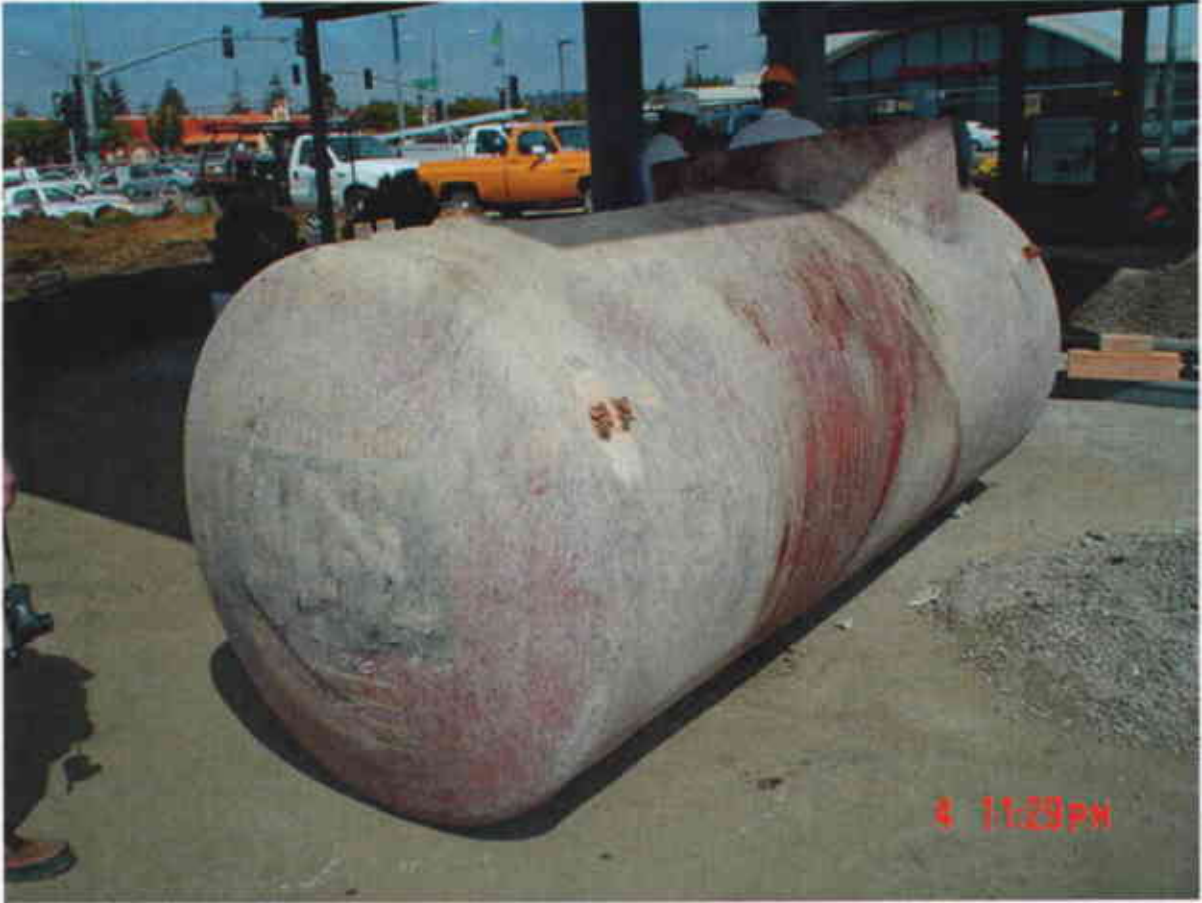
Plate 16: View Northwest showing removed waste oil tank.
