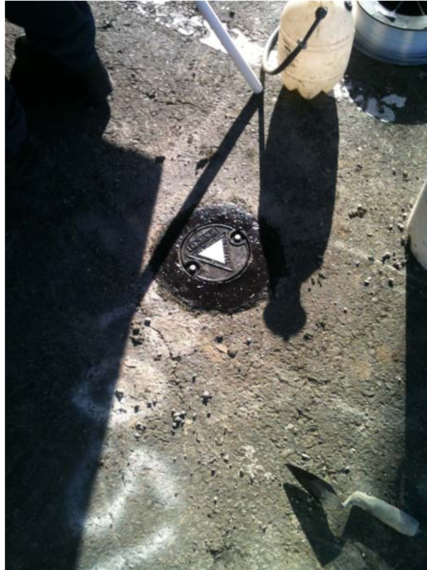
Plate 17. Soil vapor sampling point set with small well box
