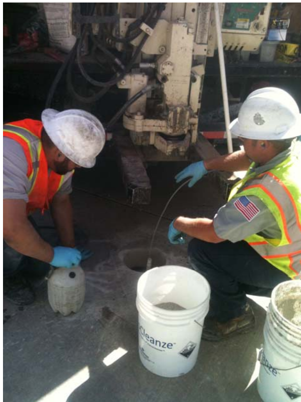
Plate 10. Installation of soil vapor point
