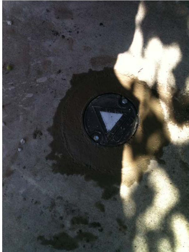
Plate 15. Soil vapor sampling point set with small well box
