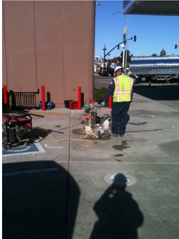
Plate 1. Vironex concrete coring for SV-3
