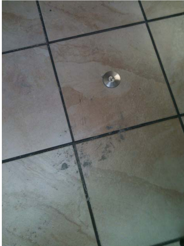
Plate 23. Soil vapor sampling pin installed through tile
