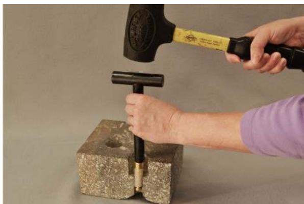
Figure 3. Flush-mount installation.
