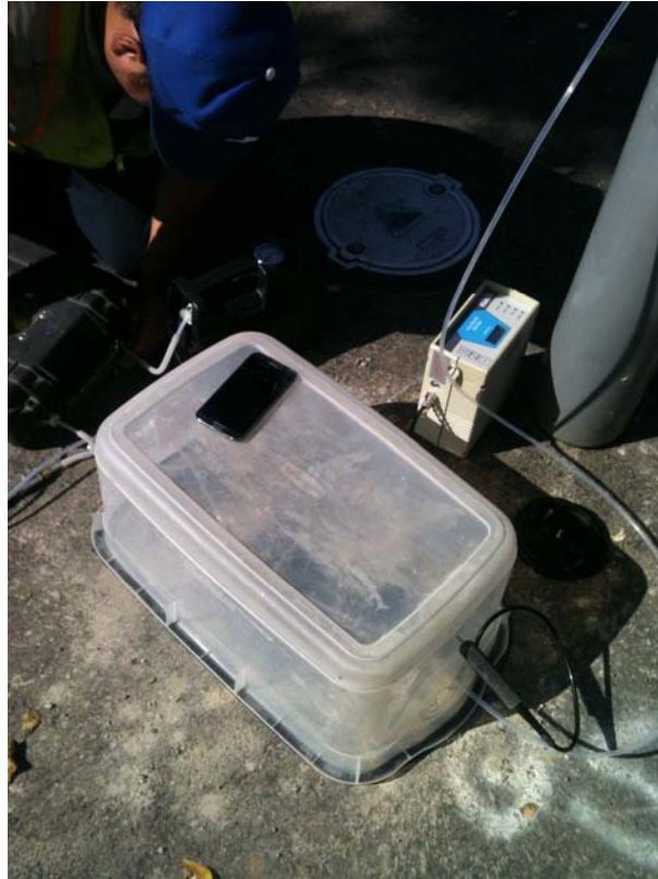
Plate 33. Soil vapor sample set up on SV-1
