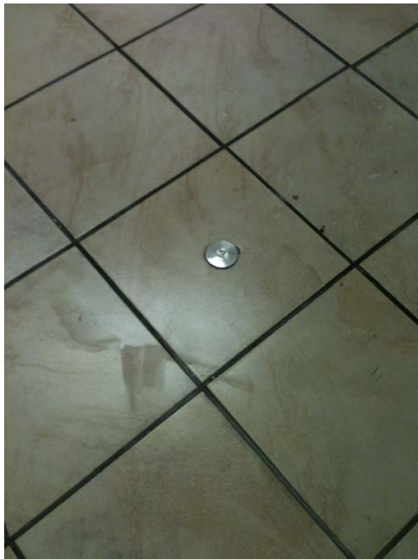
Plate 24. Soil vapor sampling pin installed through tile
