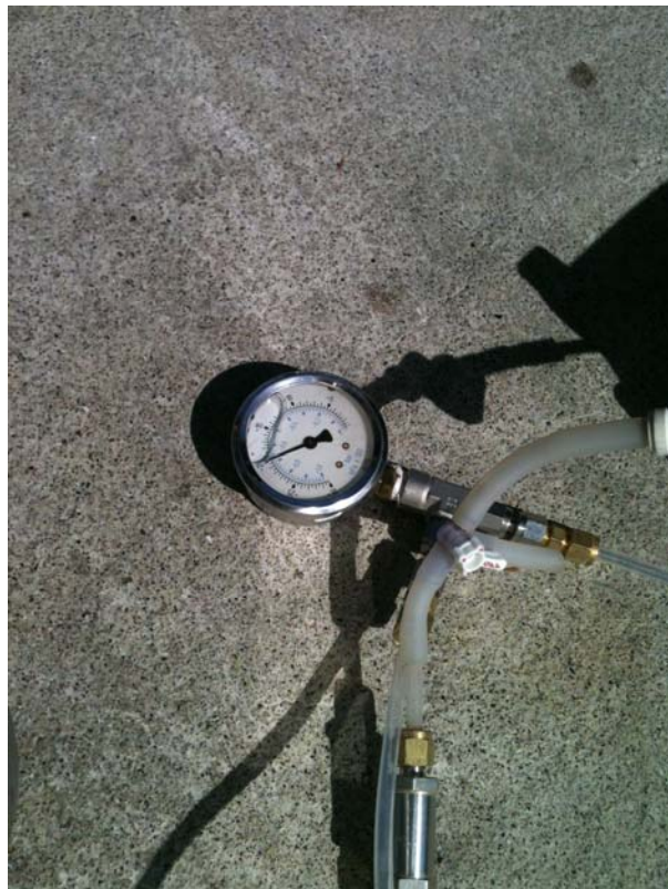
Plate 32. Shut-in test showing continuous vacuum held for two minutes
