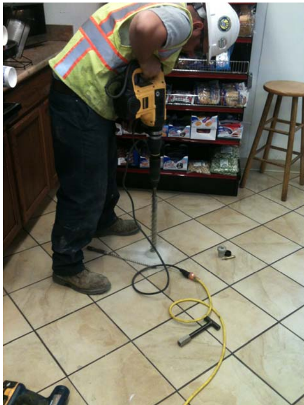
Plate 22. Drilling through tile to install soil vapor sampling pin
