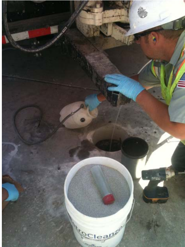
Plate 11. Installation of soil vapor point
