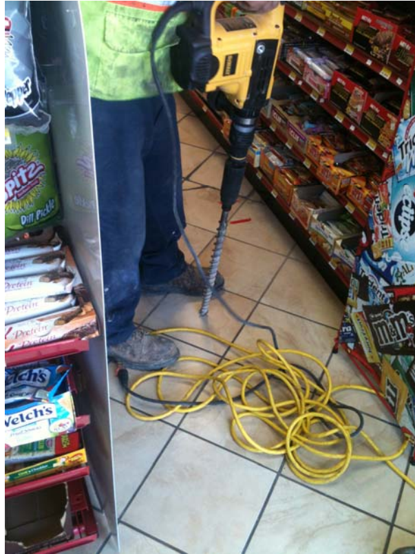
Plate 21. Drilling through tile to install soil vapor sampling pin
