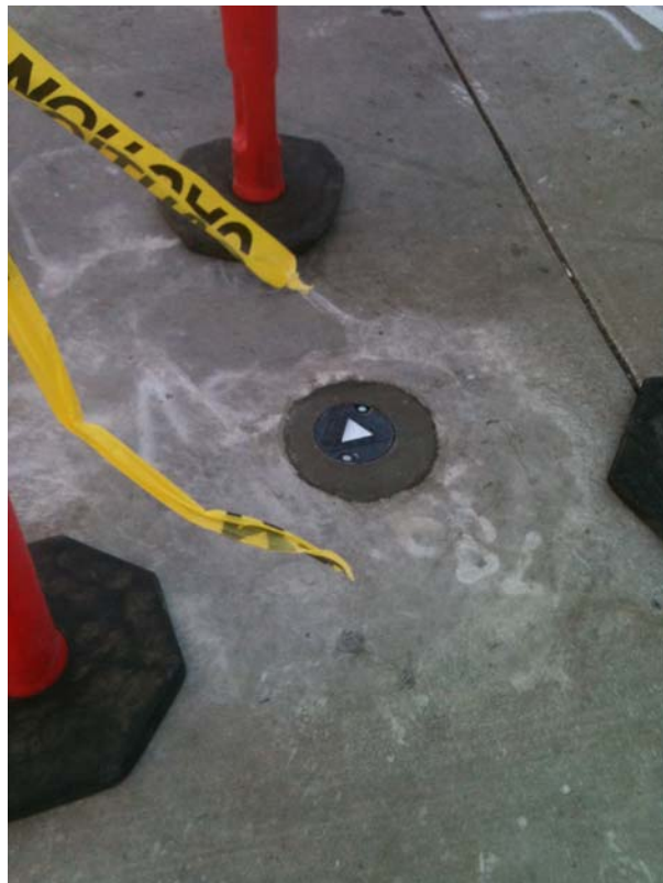
Plate 18. Soil vapor sampling point set with small well box
