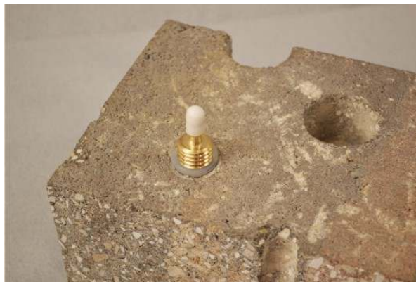
Figure 4. Installed Vapor Pin™.
