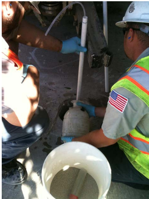
Plate 8. Adding water to hydrate bentonite for vapor point seal
