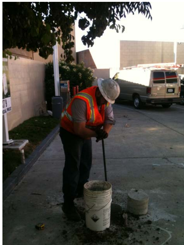
Plate 2. Using a hand auger to clear location for SV-4
