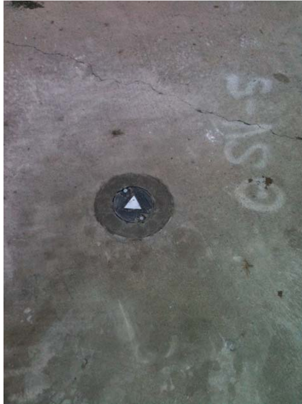
Plate 19. Soil vapor sampling point set with small well box
