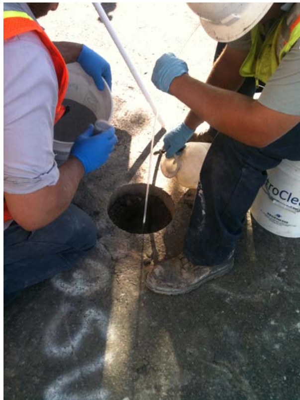
Plate 14. Adding water to hydrate bentonite
