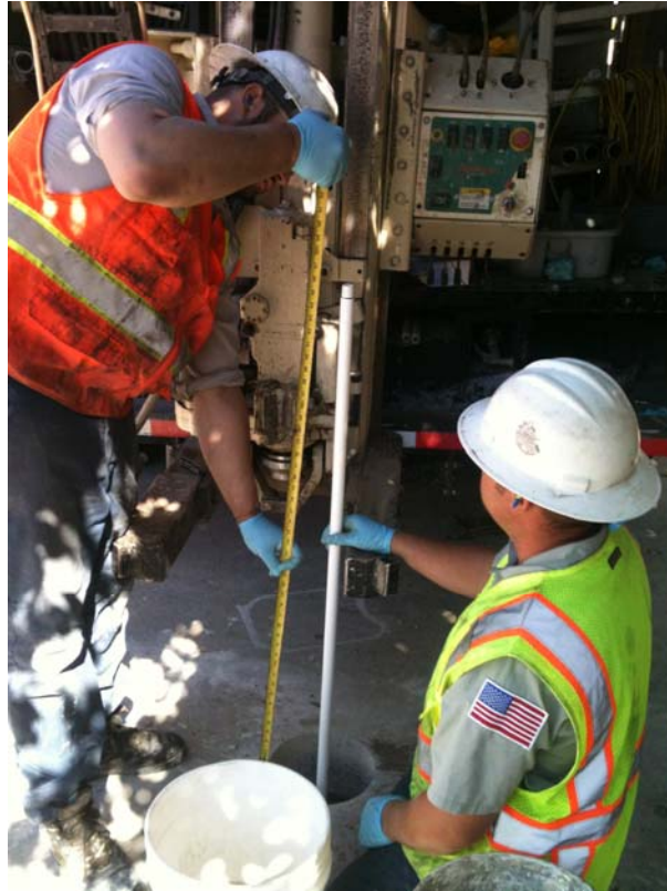
Plate 7. Constructing soil vapor point
