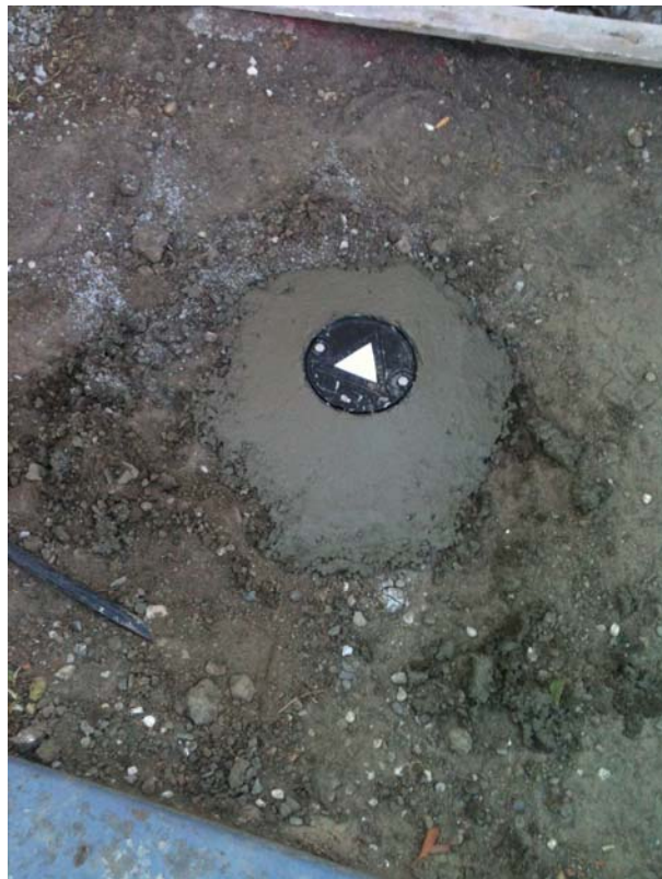
Plate 16. Soil vapor sampling point set with small well box
