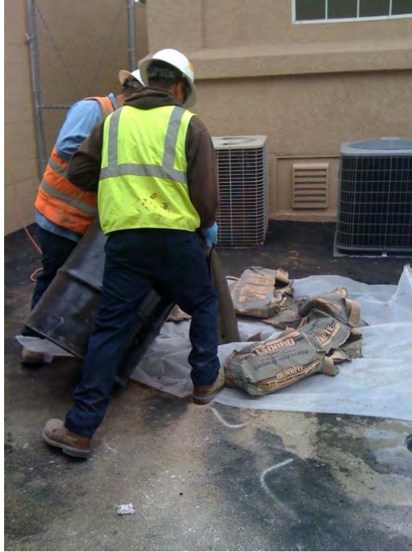
Plate 13. View of RSI grouting SOMA-9
