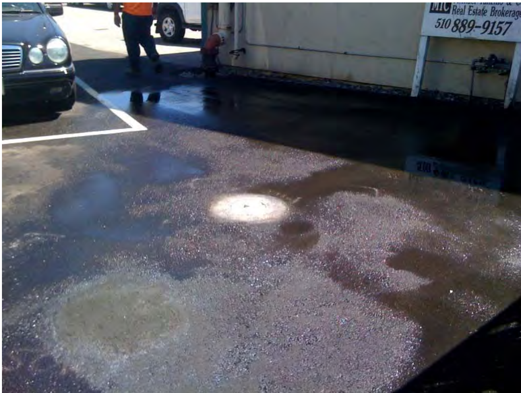
Plate 14. View of MW-7R and SOMA-9 after finishing to grade
