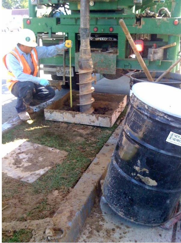
Plate 3. View of RSI setting well in MW-6R
