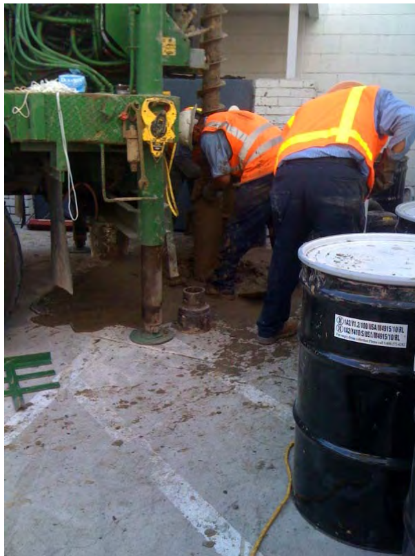
Plate 8. View of ESE-1R being over drilled with 10-inch auger
