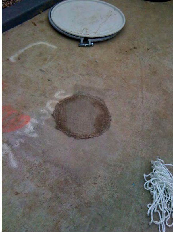
Plate 9. View of SOMA-6 after grouting and completion to grade
