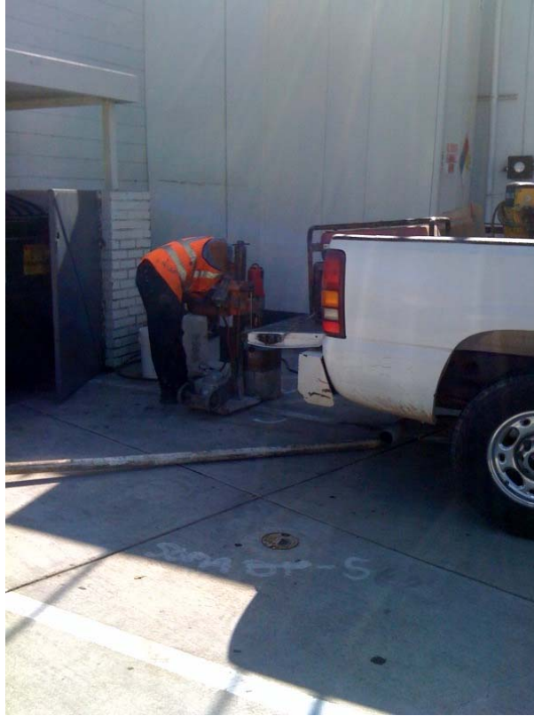
Plate 5. View of ESE-1 being concrete cored
