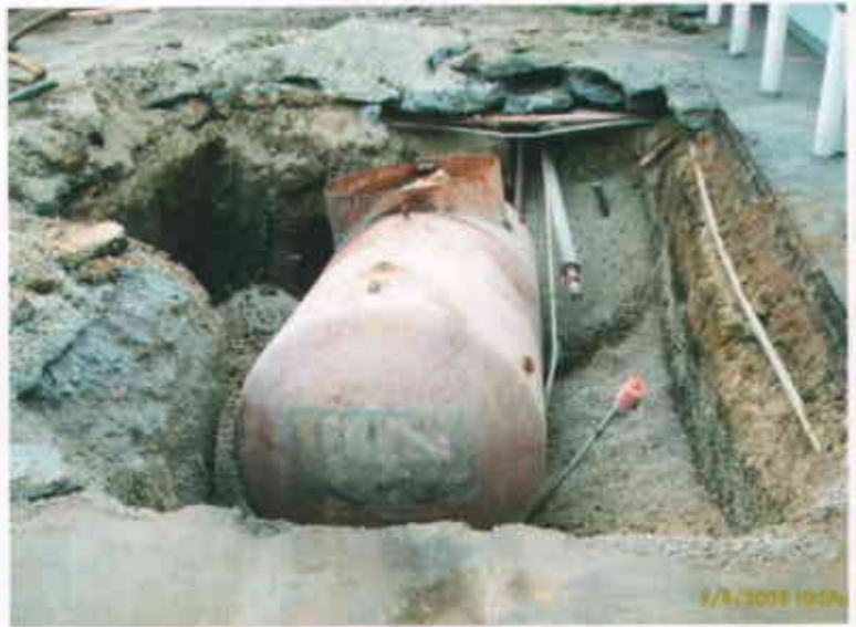
Castro Valley Chevron 3519 Castro Valley Boulevard Castro Valley CA 94546 September 4, 2003 Used oil tank 2K DW FRP
