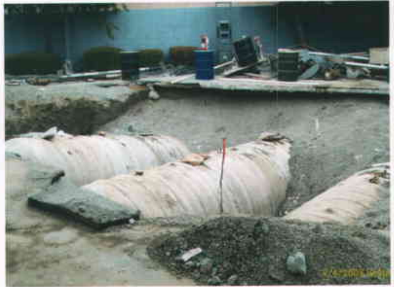
Castro Valley Chevron 3519 Castro Valley Boulevard Castro Valley CA 94546 September 4, 2003 SW FRP Fuel tanks staged for removal
