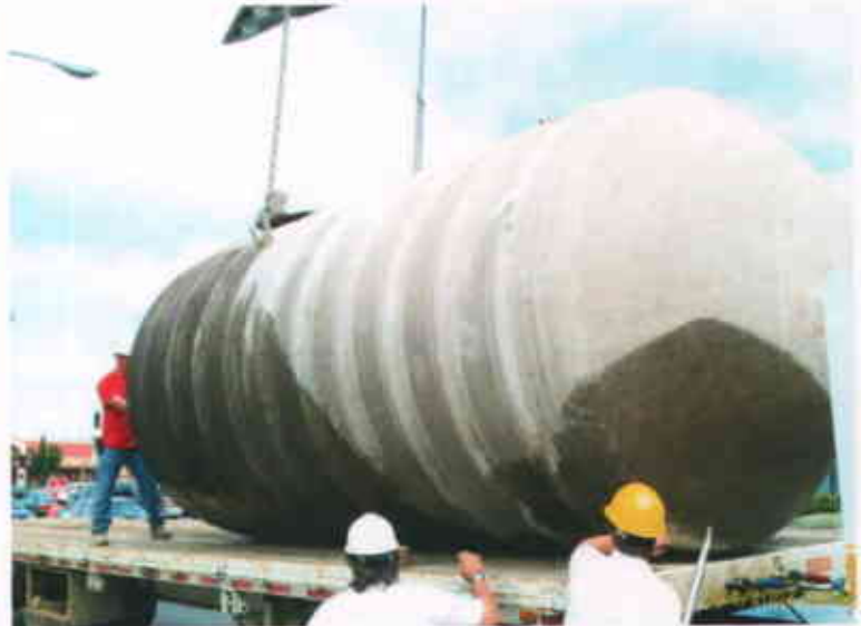
Castro Valley Chevron 3519 Castro Valley Boulevard Castro Valley CA 94546 September 4, 2003 SW FRP Fuel tank, no apparent faults
