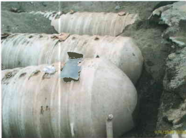
Castro Valley Chevron 3519 Castro Valley Boulevard Castro Valley CA 94546 September 4, 2003 SW FRP Fuel tanks staged for removal
