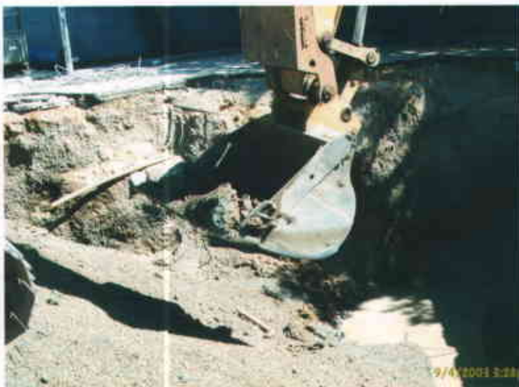
Castro Valley Chevron 3519 Castro Valley Boulevard Castro Valley CA 94546 September 4, 2003 Soil water interface sampling in former tank pit, stained soil (blue green)
