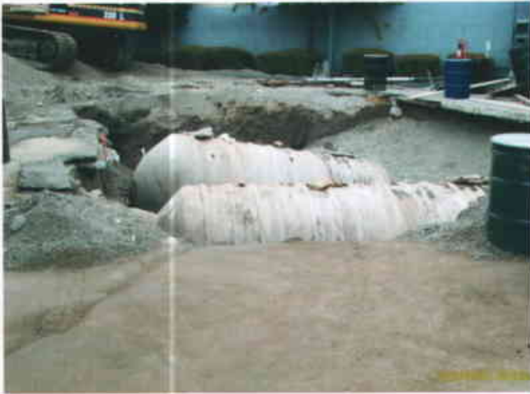
Castro Valley Chevron 3519 Castro Valley Boulevard Castro Valley CA 94546 September 4, 2003 SW FRP Fuel tanks staged for removal
