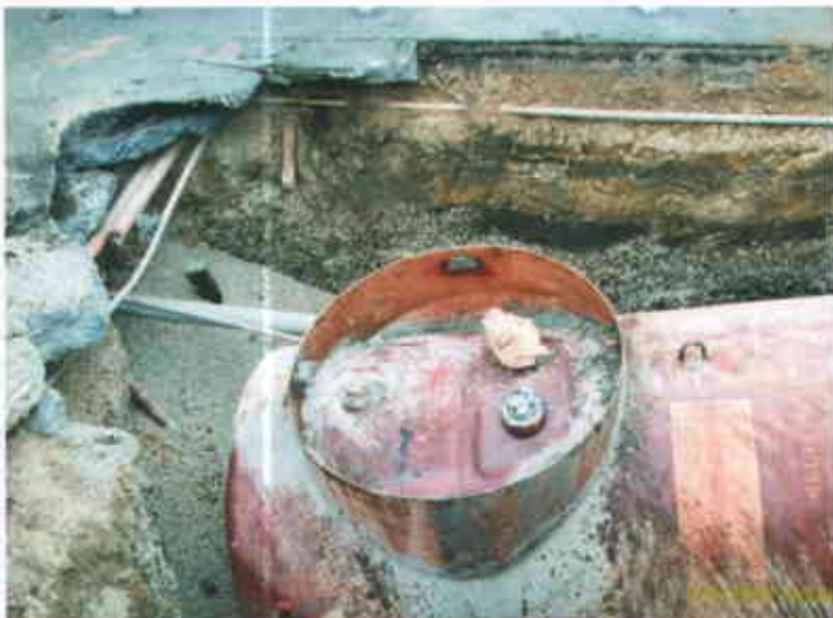
Castro Valley Chevron 3519 Castro Valley Boulevard Castro Valley CA 94546 September 4, 2003 Used oil tank 2K DW FRP No apparent leaks in tank
