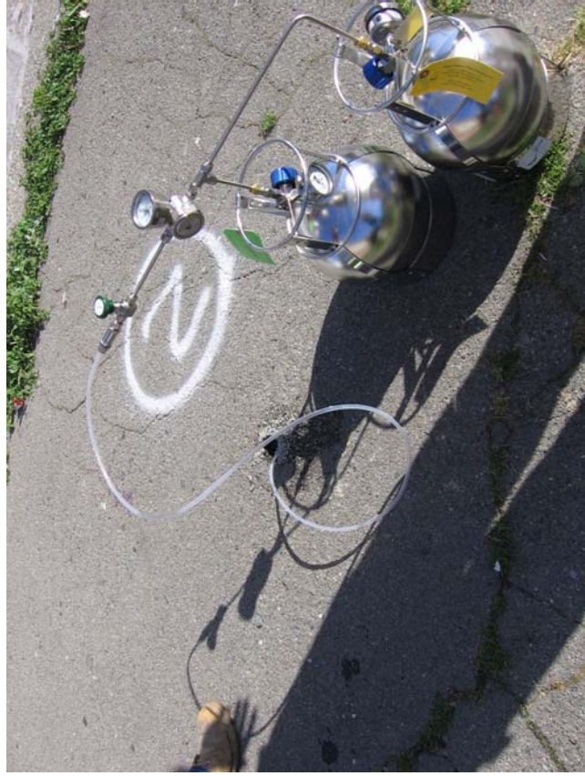
Photograph 3: Soil vapor extraction in progress.
