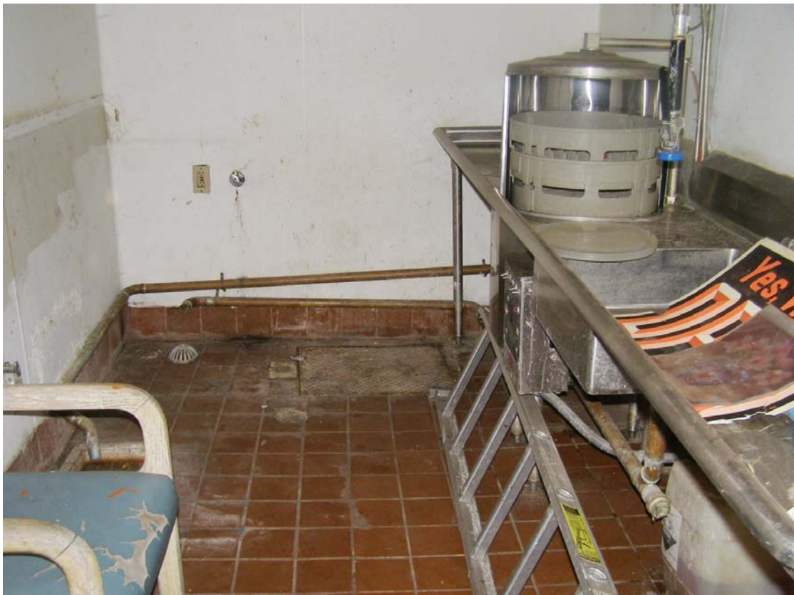
Photograph 4 - View of the dishwashing area with detergent container
