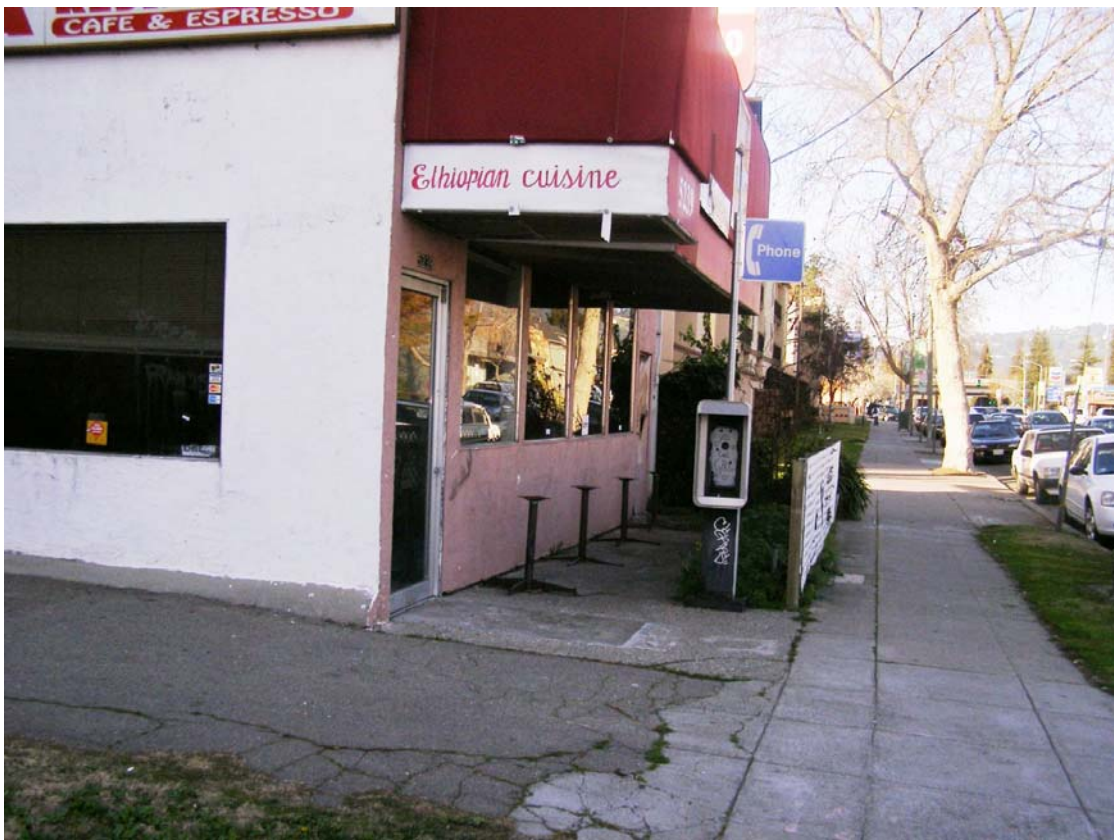
Photograph 1 - View front of the building from the south
