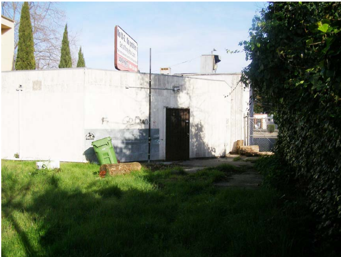
Photograph 3 - View to the east of the rear of the building and yard
