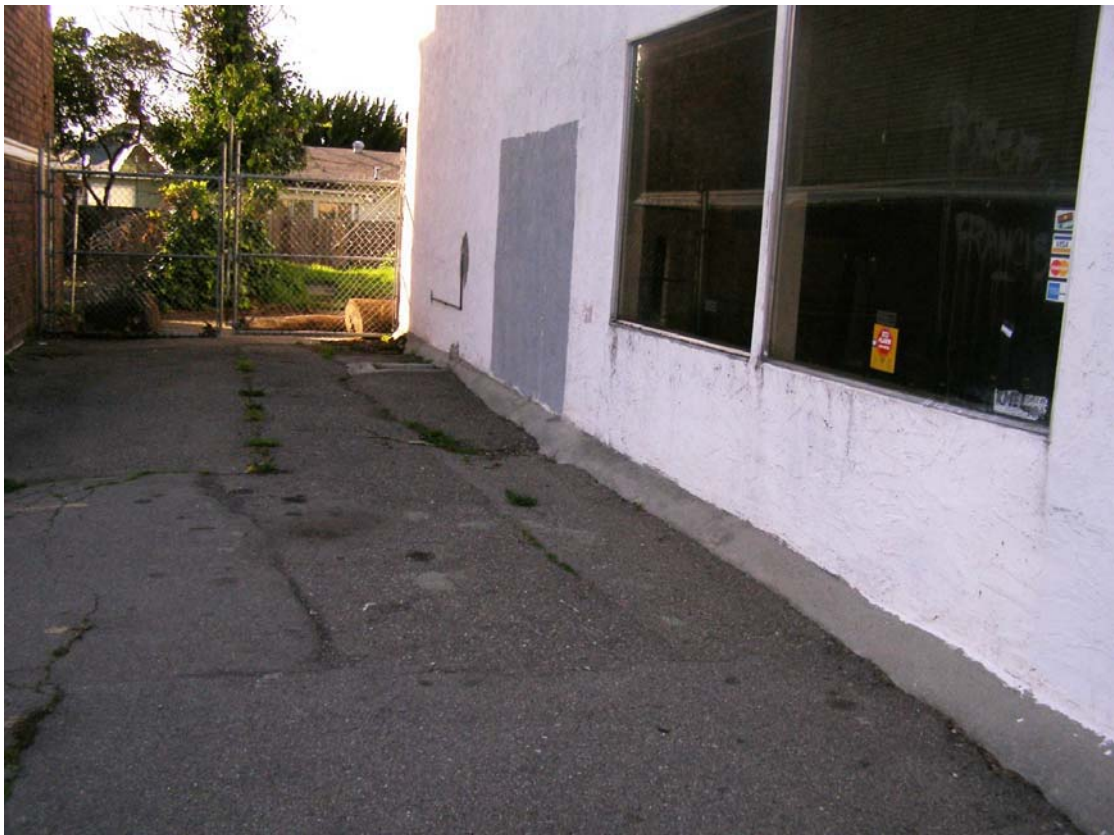
Photograph 2 - View of the south side of the building and driveway
