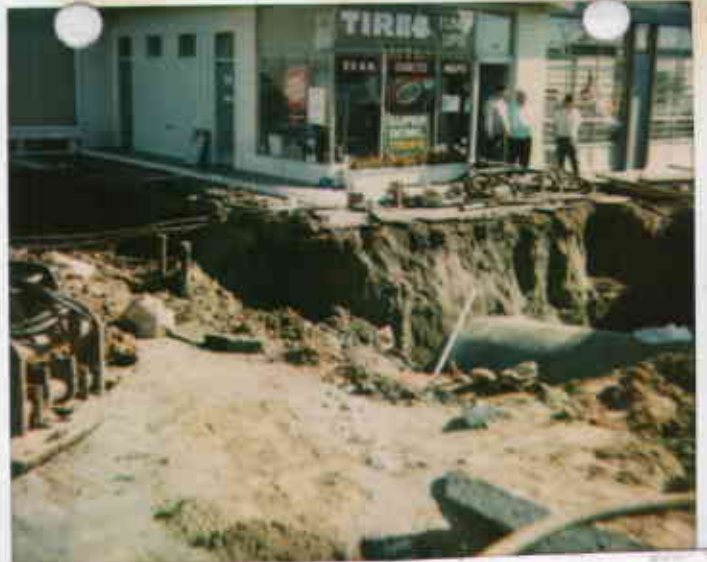
10/16/95 08416201511-2 726 2028 0192 view of 8k + 5k tanks Harrison
