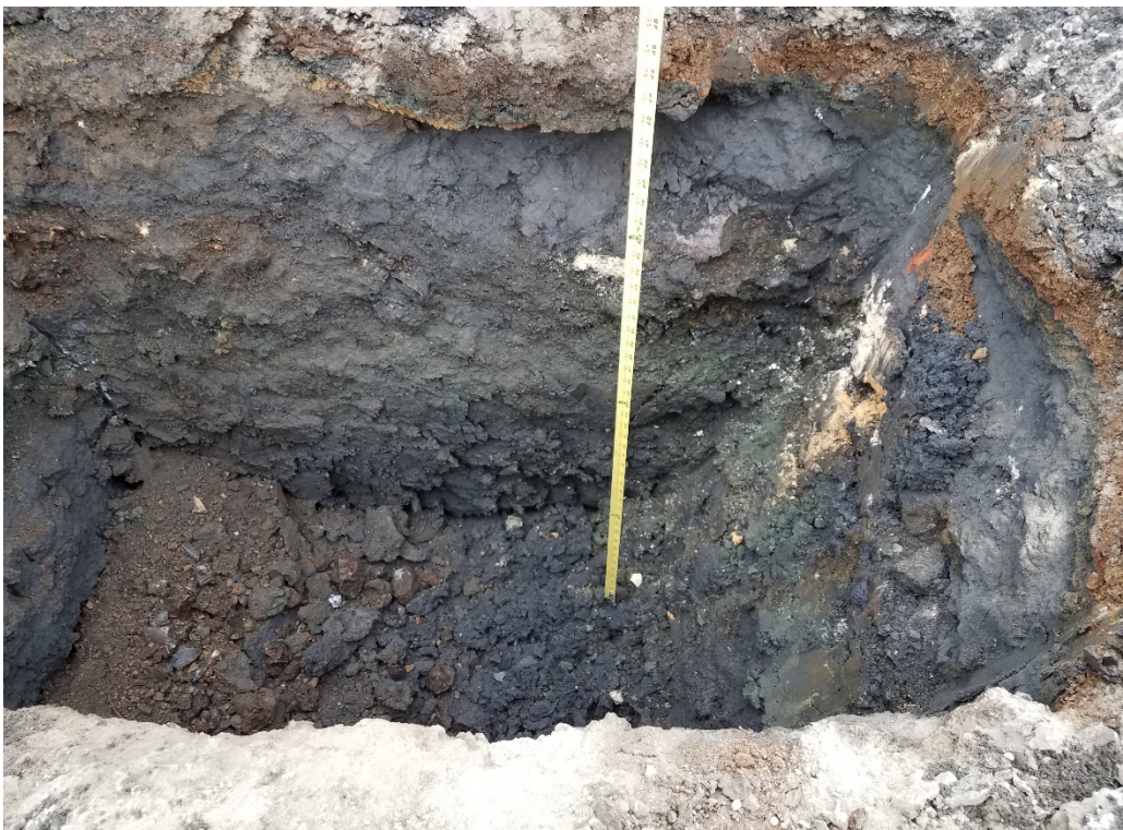
Photograph 2: Taken facing North East. Eastern pothole. No UST was found in this pothole.
