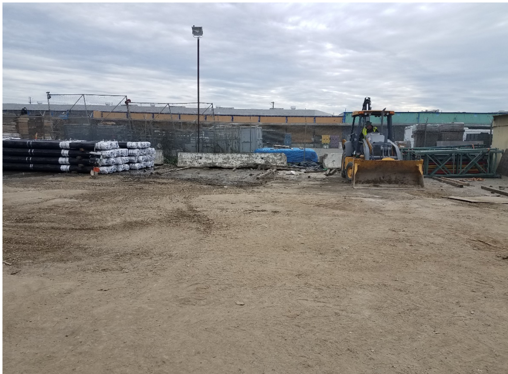
Photograph 4: Taken facing South East. Pothole area post backfill and clean up.
