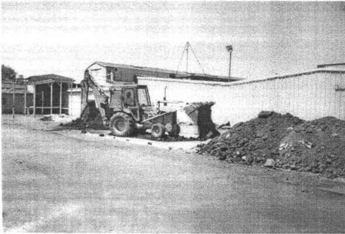
Picture 13 Placing excavated soil onto plastic lining. August 3, 1992
