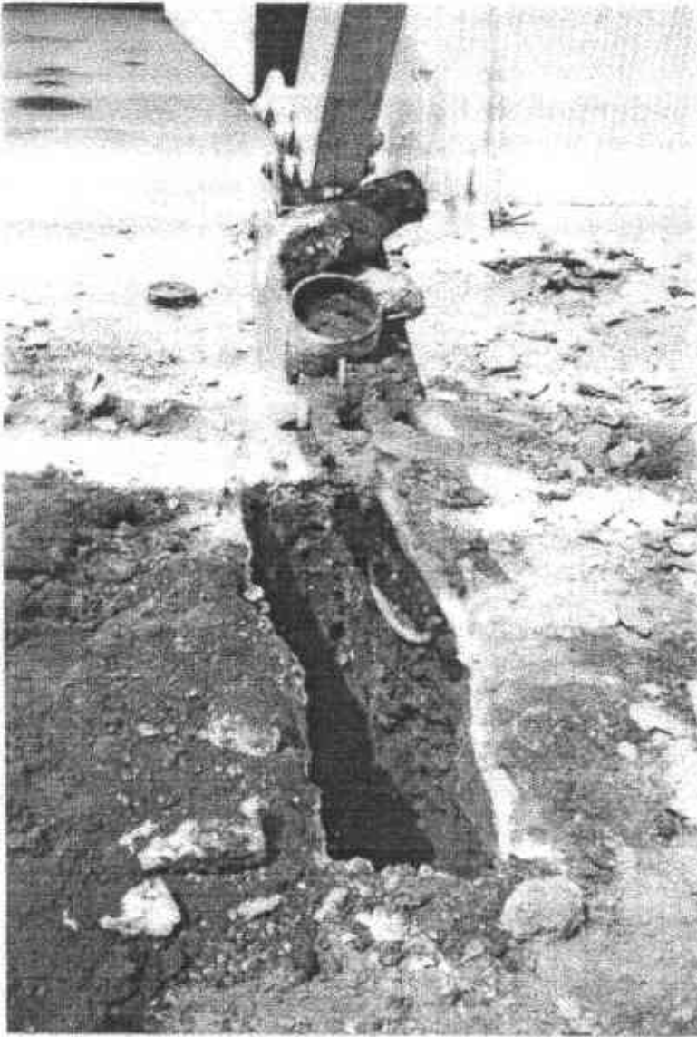
Picture 3: Backhoe removing debris found in excavation. June 29, 1992
