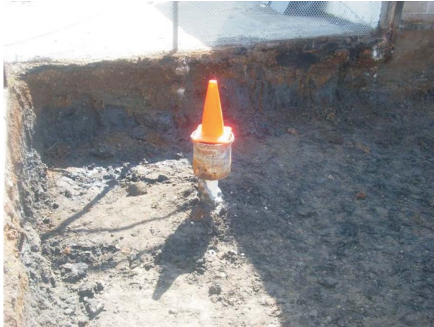
Excavation Around Well MW-2
