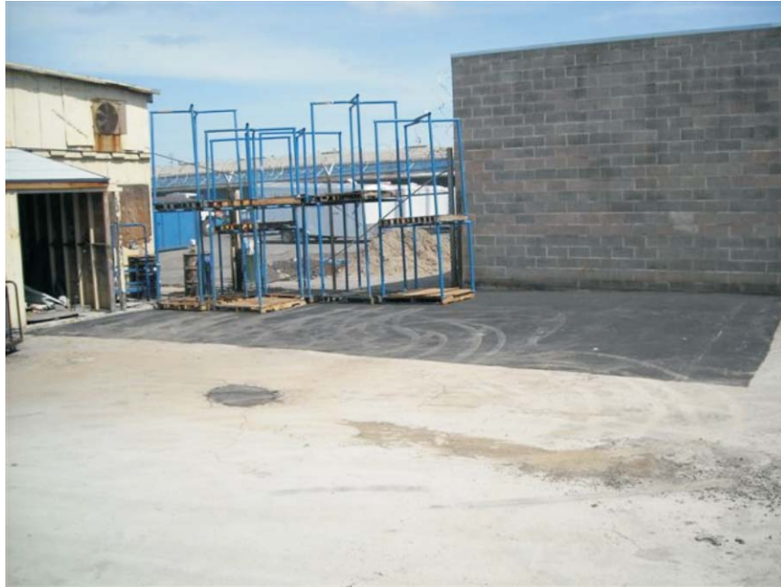
Area of Excavation Post-Paving
