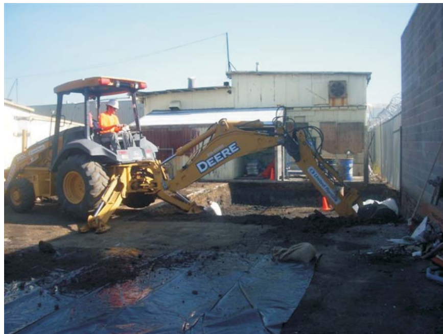
Expanding Excavation Looking East
