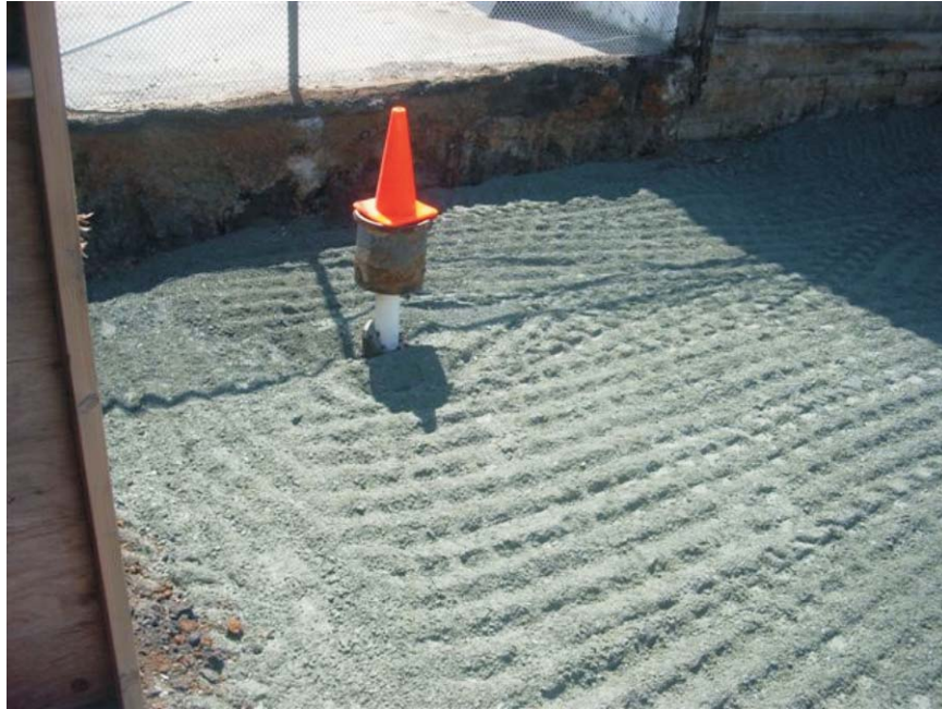
Backfilling Excavation Around Well MW-2
