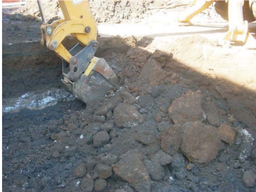
Excavation of Soil Along the Northern Wall
