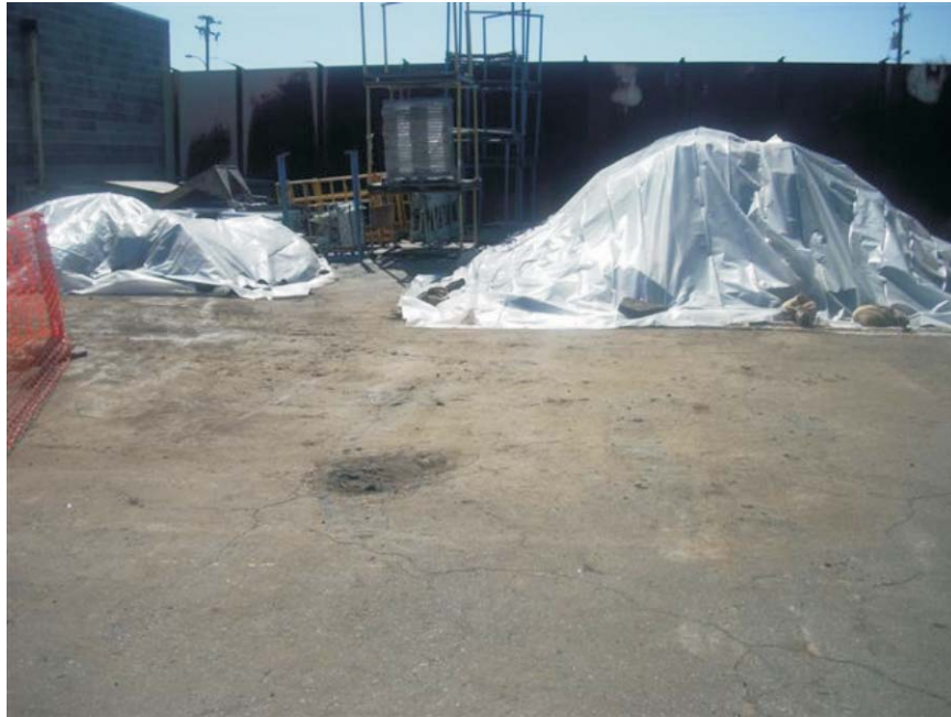
Covered Stockpiles of Excavated Soil
