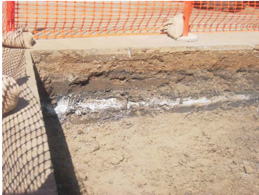
Northwestern Wall of Excavation
