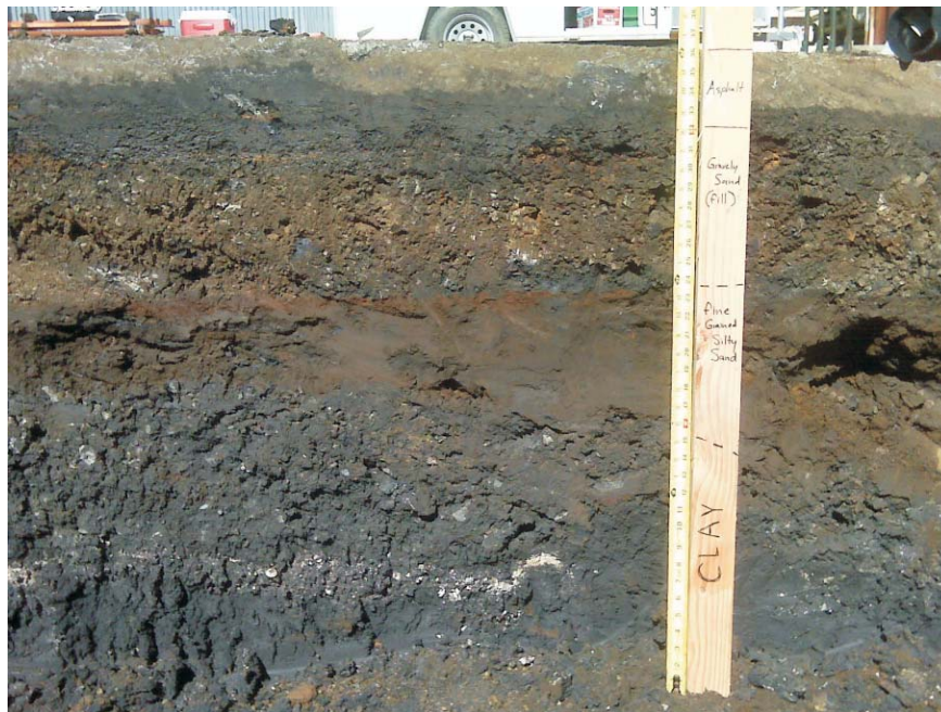
North Wall of Excavation Prior to Excavation Expansion
