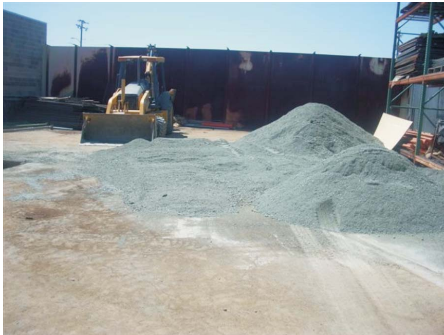
Imported Backfill
