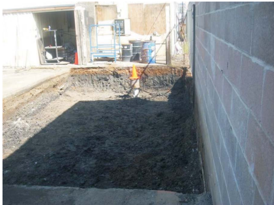
Initial Excavation Looking East
