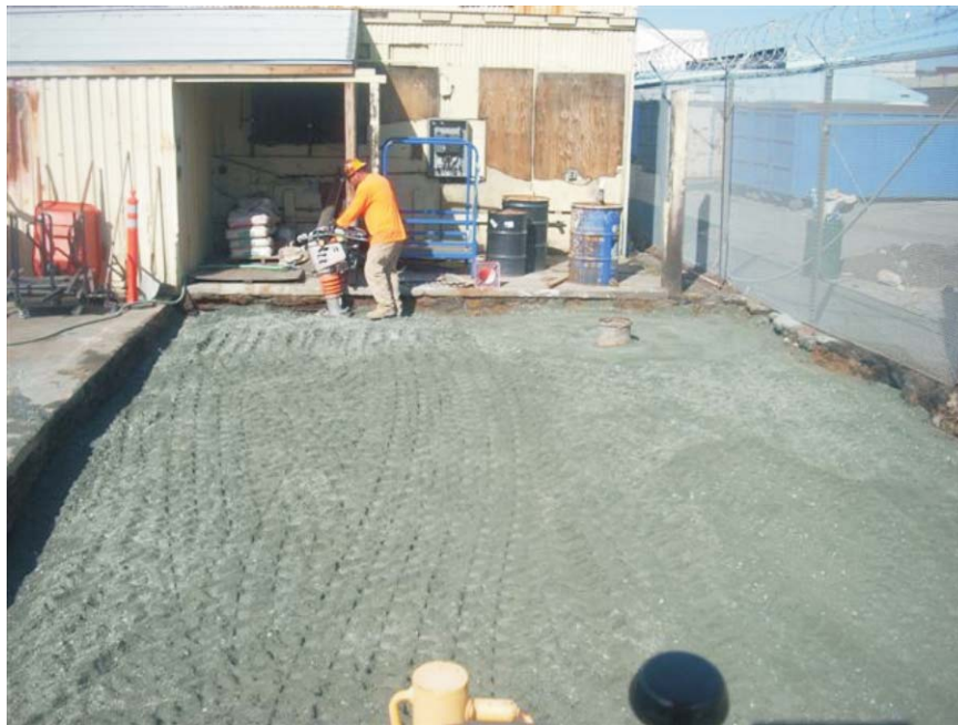
Compacting Excavation
