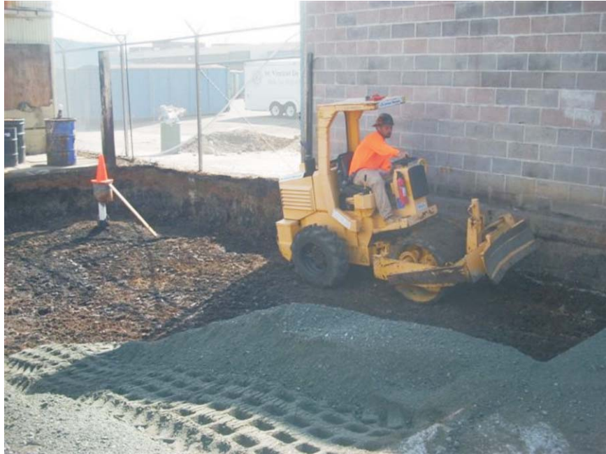
Compacting Excavation-1
