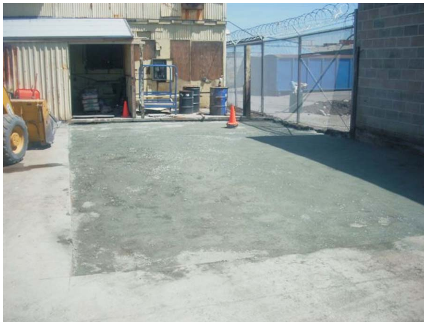
Backfilled Excavation
