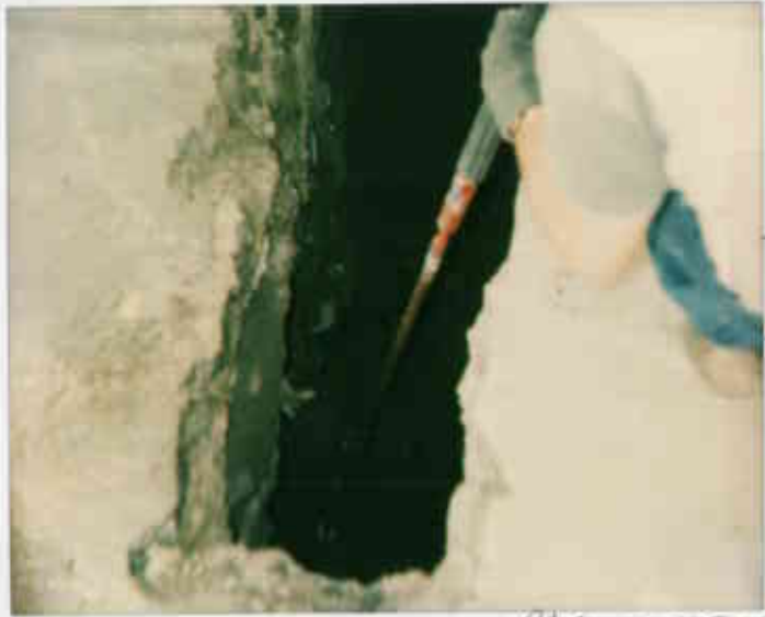
6/30/92 Drive spile @ 6' w pit (tranche) Photo 9201 SLST where tank was removed (B1) (P1) = spile from soil pile
