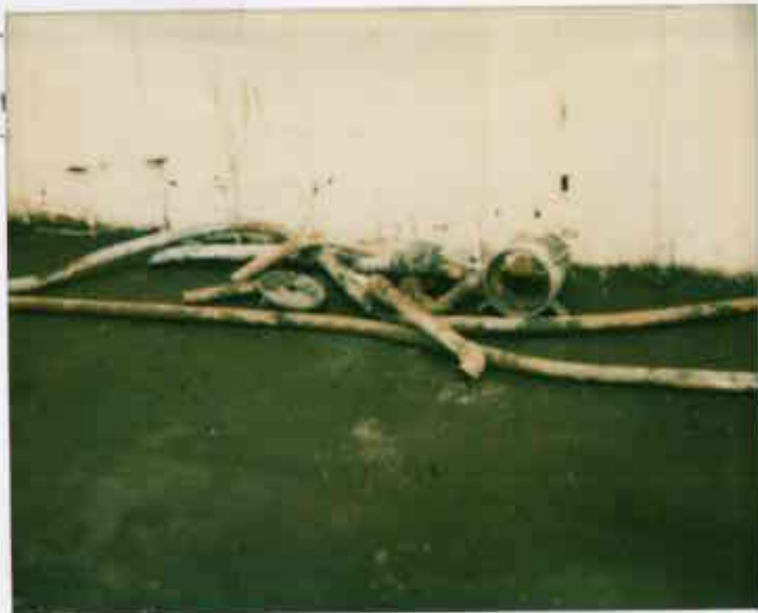
6/30/92 - From trench (pit) 9201 San Pedro St (pipes + trench)
