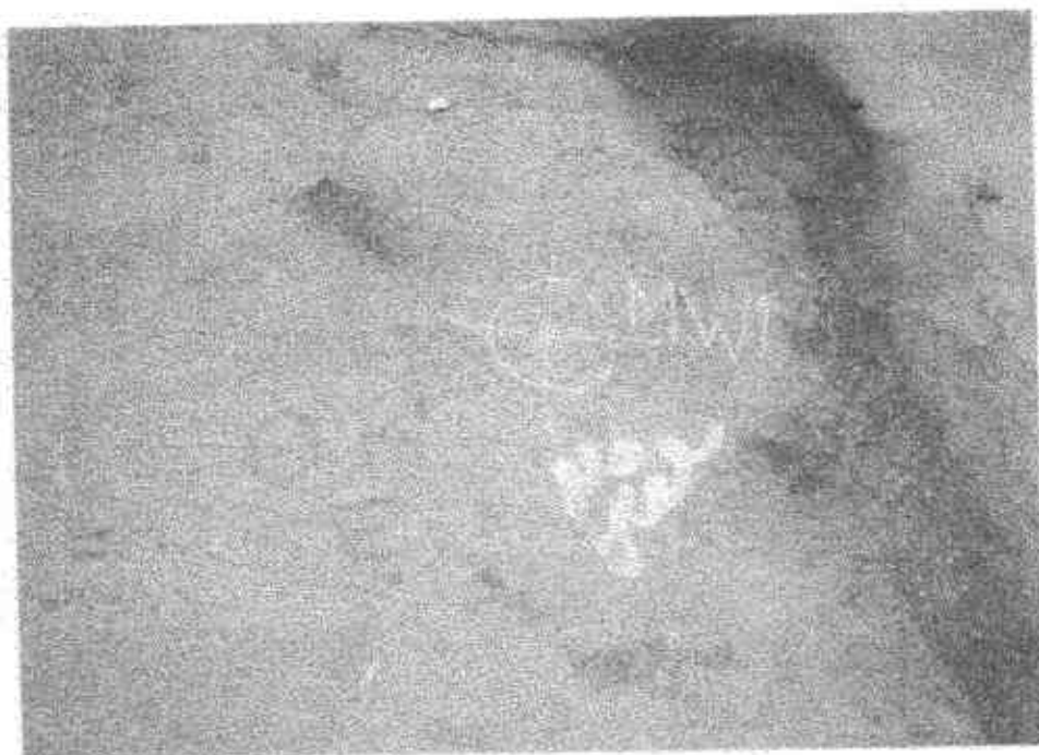
Picture 3: November 4, 1992 Approval to drill markings from utility inspectors at the proposed location of monitoring well 9MW1.
