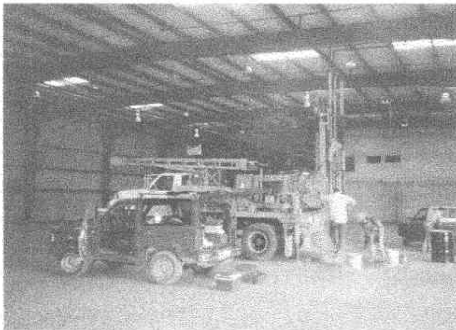
Picture 11: November 9, 1992 Drilling borehole for monitoring well 9MW4.
