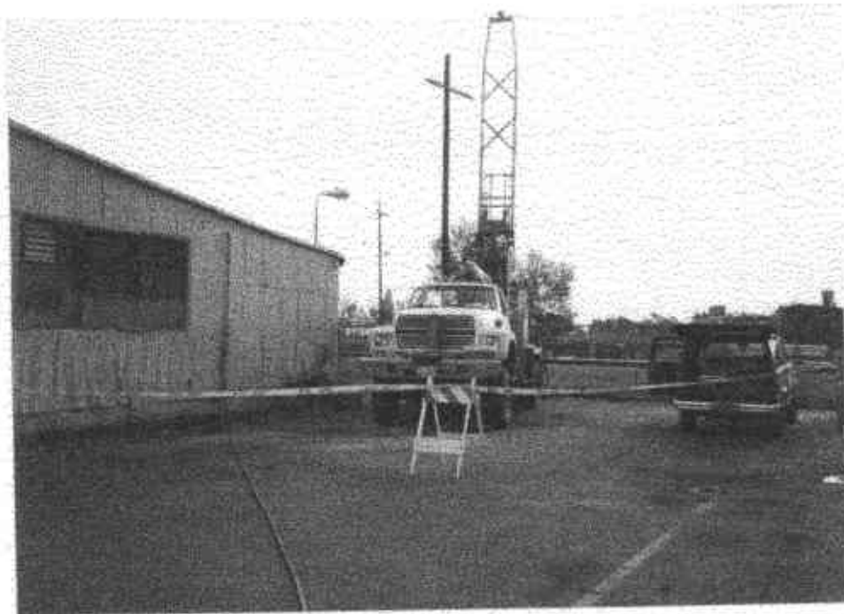
Picture 2: November 4, 1992 Advance Drilling Company CME-75 rig drilling monitoring well 9MW1.
