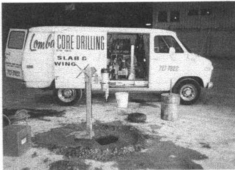
Picture 10: November 9, 1992 Coring through the floor of the warehouse prior to drilling the borehole for monitoring well 9MW4.
