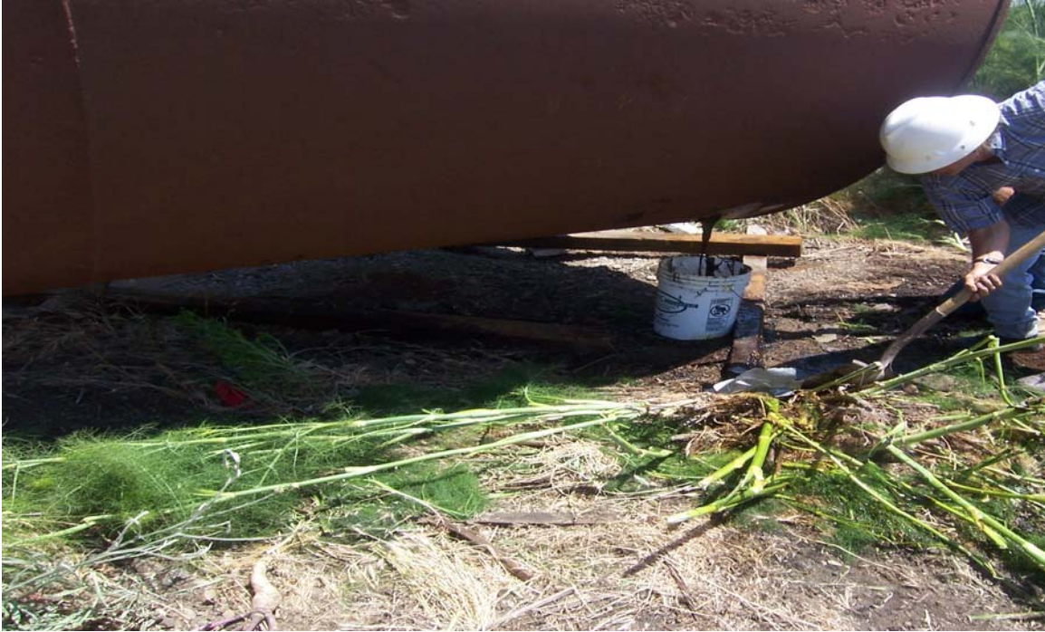
9. Waste oil sludge leaking from a hole in AST T-2.
