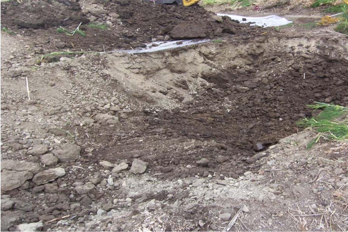
19. Excavation in the former location of AST T-3.
