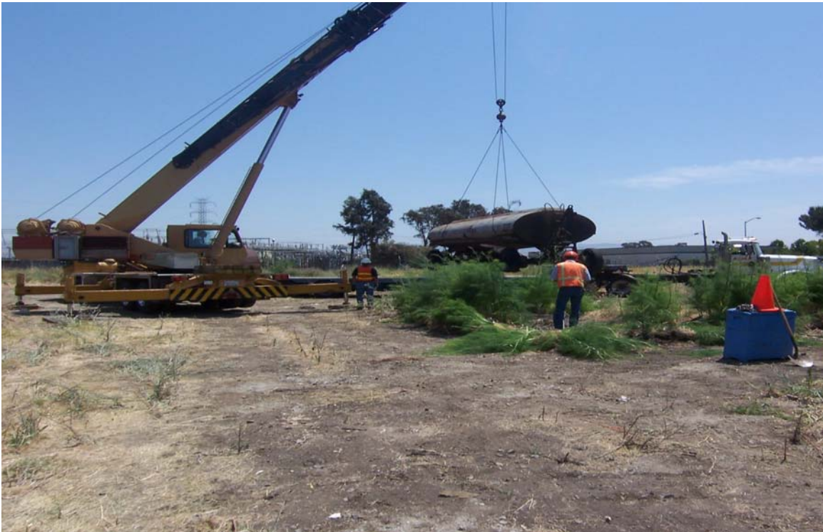
14. AST T-3 being moved onto the ECI truck.
