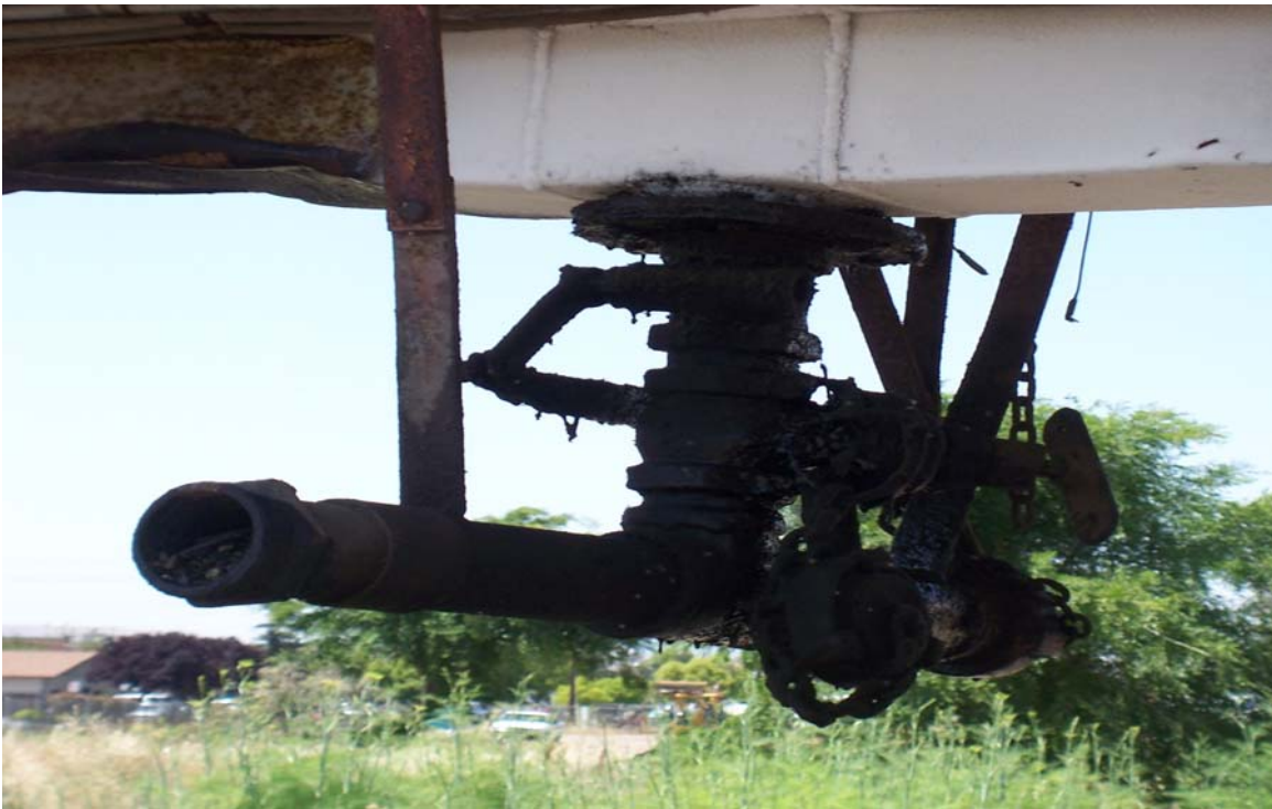
16. Detail view of the piping under AST T-3.
