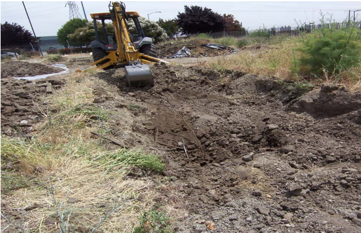
20. Excavation of former AST location T-4.
