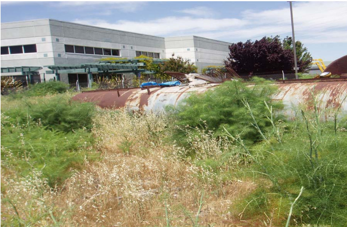
2. View of AST T-1 from the southwest.
