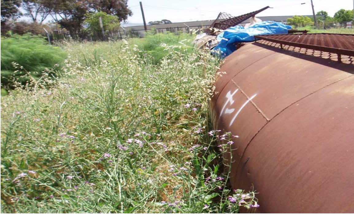
3. View along the eastern side of AST T-1. There is a large hole in the tank near the center, under the tarp.
